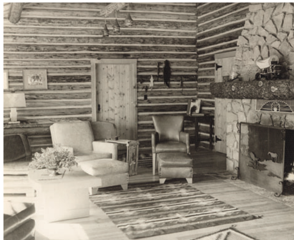
Main Lodge at the Firehole Ranch
