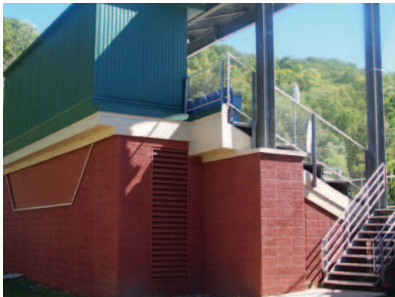
After power cleaning and new paint
