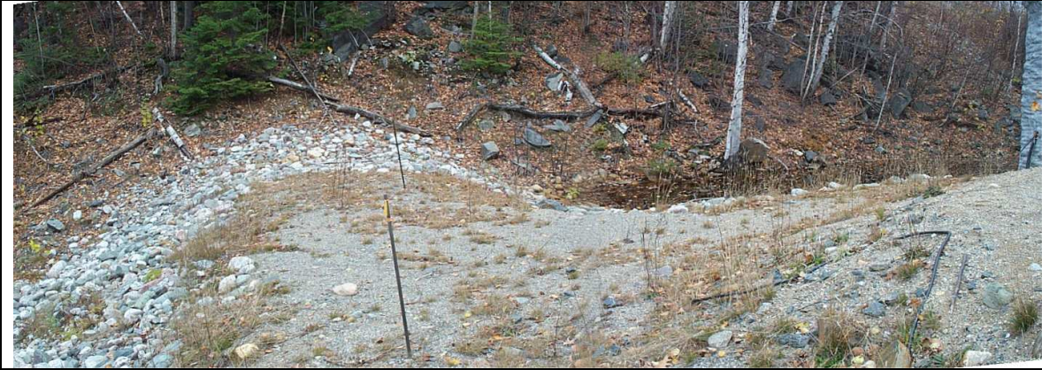
Photo 1: East Seepage Collection Pond Dam – Nordic TMA
