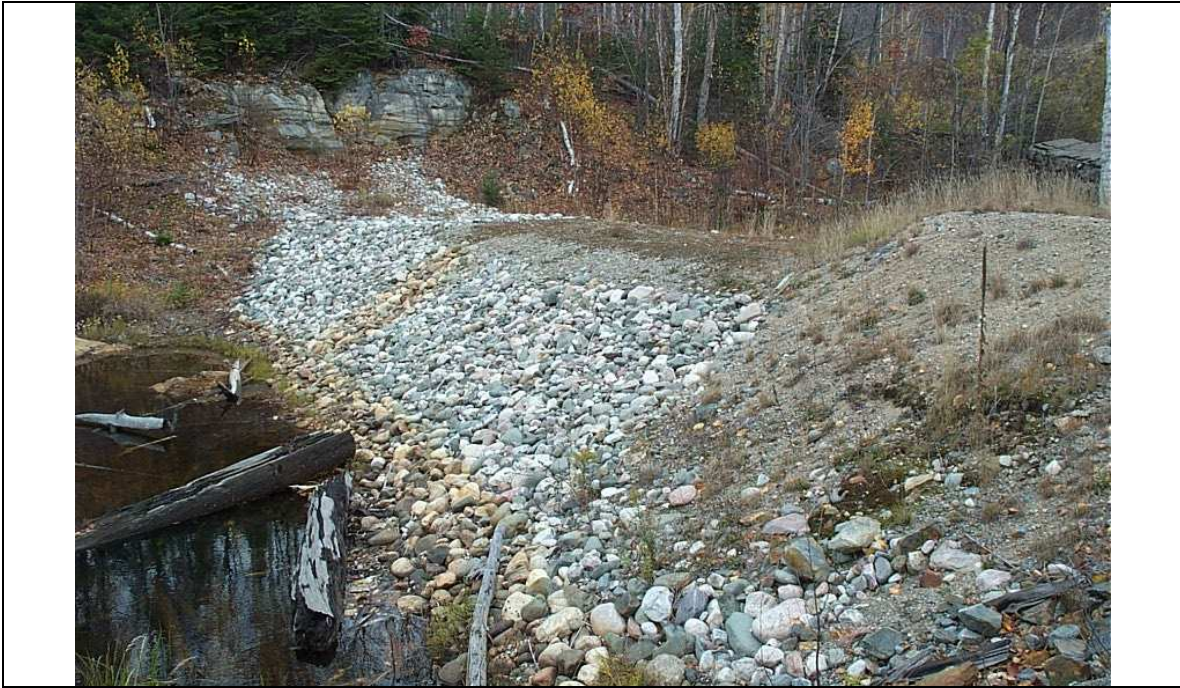
Photo 1: West Seepage Collection Pond Dam – Nordic TMA
