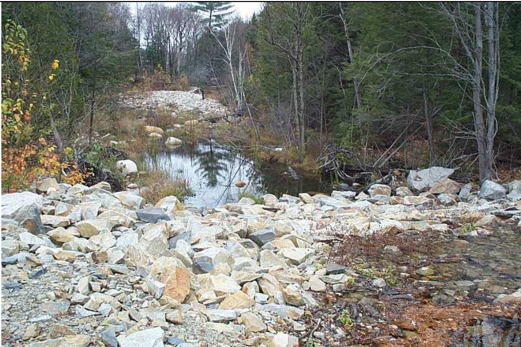
Photo 2: Rip rap lined spillway
