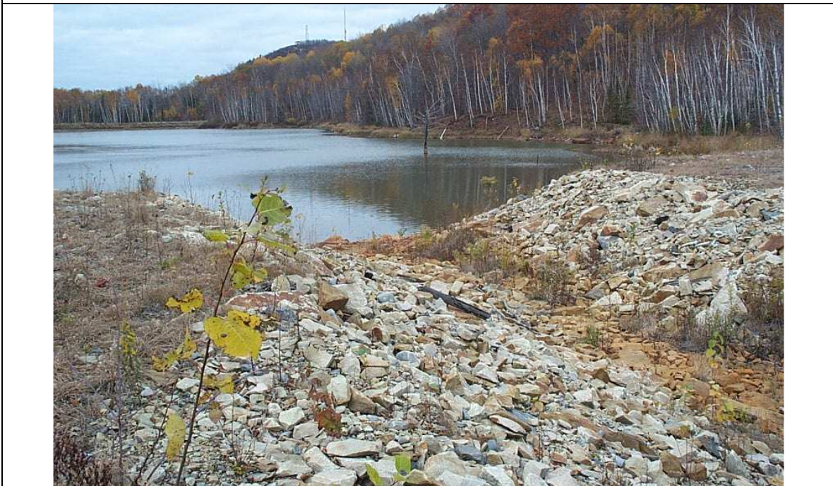
Photo 2: Spillway on Dam B – Nordic TMA
