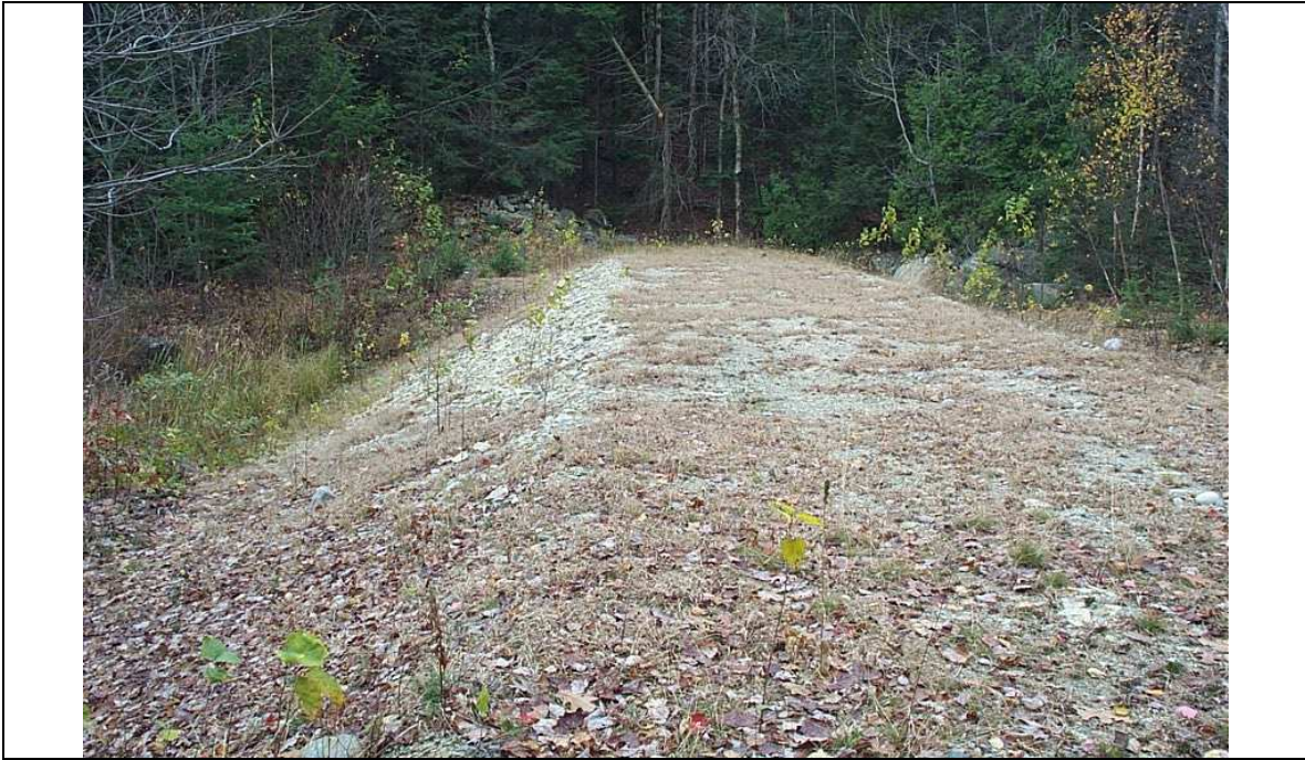
Photo 1: Nordic Settling Pond Berm – Nordic TMA
