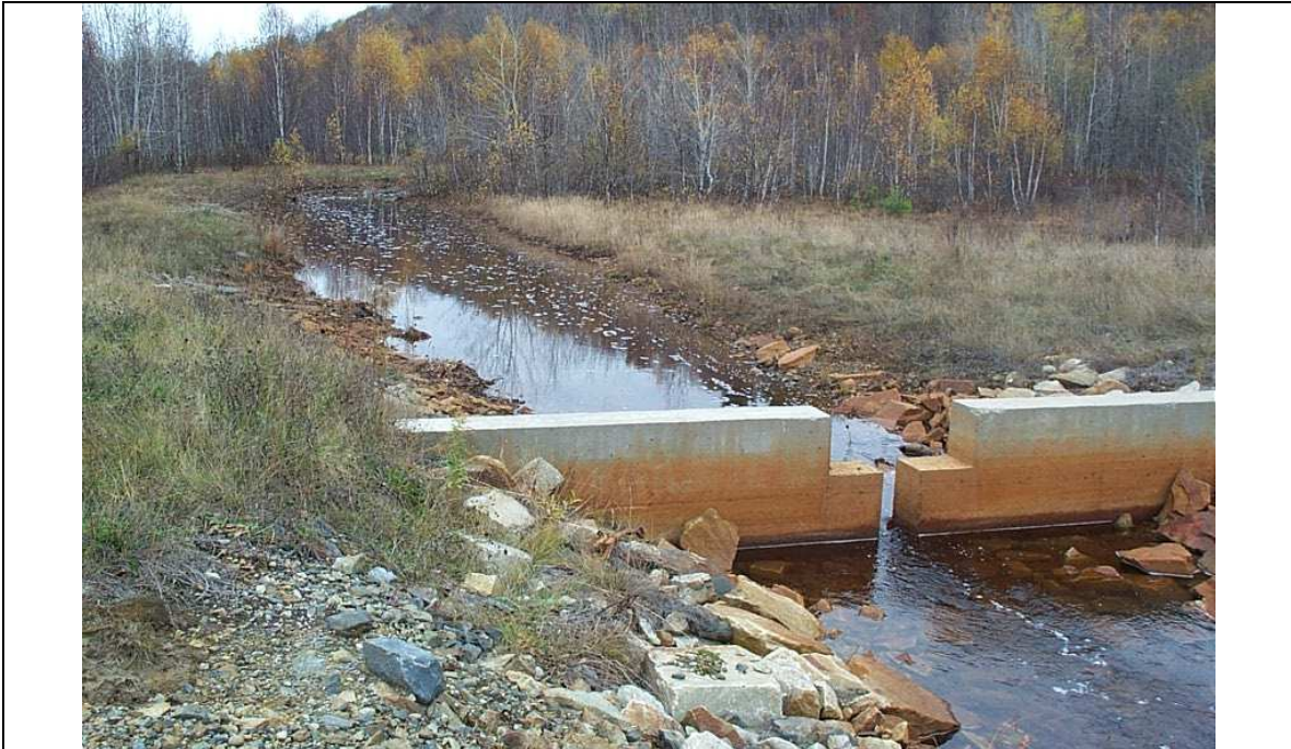
Photo 3: Dam F spillway flow control structure – Nordic TMA
