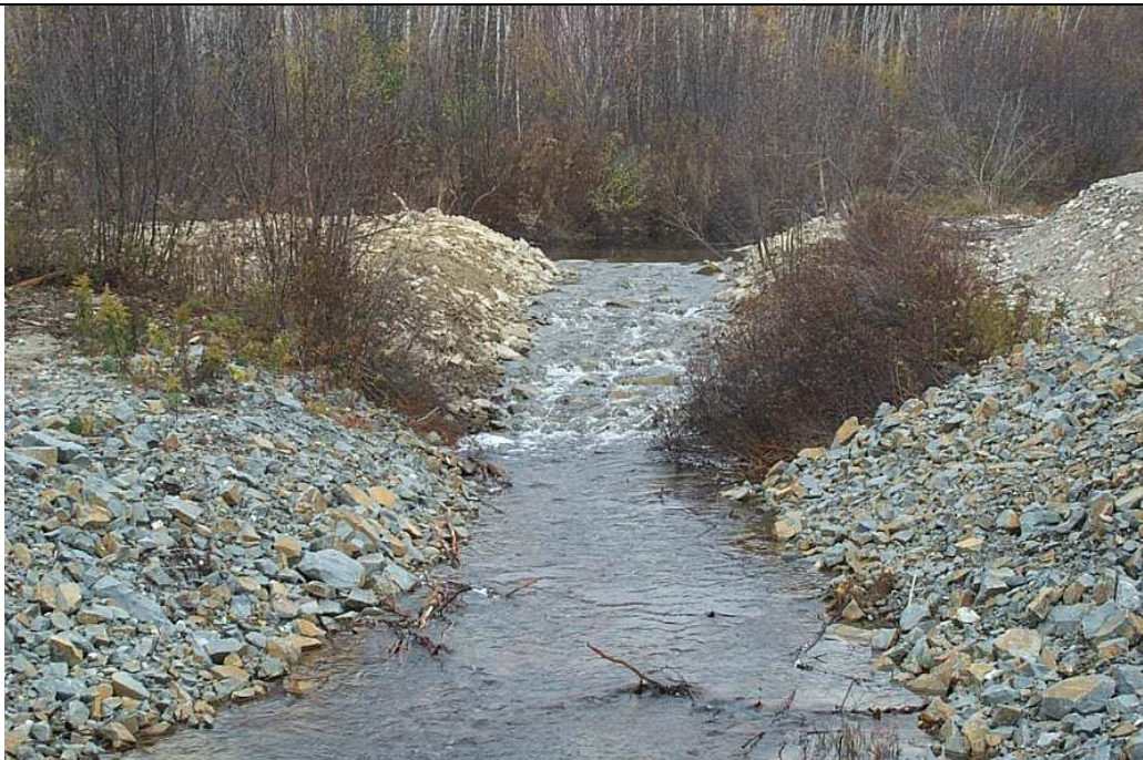
Photo 2: Looking upstream towards cofferdam
