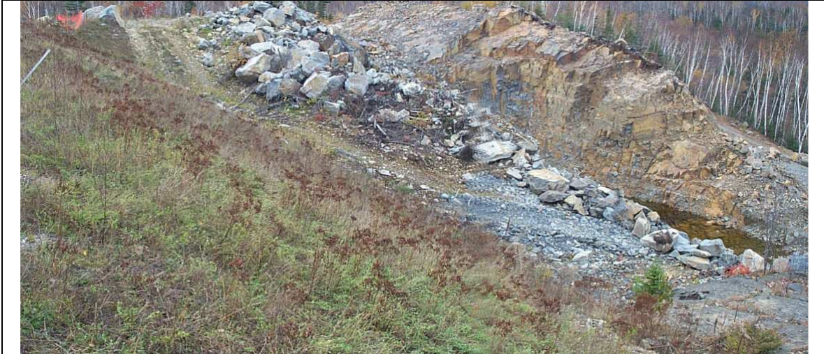
Photo 1: Dam D – Nordic TMA
