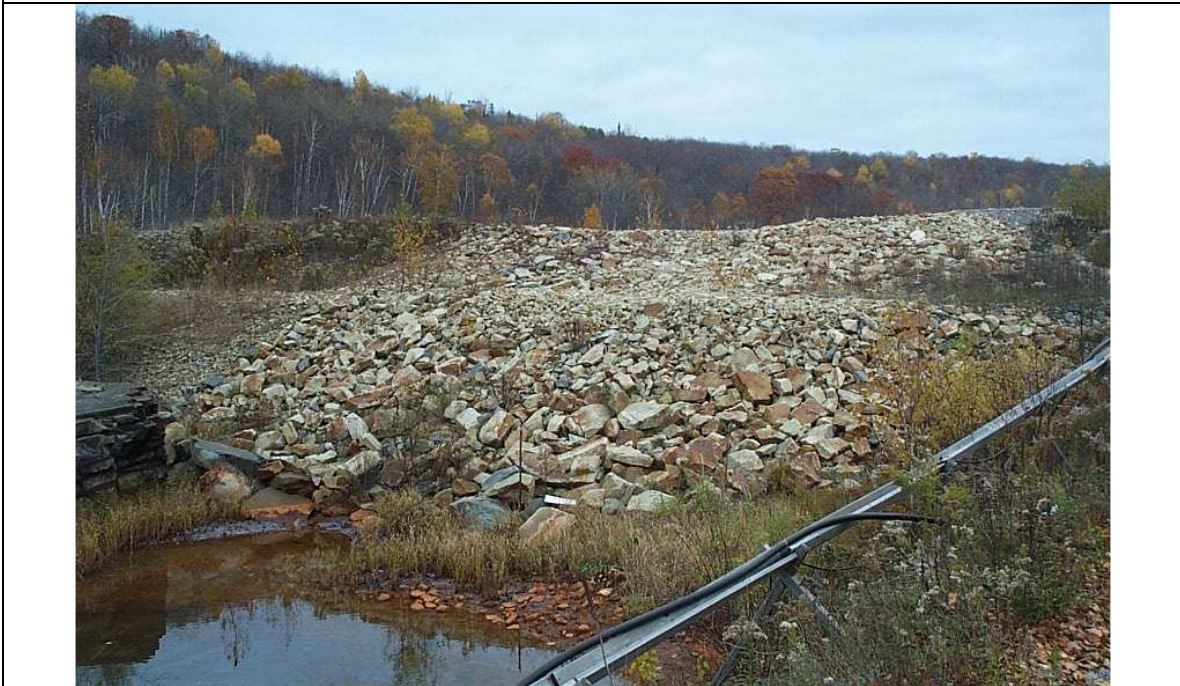
Photo 2: Downstream slope of Dam A – Nordic TMA
