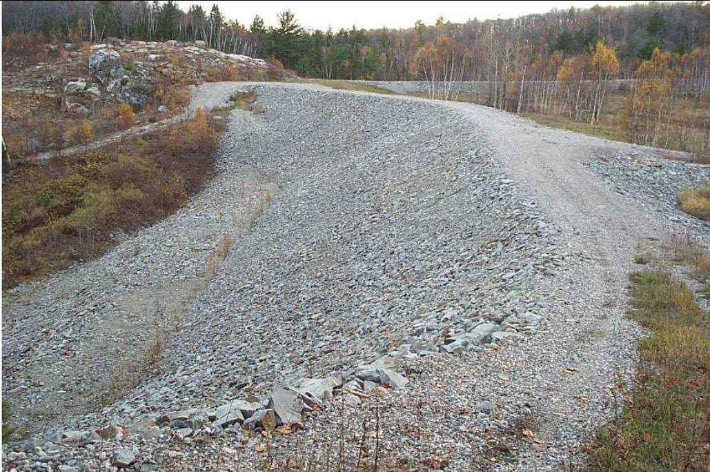
Photo 2: Dam A – Lacnor TMA
