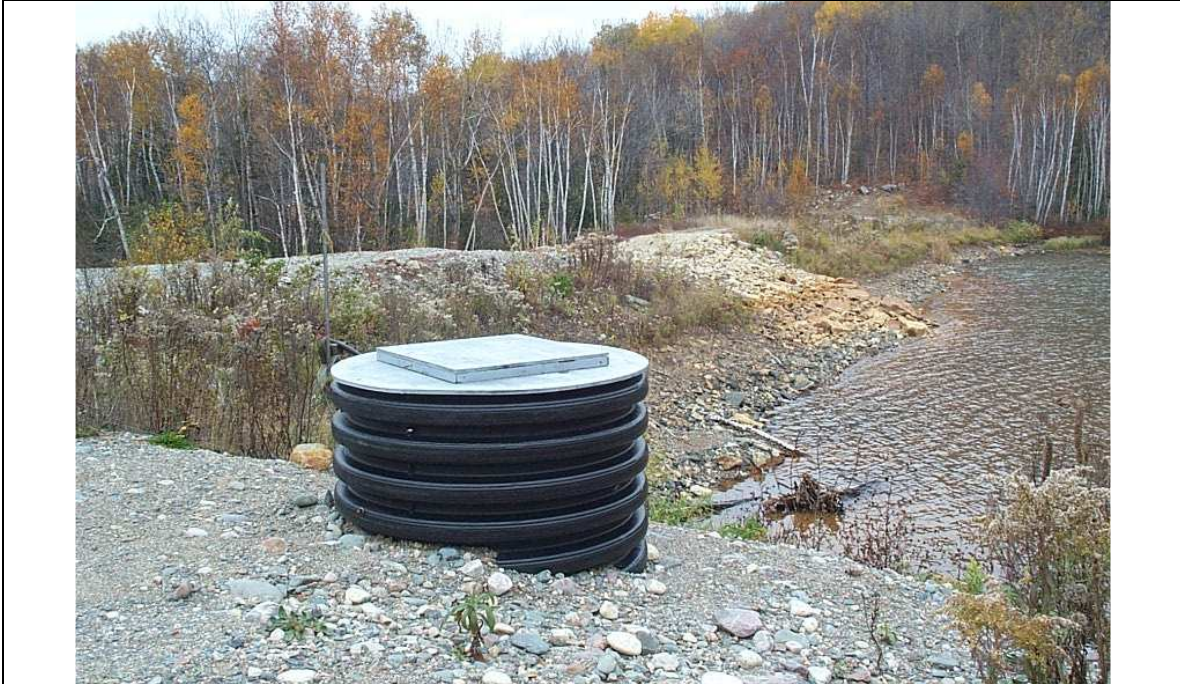
Photo 1: Dam A upstream view – Nordic TMA. Decant installed in 2006.
