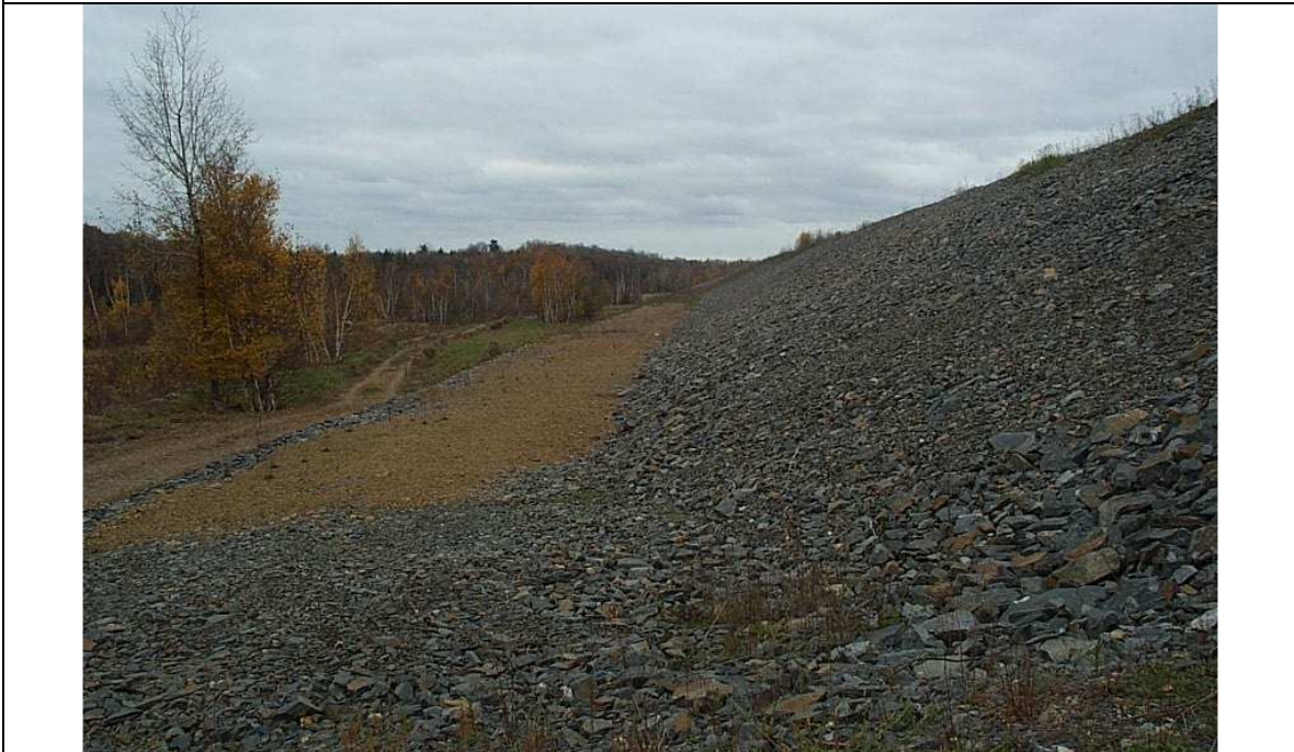
Photo 2: Dam F downstream slope looking from spillway – Nordic TMA
