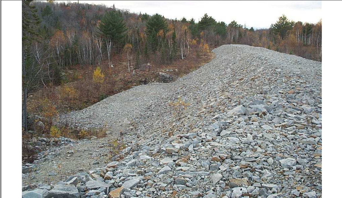
Photo 1: Dam B – Lacnor TMA
