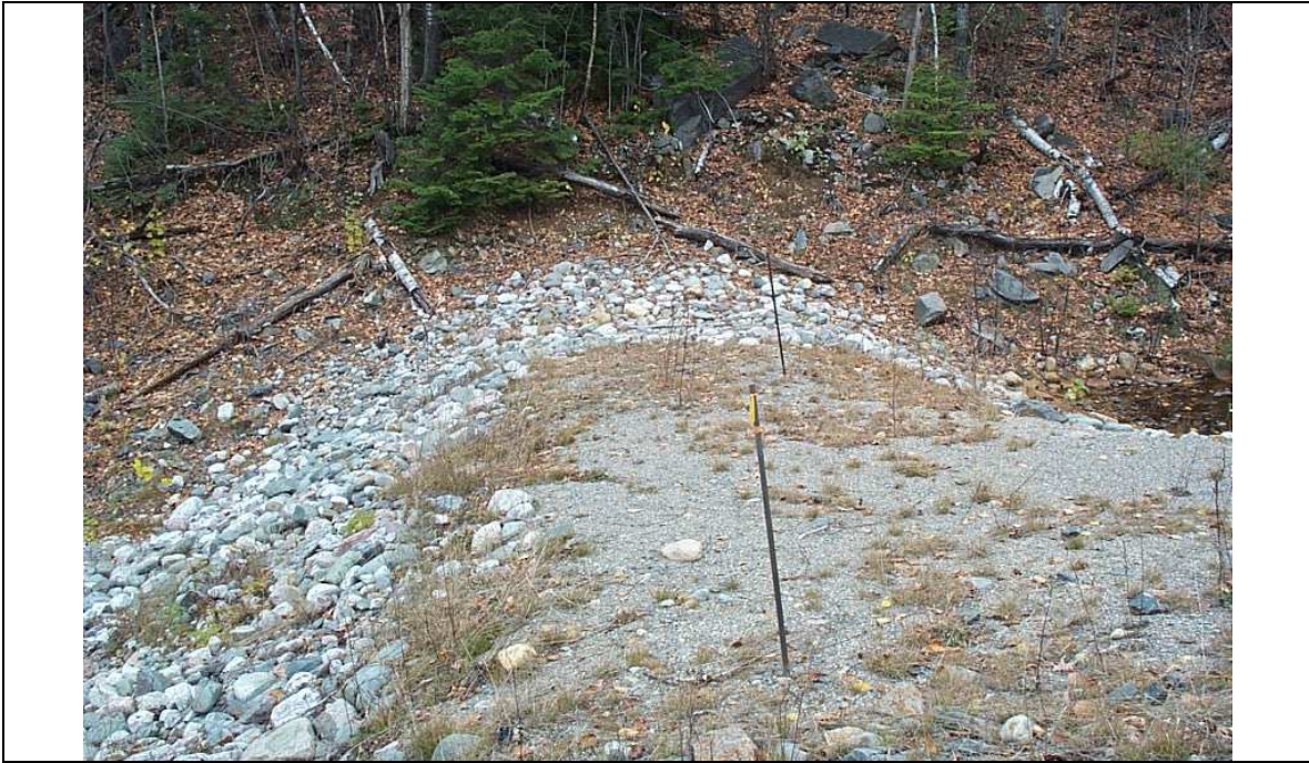
Photo 1: East Seepage Collection Pond Dam – Nordic TMA
