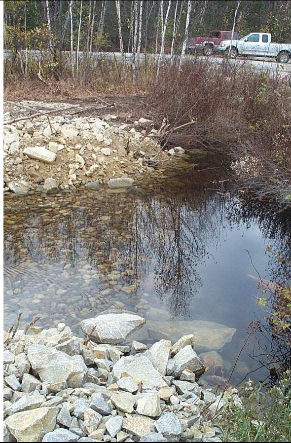
Photo 1: Cofferdam on Buckles Creek in placement of an old beaver dam
