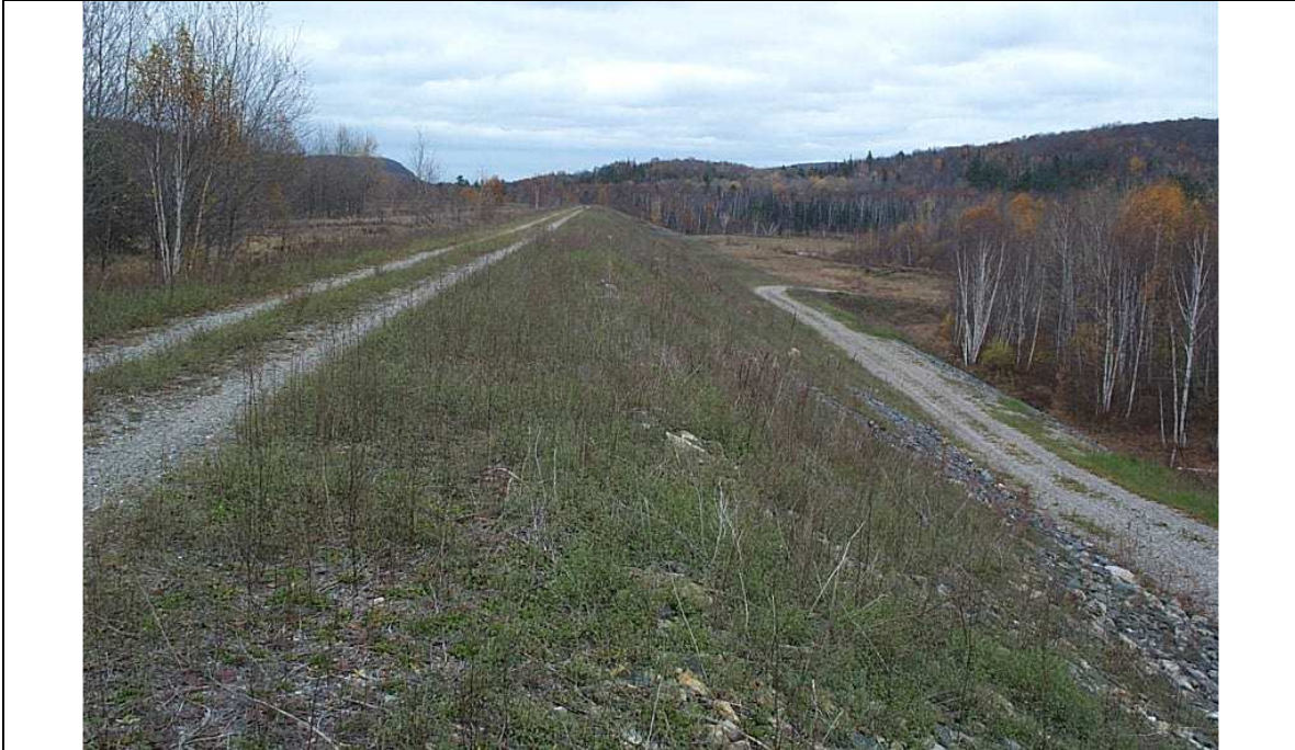
Photo 1: Dam F south arm – Nordic TMA
