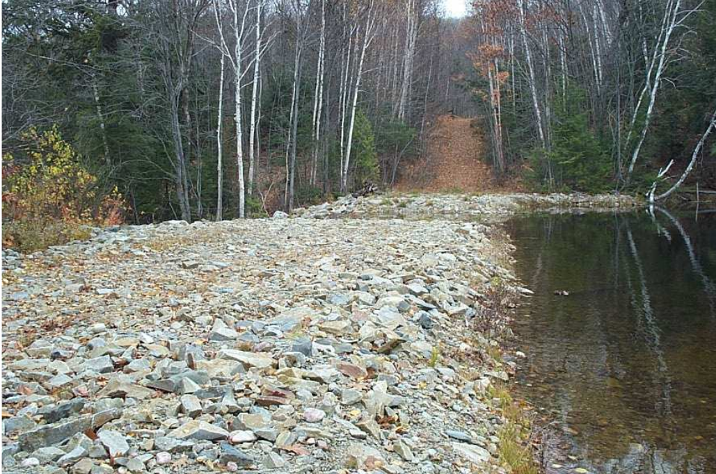
Photo 1: Upstream view of Westner Lake Outlet Berm
