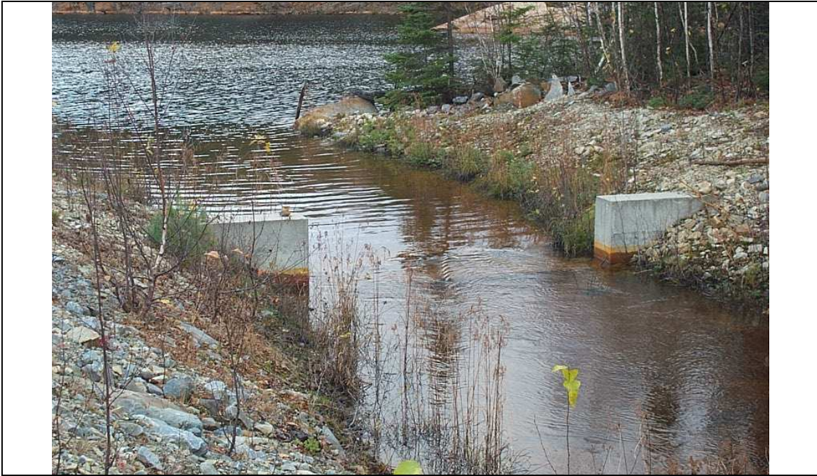
Photo 1: Tailings pond spillway inlet – Lacnor TMA
