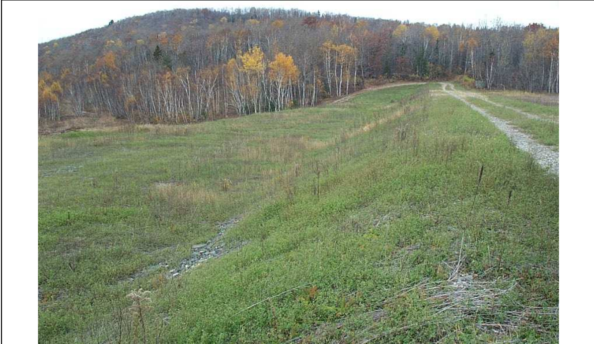
Photo 1: Dam C upper slope and toe buttress – Nordic TMA
