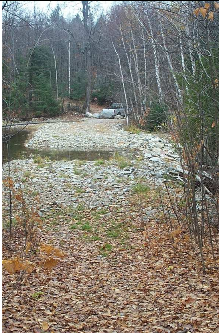
Photo 3: Water overflowing spillway on crest of dam
