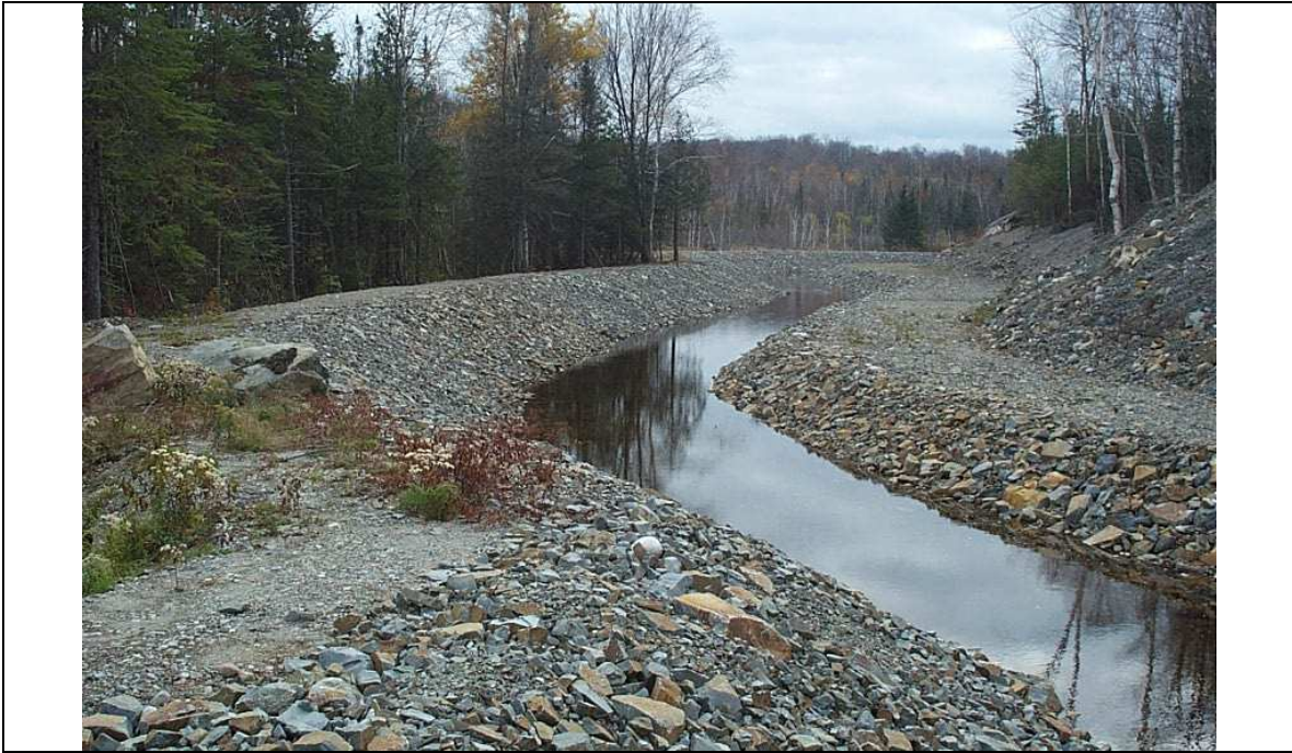
Photo 3: Buckles Creek Channel looking from Nordic Road.
