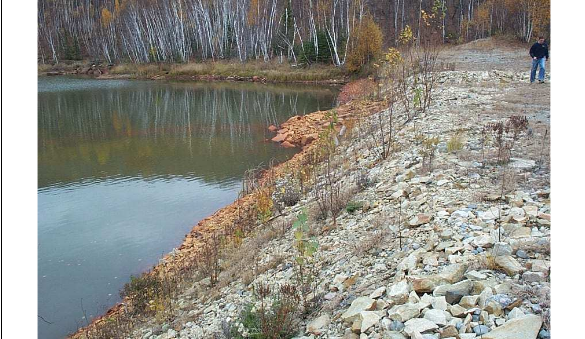
Photo 1: Dam B – Nordic TMA
