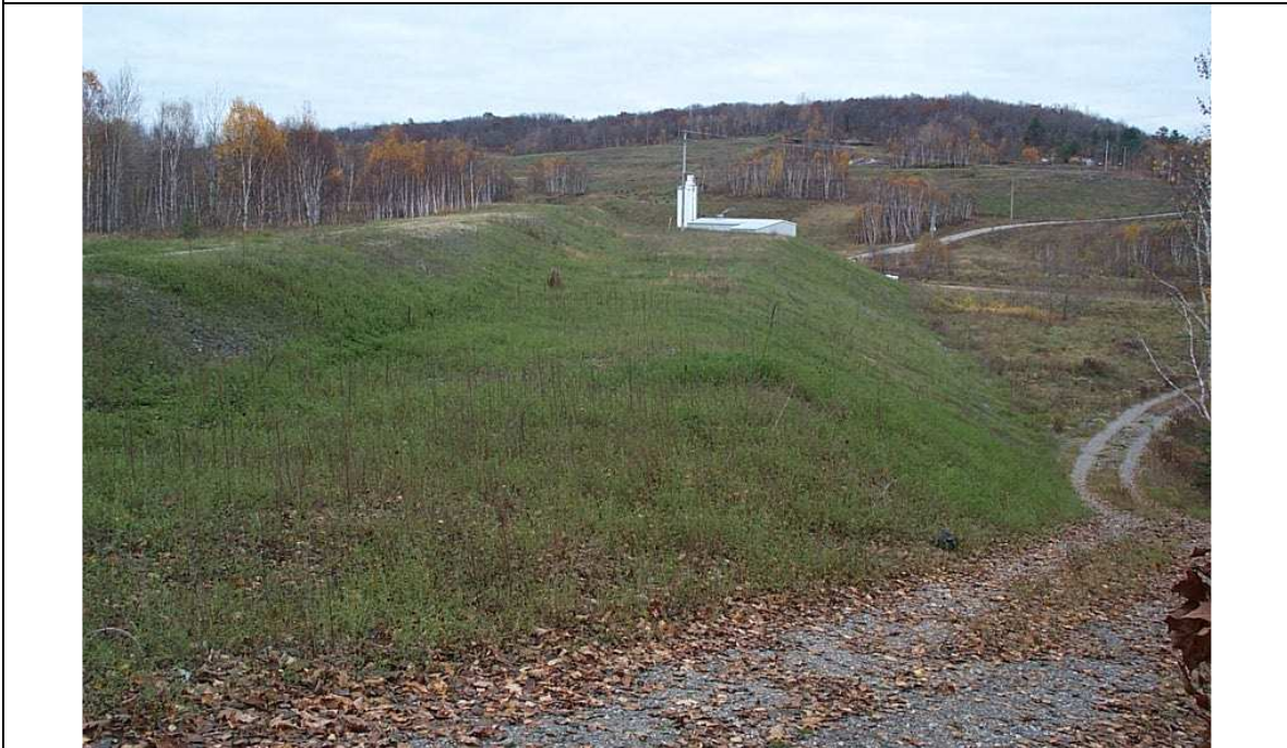
Photo 2: Dam C downstream slope – Nordic TMA
