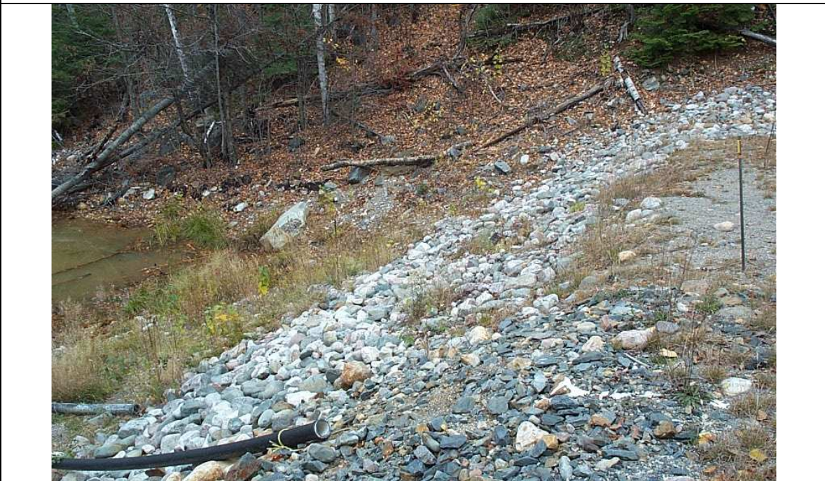
Photo 2: Downstream slope of dam – Nordic TMA
