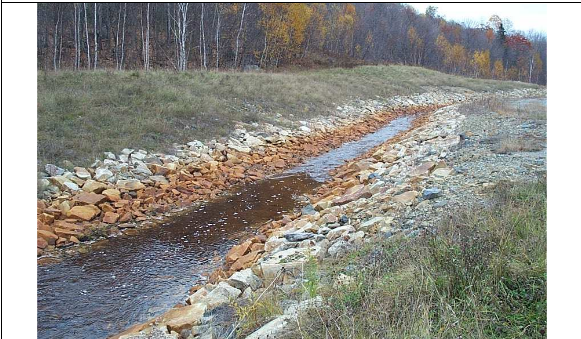
Photo 4: Dam F spillway outlet channel – Nordic TMA
