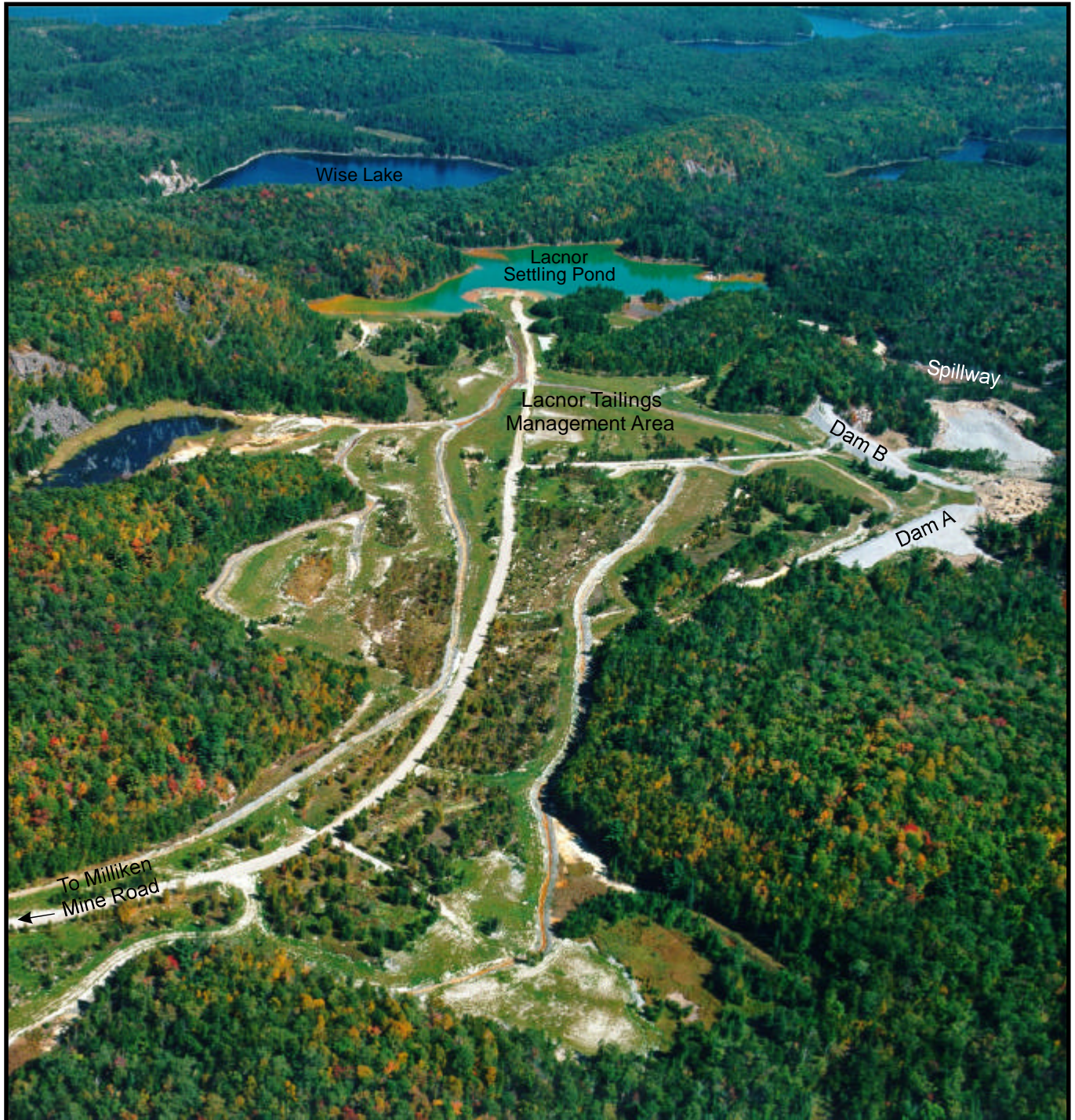
Lacnor TMA Looking to the North-East - September 1999
