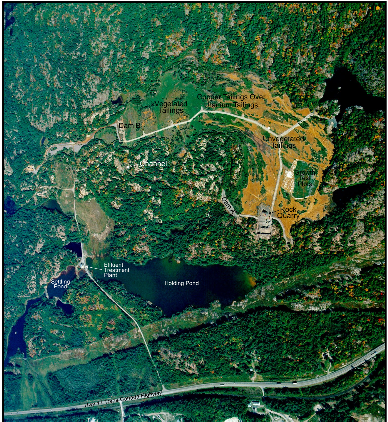
Pronto TMA Viewed From the South - September 1999
