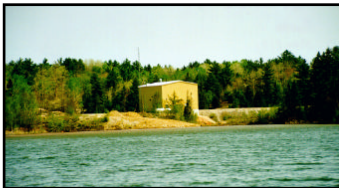
Pronto Effluent Treatment Plant 1997
