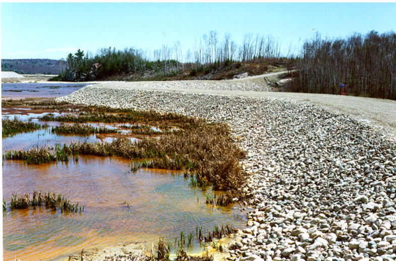
Upstream slope of completed dam
