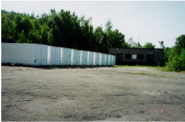
Licensed PCB storage site of specially modified containers; prior to shipping for disposal.
