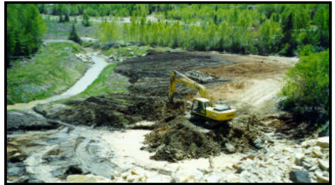
Nordic Dam E Toe Berm Upgrade 1999
