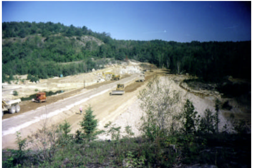
Dam nearing completion showing final slope
