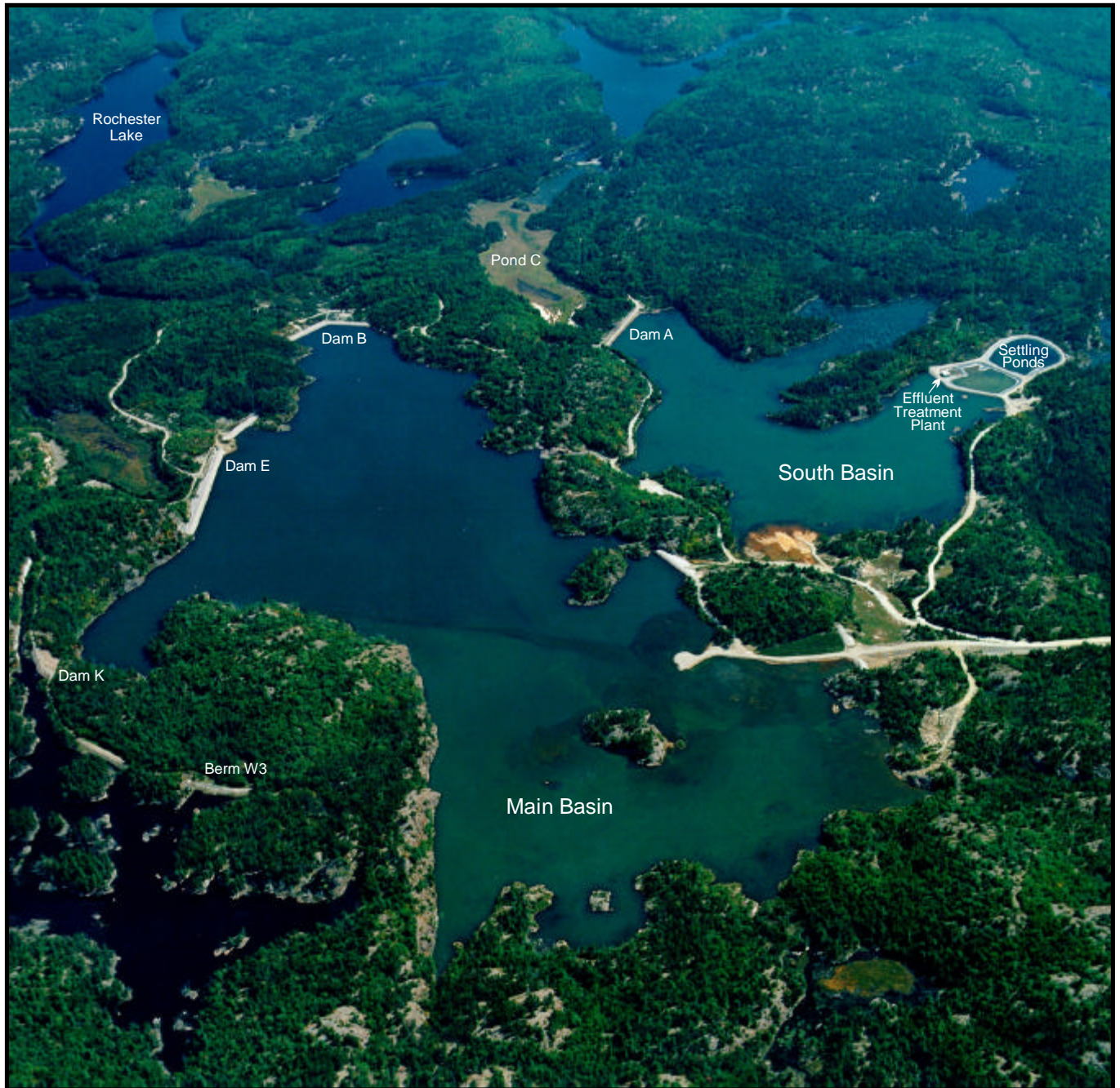
Panel TMA Viewed from the West - September 1999
