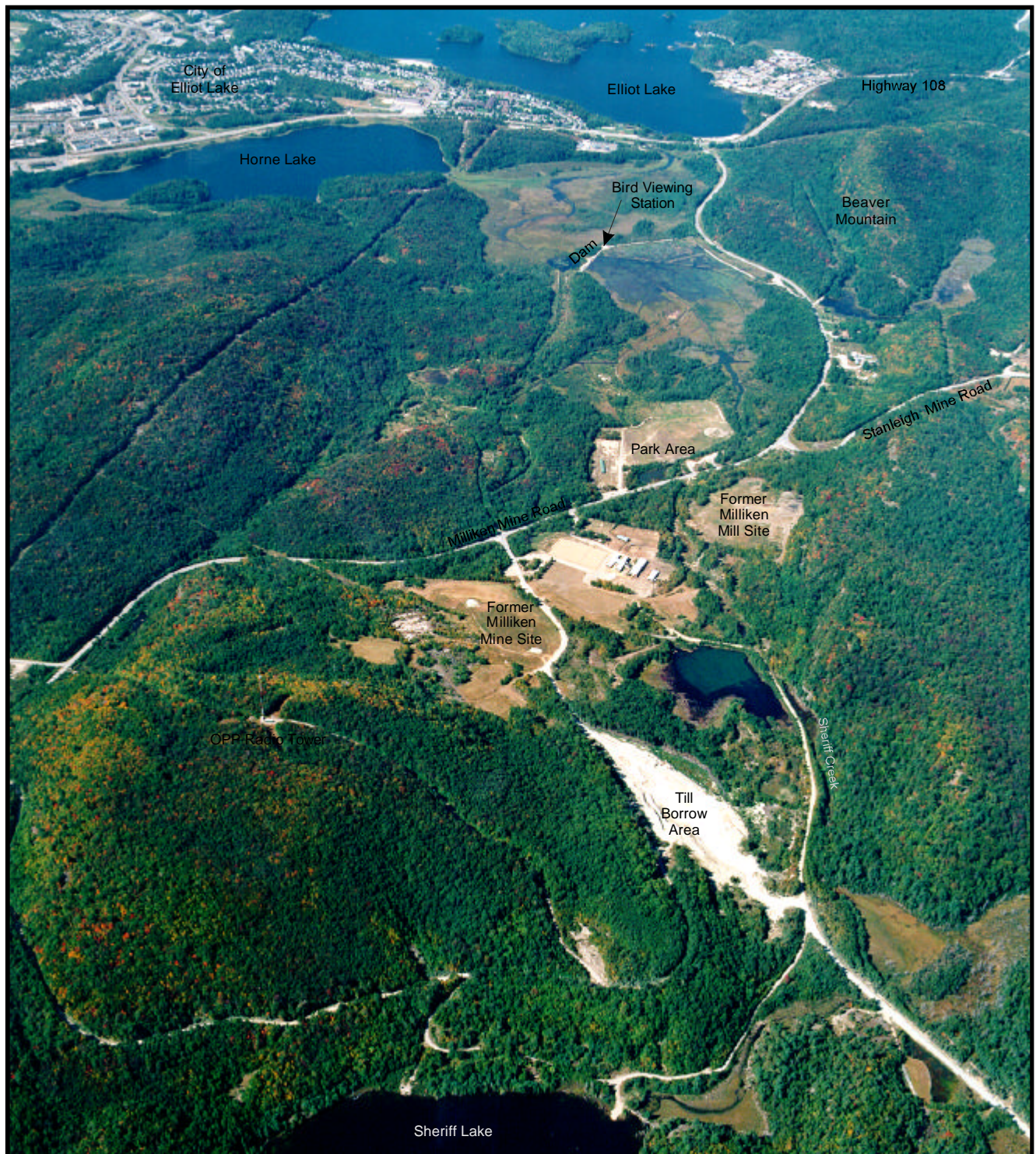
Milliken Mine and Mill Site Viewed from the East - August 1999
