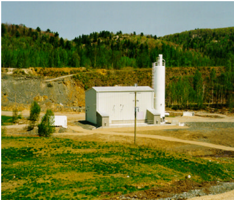
Effluent treatment plant, Nordic mine site
