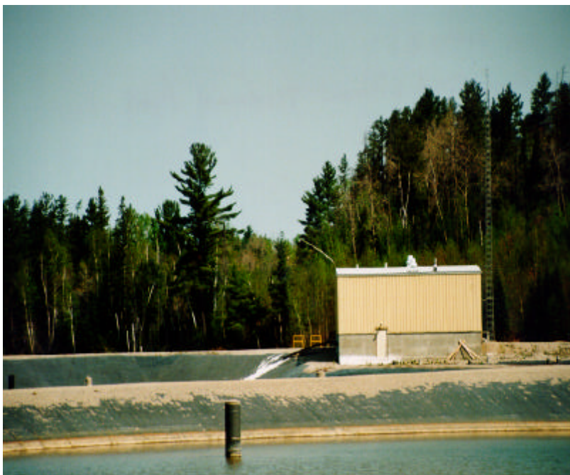
Effluent treatment plant, Panel tailings management area
