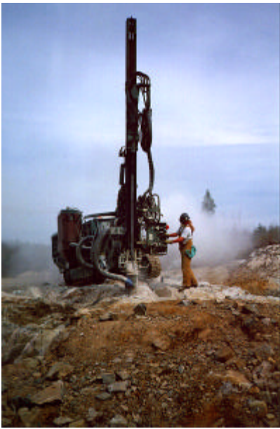
Bedrock drilling
