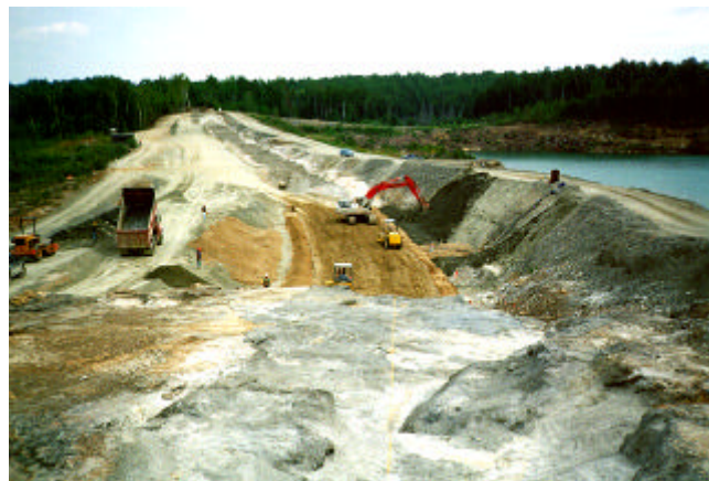
Dam building commences
