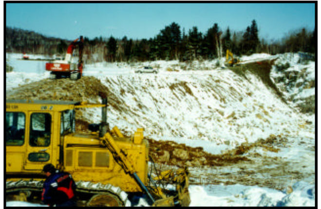
Lacnor Dam A Construction Winter 1999
