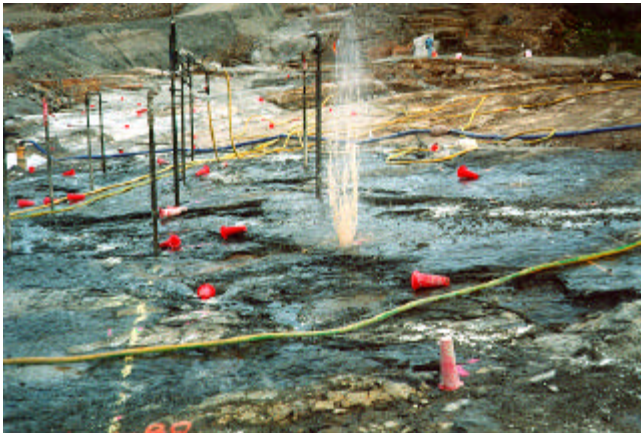
Grout hole testing and washing
