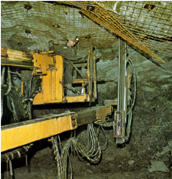
Rock bolting, Stanleigh Mine
