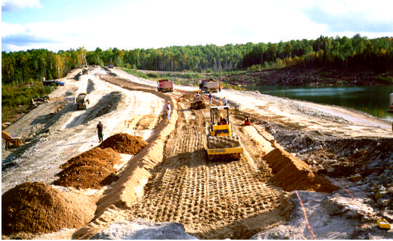
Dam construction well advanced
