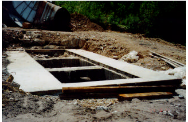
Placing reinforced concrete slabs on shaft collar.
