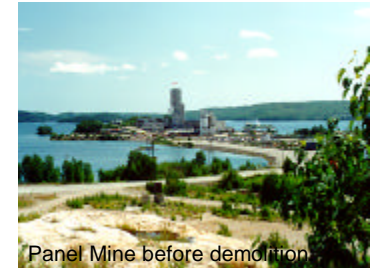
Panel Mine before demolition.
