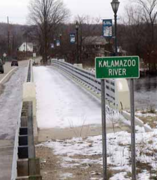
Cooperation among Cooper Township, Richland Township and the Michigan Department of Transportation made possible this safe, peddler/pedestrian crossing of the Kalamazoo River at D Avenue and allows for a loop of the Kalamazoo River Valley Trailway on both sides of the river.
