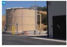
**Water desalination facility**. Chemicals are delivered to the WDTF at outdoor connections (6). Source water is pressurized through the desalination plant via these feed pumps (7). First stage EDR demineralization system (8) with the reject concentrated by the VSEP RO system (9). The concentrated brine is stored in a tank for off-haul disposal (10).
