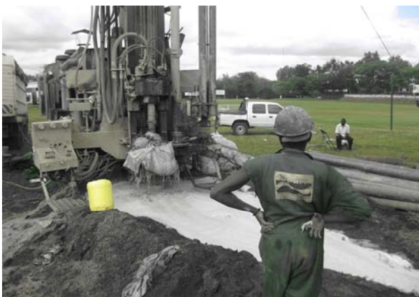
Borehole being dug at the RFUEA Grounds
