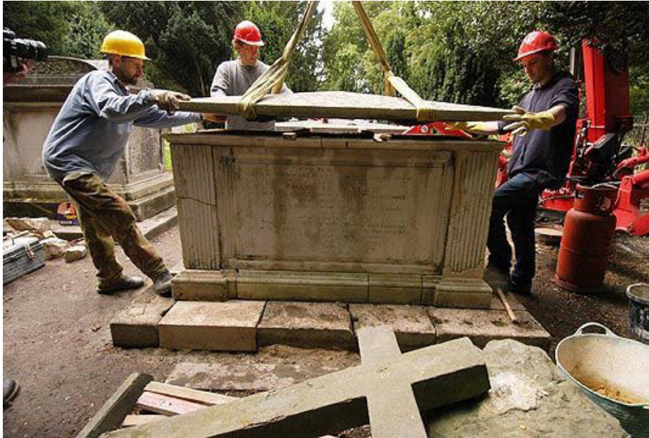
Above: the top slab craned back into position
