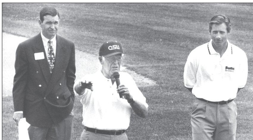
Athletic director Mitch Barnhart, John Goss and Pat Casey at the groundbreaking for Goss Stadium at Coleman Field in 1998
