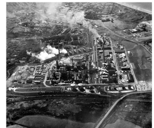
Figure 5: Historic image of nylon works
