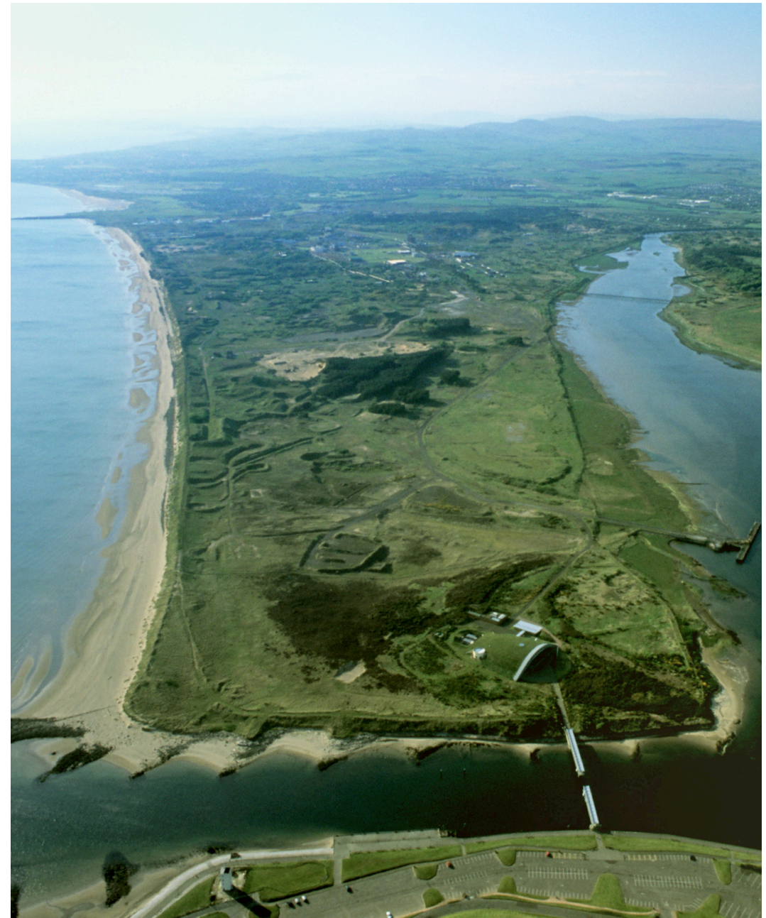
Figure 19: Aerial view of the Ardeer Peninsula
