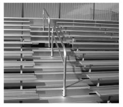
Four foot aisle with aluminum handrails and steps with marked front edges. Uniform seat slope increases safety when walking up or down bleachers.
