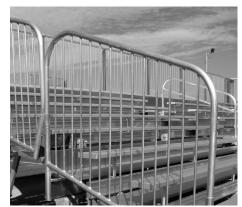
Spectator-friendly rounded aluminum guardrails with vertical balustrades.
