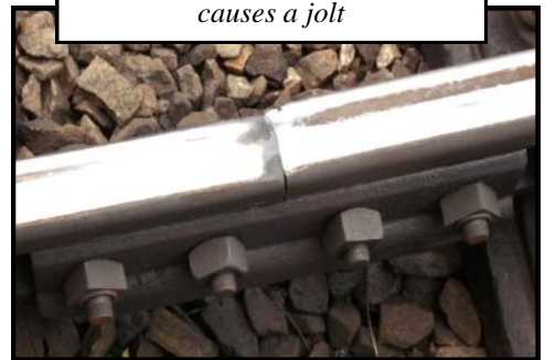
Two rail joints at Stourbridge Junction station: above, the rail ends are misaligned, causing the railcar to lurch; below, a 'dropped joint' which causes a jolt
