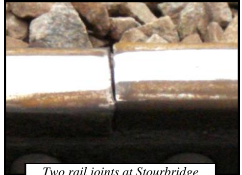
Two rail joints at Stourbridge Junction station: above, the rail ends are misaligned, causing the railcar to lurch; below, a 'dropped joint' which causes a jolt
