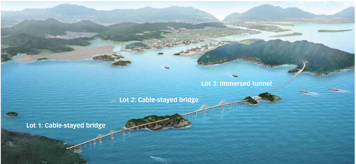
The Lot 1 cable-stayed bridge is 1.65 km long that has approach viaducts between Jeo and Geoje islands. The Lot 2 cable-stayed bridge is 1.87 km long and has viaducts between Jungjuk and Jeo islands. The Lot 3 immersed tunnel is 3.2 km long.
