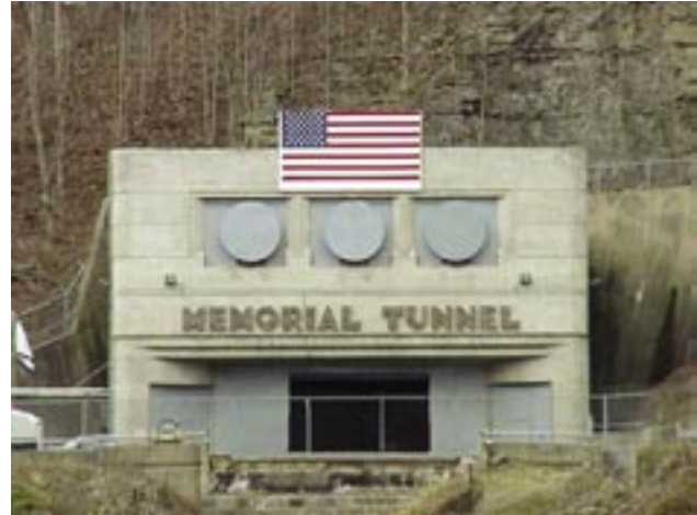
East portal of Center for National Response (Memorial Tunnel)
