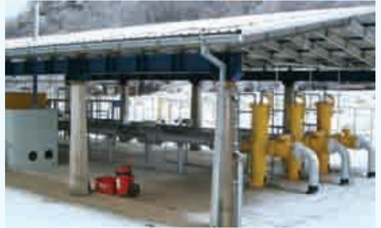
The Makpetrol Border Station in Macedonia uses Daniel SeniorSonic meters for primary flow measurement
