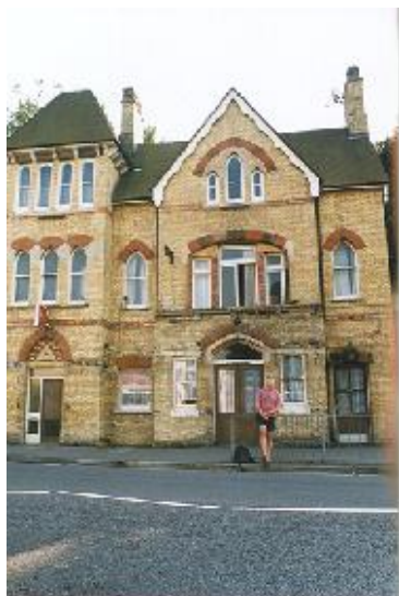
Fig. 18 Railway and Bicycle Public House
