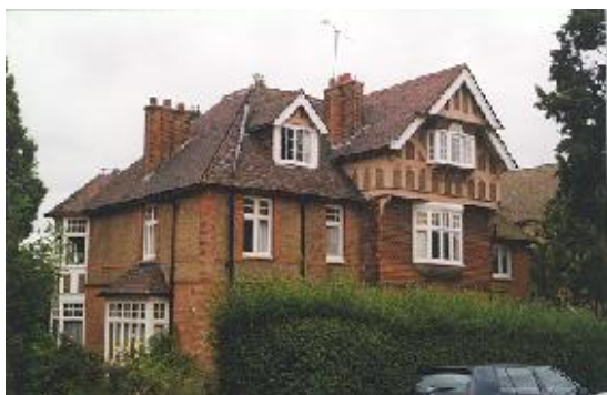
Fig. 4 One of the Larger Villas
