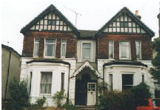
Fig. 15 Deterioration of two Granville Road villas
