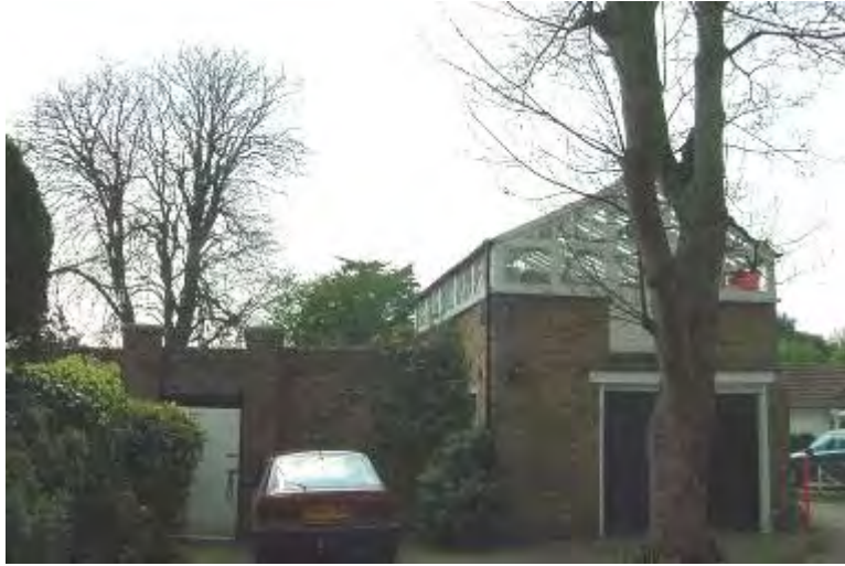
Former Coach House, 27 Streete Court
