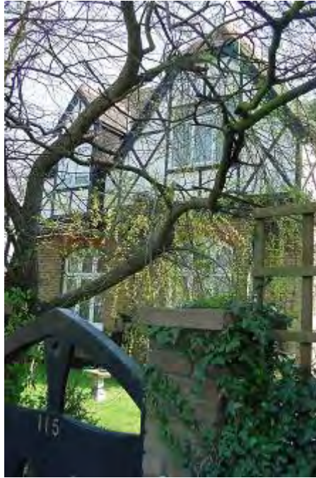
Former Lodge to Westgate House
