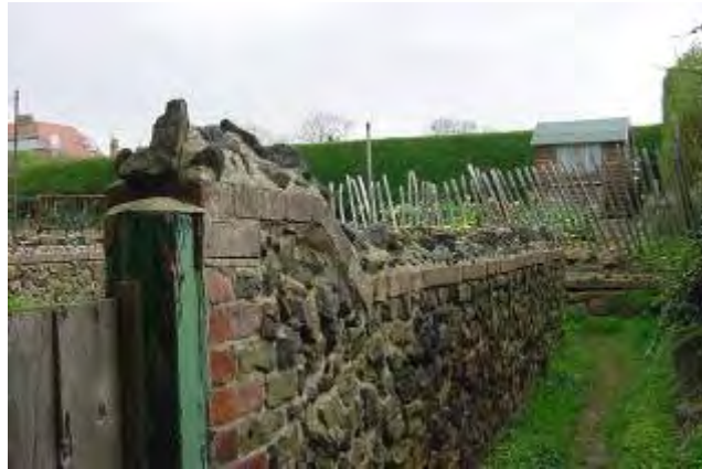
Rear Gardens 5-33 Quex Road
