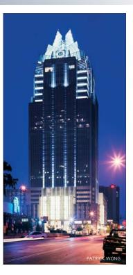
Layered lighting reinforces Frost Bank's design by weaving together its base, tower, and top. Above the glass screens, 4200K sources highlight vertical and horizontal bands. The faceted glass crown is also backlighted using shielded metal halide floodlights. This attention to transition leads the eye seamlessly from bottom to top.
