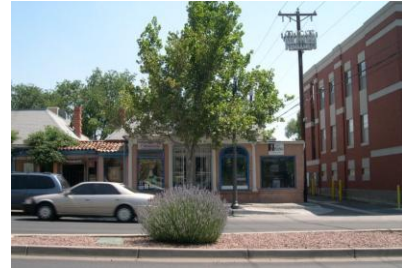
Photograph 10.a. Residential-Commercial structure perhaps a century older than its new neighbor.
