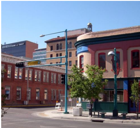
Photograph 29. An example of “tarting up” to appeal to era’s aesthetic; painted brick façade. Note modern high rise structures a block or two south.
