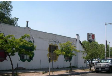
Photograph 4. Bakery, converted to a theater. Front, retail store is vernacular Cottage Architecture; unique, eye catching, European.
