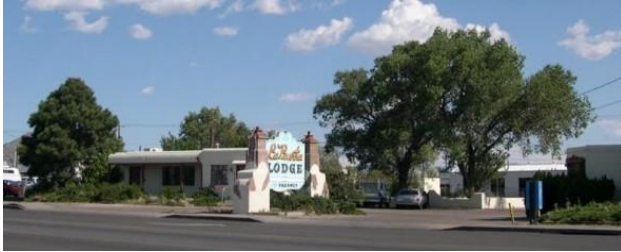
La Puerta Lodge, East Central. Still in operation, in good repair.
