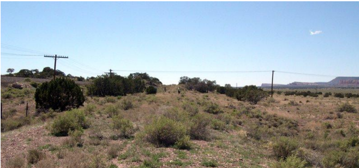
Photograph 24. The early alignment, looking westward from the bridge. The space between the vegetation is where the roadbed lies atop an earthen berm. In the high desert, evidence of soil disturbance remains for centuries.
