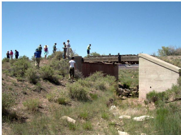
Photograph 22. Bridge built in about 1905, part of early alignment pre-dating Route 66.
