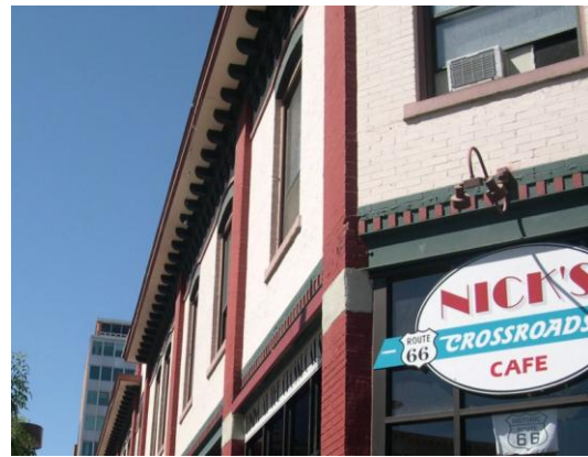
Photograph 32.a. Nick's Crossroads Café, and building detail to south.
