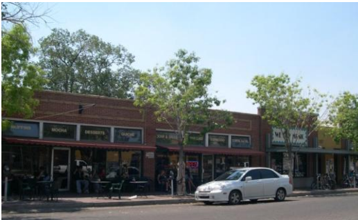
Photograph 3. Decorative brick façade, street wall, Harvard at Central.
