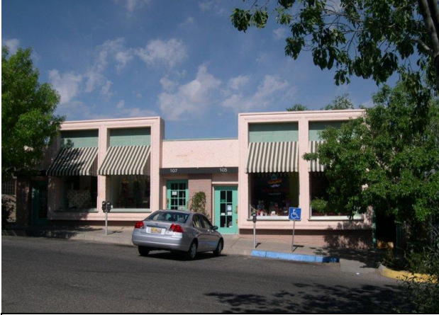
Photograph 37. This example of early architectural design is not yet protected for preservation. Documentation is needed.
