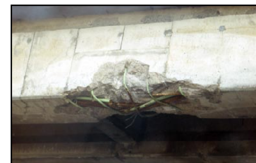
Patch repair over Hwy 401 east bound
