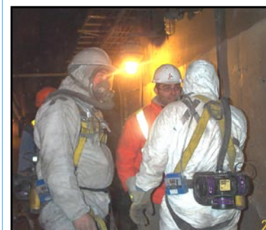
Pre-entry meeting for plenum confined space entry @ Thorold tunnel
