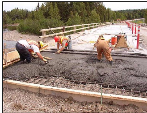
Approach slab at Bearberry
