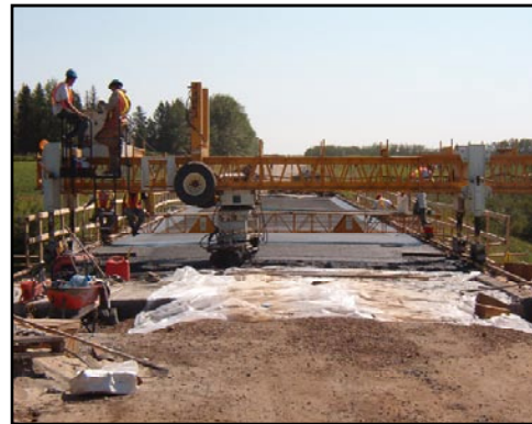
Deck Finishing at Castor
