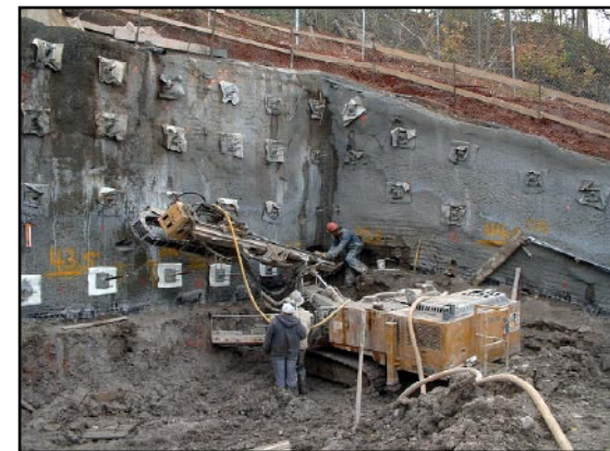
Versatile drill working in the SW corner
