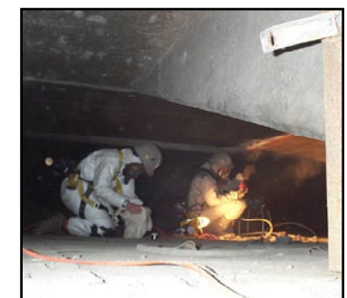
Mock demolition to allow personal air quality testing
