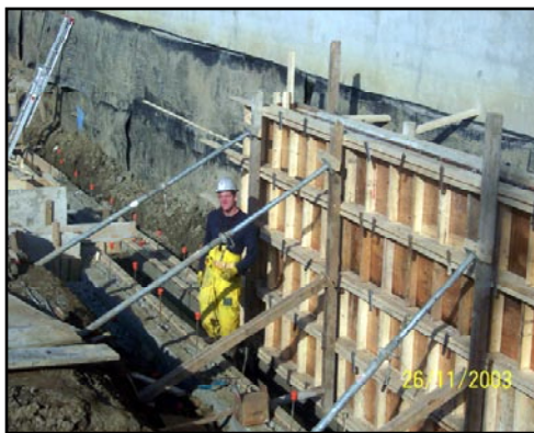
Forming and placement of reinforcing steel
