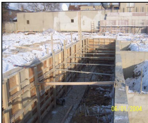
Foundation wall ready to be poured
