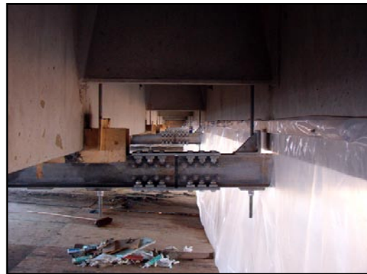
Grouting of the underslung diaphragms at Bearberry
