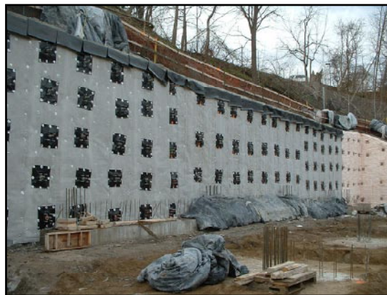
Completed soil nail wall with waterproofing membrane
