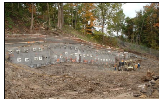
Installing soil nails in the south wall
