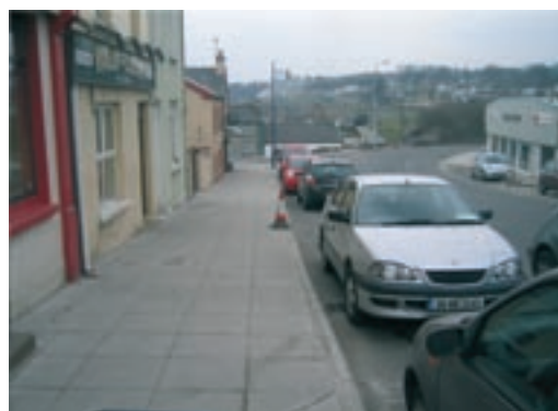
PHOTOGRAPHS OF SUBSTANTIALLY COMPLETE SCHEME AT ARDARA (PHASE I)
