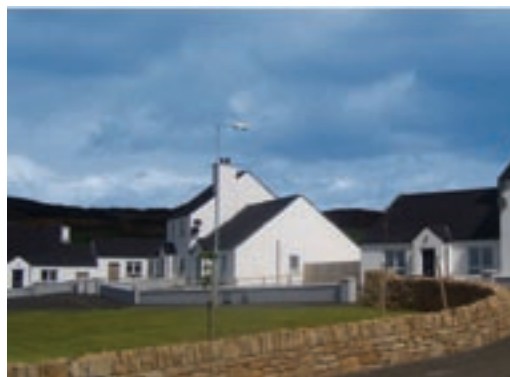
SOCIAL HOUSING SCHEME AT MALIN
