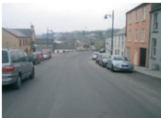
PHOTOGRAPHS OF SUBSTANTIALLY COMPLETE SCHEME AT MOVILLE (PHASE II)
