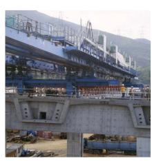
▲ The chords of the launching gantry are 85m long, twice a span length
