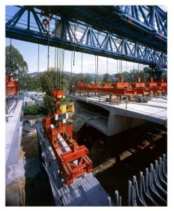
▲ 14 pre-cast segments for each span
