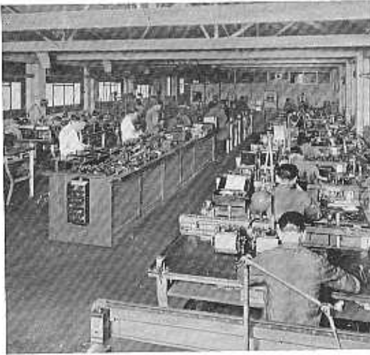
Assembling electrical instruments
