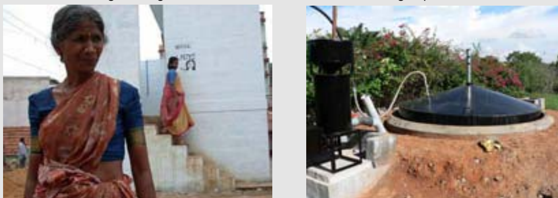
Figure 31: Urine diverting public toilet in Bangalore (left; Heeb); biogas plant (right; Wafler)
