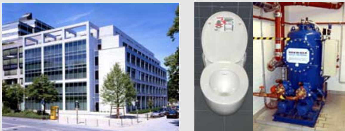
Figure 19: KfW office building “Ostarkade” (left); Vacuum toilet and pumping unit (right) (KfW)
