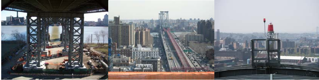
Contract #8 in 2008: East River Park Piers. Manhattan Approach. Aviation Light on the Manhattan Main Tower.
