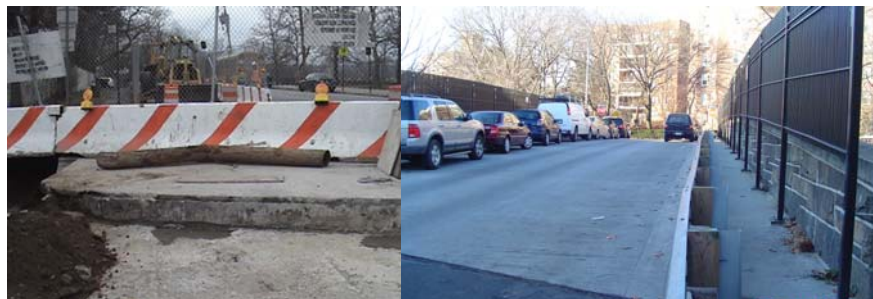
Manhattan College Parkway Bridge Deck During Construction. Completed Bridge.
