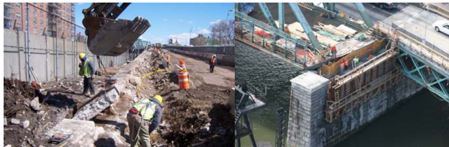
2006: Demolition of 145 th Street Bridge Manhattan Approach. Aerial View of Construction.
