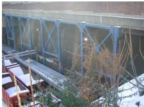
West 31 st Street Bridge in 2004. (Credit: NYSDOT)
