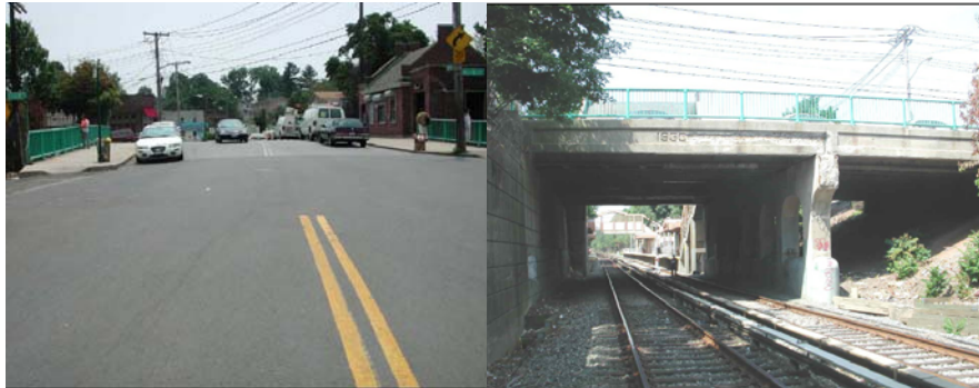
Annadale Road Bridge in 2001. (Credit: NYSDOT)
