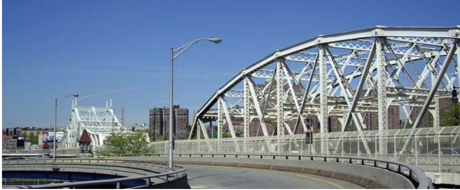
Macombs Dam Bridge in May 2007.
