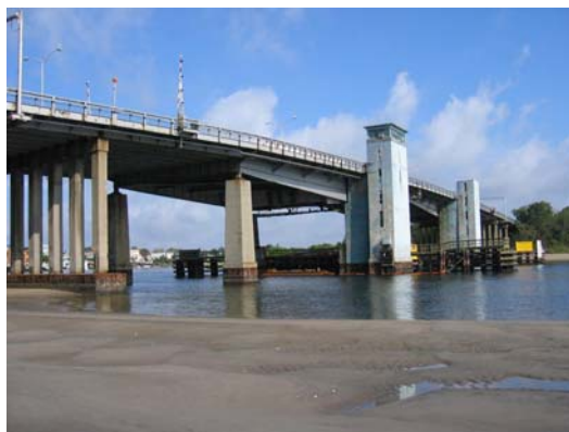
Belt Parkway Bridge Over Mill Basin.
