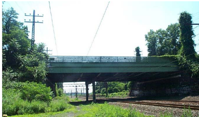
Shore Road Circle Bridge in 2003. (Credit: NYSDOT)
