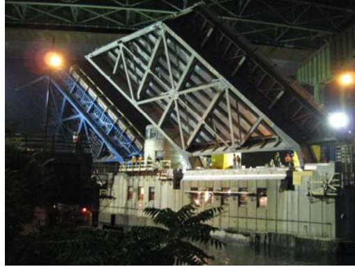
Open Hamilton Avenue Bridge in August 2007.
