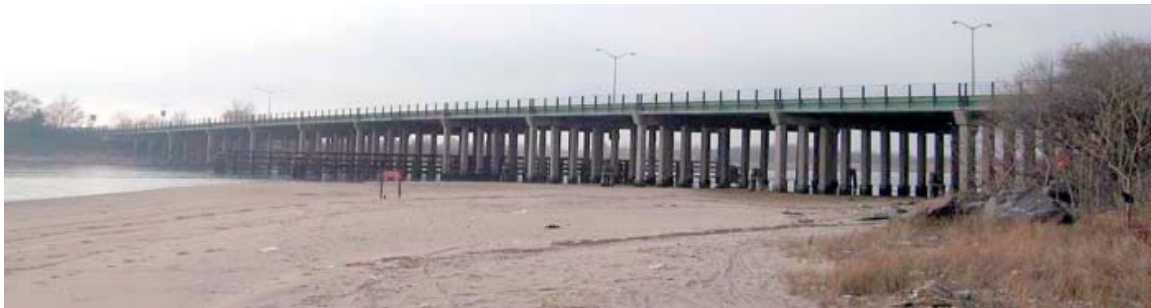
Paerdegat Basin Bridge.
