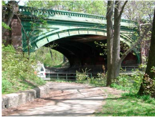
Hill Drive Bridge in 2001. (Credit: NYSDOT)
