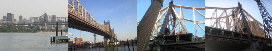
Protective Coating in 2007: Middle and Last Part of the Year.
