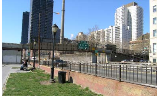
East 78 th Street Bridge.
