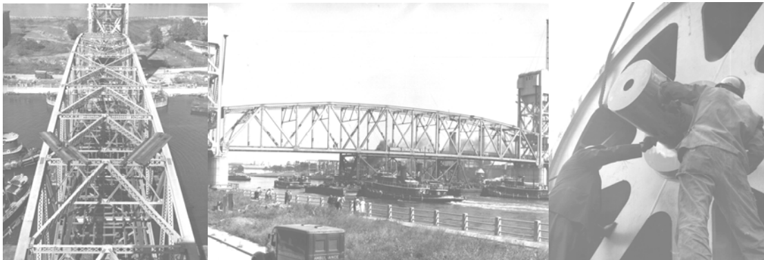
Roosevelt Island Bridge Under Construction in 1952.
