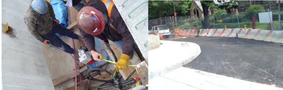
West 252 nd Street Bridge: Transverse Post-Tensioning of the Pre-Cast Concrete Beams in March 2007. Installed Asphalt on Bridge Approach in July 2007.
