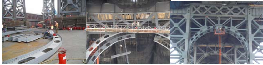
Contract #8 in 2005: Preassembling and Erecting Brooklyn Intermediate Tower Arch Steel.
