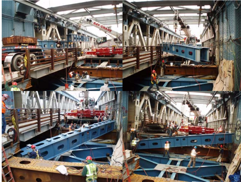
Contract #11 in 2006: Sequence of Installing New Double Floorbeam at Brooklyn Tower.
