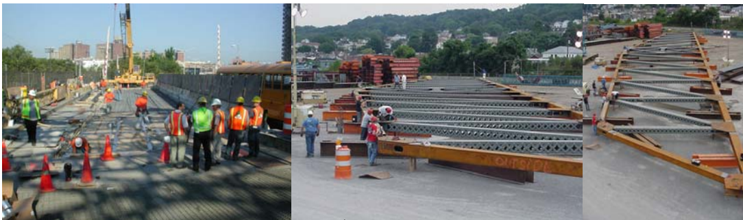
2005: Replacing Span #3 of the 145 th Street Bridge. Swing Span Truss Assembly.
