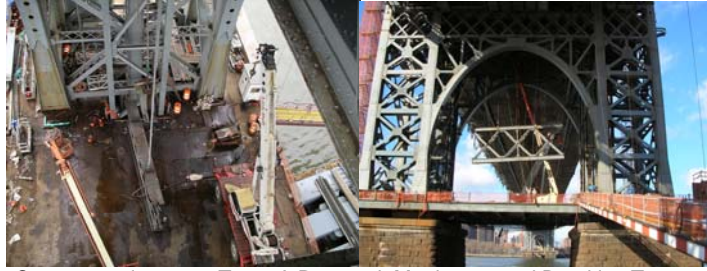
Contract #8 in 2006: Truss A Removal, Manhattan and Brooklyn Towers.
