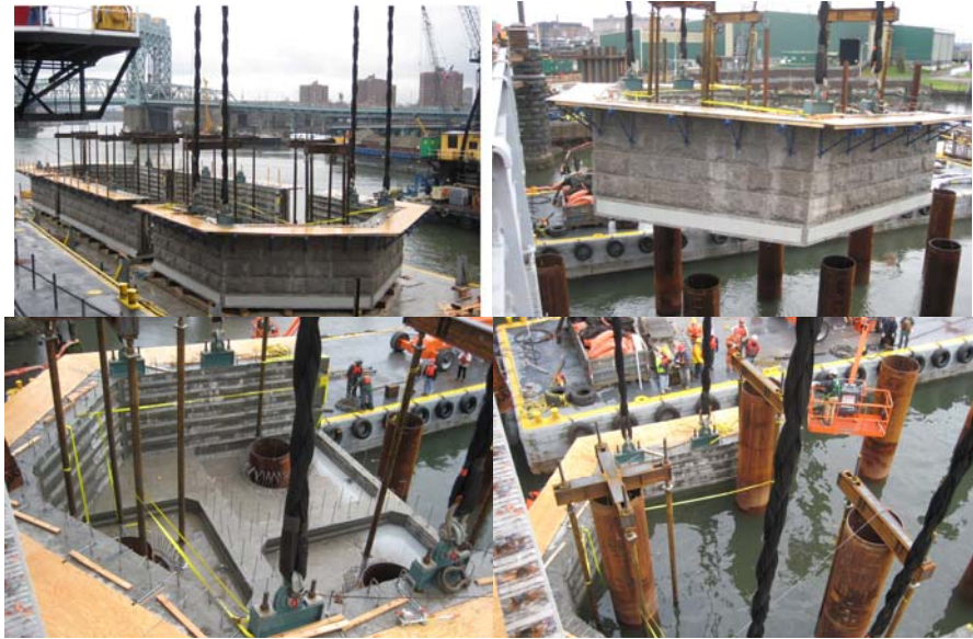
The First River Pier in November 2008.
