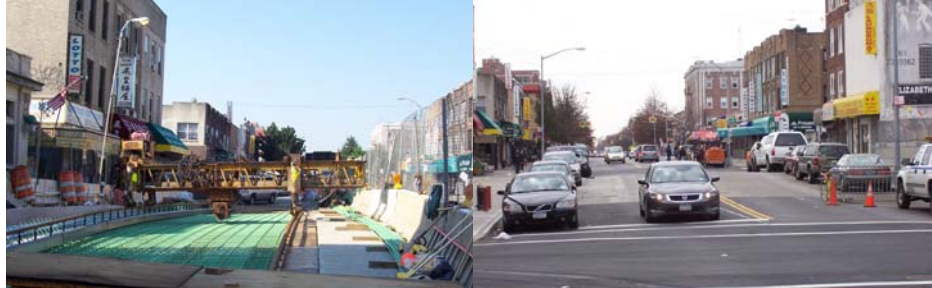
Installation of Slab Rebars in August 2008. New Bridge Open to Traffic.
