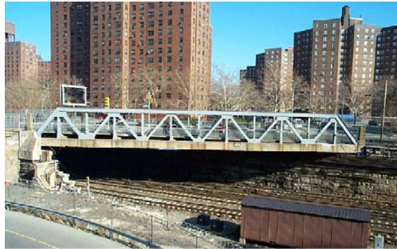
Concourse Village Avenue Bridge. (Credit: NYSDOT)
