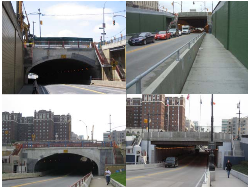
East 161 st Street Underpass East Portal in 2005 and 2008. West Portal in 2005 and 2008.
