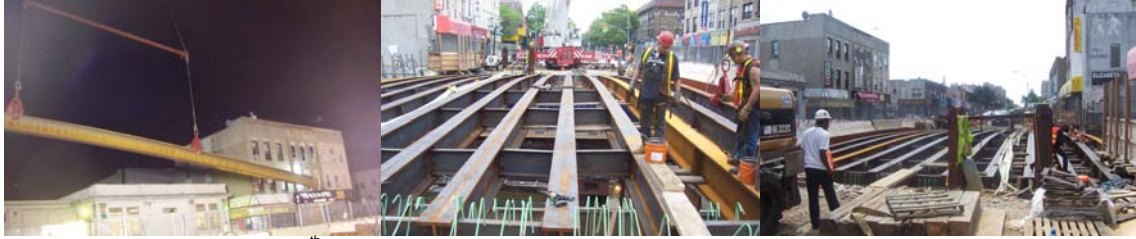
20 th Avenue Bridge Structural Steel Erection in August 2007.
