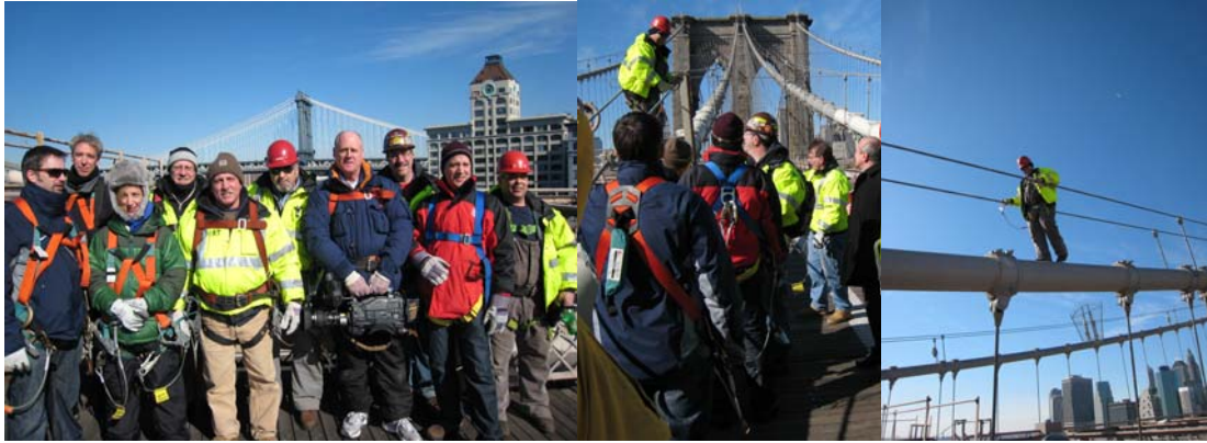
Electricians on the Brooklyn Bridge With NBC Staff in February 2008: Executive Director of Bridge Preventive Maintenance and Repair Thomas Whitehouse (4 th From Left), Electrician Robert Stackpole (5 th From Left), Supervisor Electrician Ben Cipriano (Center), Electrician Jerry Salzman (3 rd From Right), Ted Timbers (2nd From Right), and Electrician Richard Parisi (on Right). Electrician Michael Marino and Chief Bridge Officer Henry Perahia (on Right). Electrician Richard Parisi on the Cable. (Credit: Russell Holcomb)
