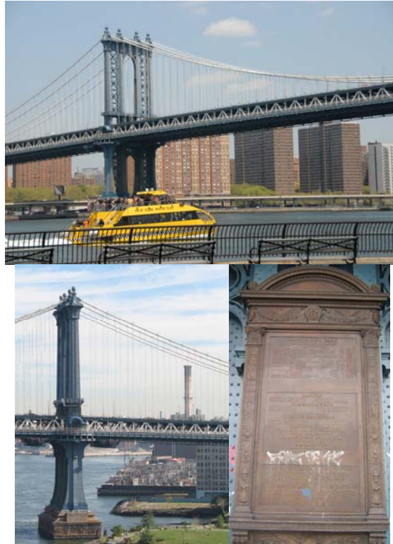
Water Taxi Approaching the Bridge. (Credit: Peter Basich) Manhattan Bridge. (Credit: Michele N. Vulcan) Construction Plaque. (Credit: Peter Basich)
