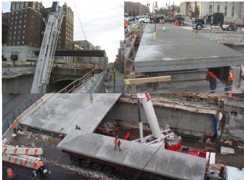
2006: Installing the Precast Panels.
