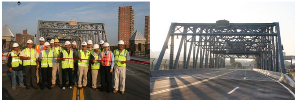
Division and Contractor Personnel at the Reopening of the 145 th Street Bridge, Including: Civil Engineer Rafeek Shaker (2 nd From Left), Chief Bridge Officer Henry Perahia (4 th From Left), Deputy Chief Engineer Jay Patel (7 th From Left), Administrative Engineer Robert Collyer (5 th From Right), Civil Engineer Hani Faouri (2 nd From Right), and Assistant Civil Engineer Khalid Mohammed (On Right). New Bridge Ready for Traffic.
