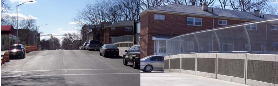
Completed 17 th Avenue Bridge and Fence.
