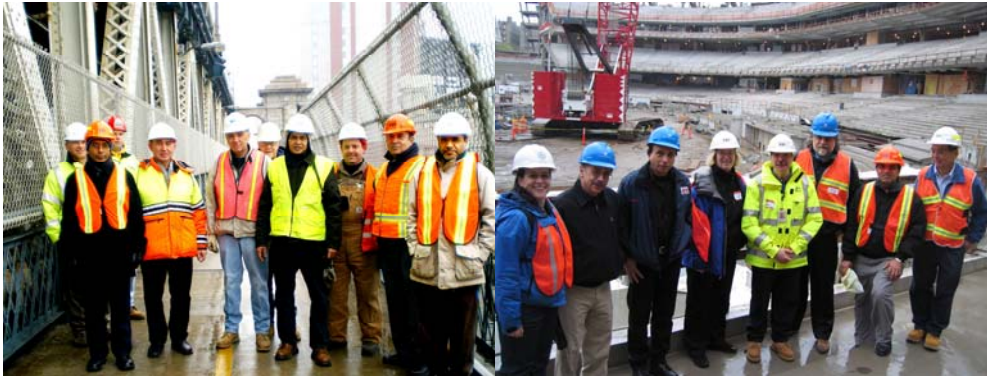
Division and Contractor Personnel at the Final Inspection of the Manhattan Bridge Anchorage in February 2008: Director of Quality Assurance Muhammad Afzal, Assistant Civil Engineer Javed Sarwar, Contractor Chief Inspector A. Perez, Assistant Engineer-in-Charge Syed Arfeen, Contractor Assistant Resident Engineer T. Mee, Contractor A. Farkas, Assistant Civil Engineer Yuliy Zak, and Civil Engineer Mohammad Hossain. Touring the Yankee Stadium Redevelopment Project in May 2008: Jennifer Tabakin, Executive Director of OCMC Joe Noto, Deputy Director of OCMC Frank Puccio, Bronx Borough Commissioner Constance Moran, Chief Bridge Officer Henry Perahia, Traffic Deputy Commissioner Michael Primeggia, Director of Engineering Support Mahabal Shah, and Civil Engineer Wen-Yang Tsay.
