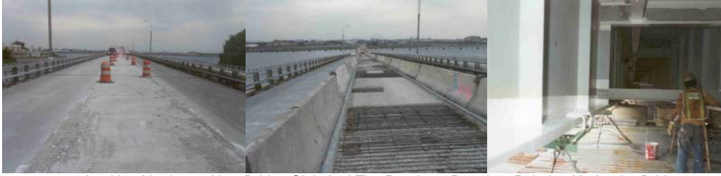
2006: Looking North at a New Bridge Slab And The Roadway Repairs. Painting Under the Bridge.
