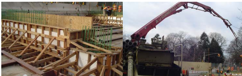
2007: West 252 nd Street Bridge Formwork and Rebar Fabrication at the Pier and West Abutment. Concrete Placement in Progress.
