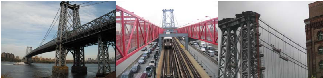
Williamsburg Bridge. Bridge Subway Structure. (Credit: Peter Basich). Contract #8 in 2004: Looking South at a Cable Band Retensioning Crew.
