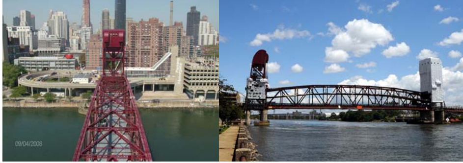
Tower Containment in August 2008. (Credit: Bernard Ente) Lift Span and West Tower in September 2008.
