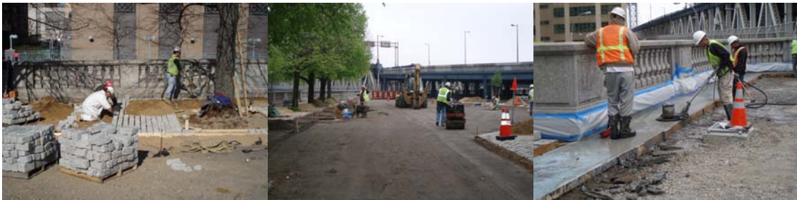
Installation of New Granite Blocks for the Plaza. Renovating the Plaza.
