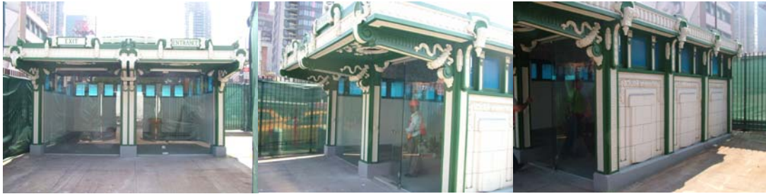
Contract #6 in 2006: Restored Queensboro Bridge Kiosk.
