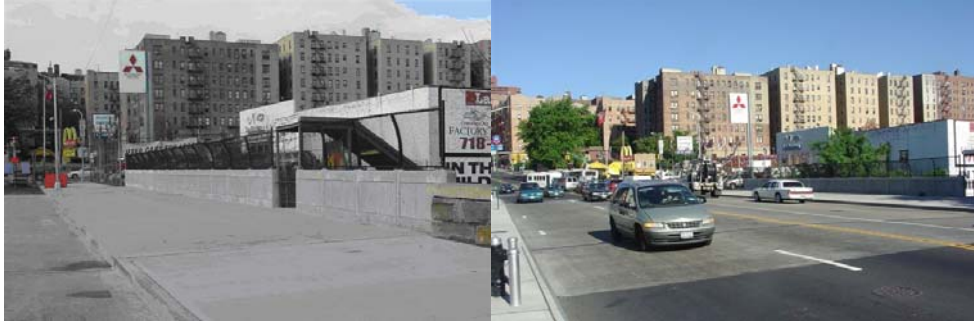
North Bridge Parapet in December 2007. Completed Bridge.
