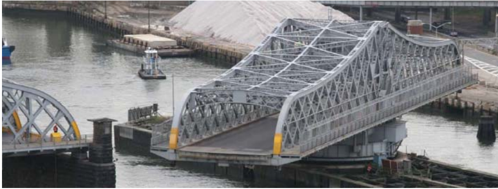
Open Willis Avenue Bridge.
