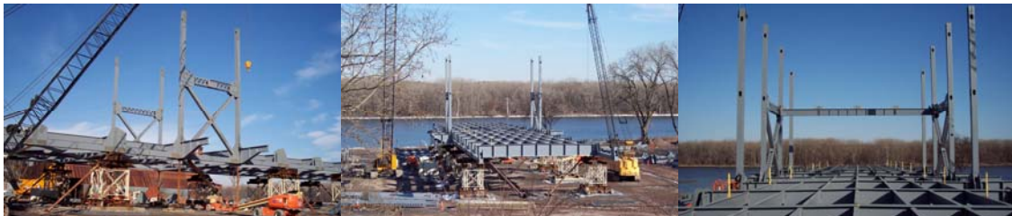
2006: Assembling the New 145 th Street Bridge Swing Span in Albany.
