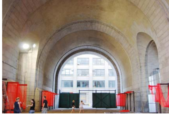
Manhattan Bridge Water Street Arch. (Credit: DUMBO NYC)
