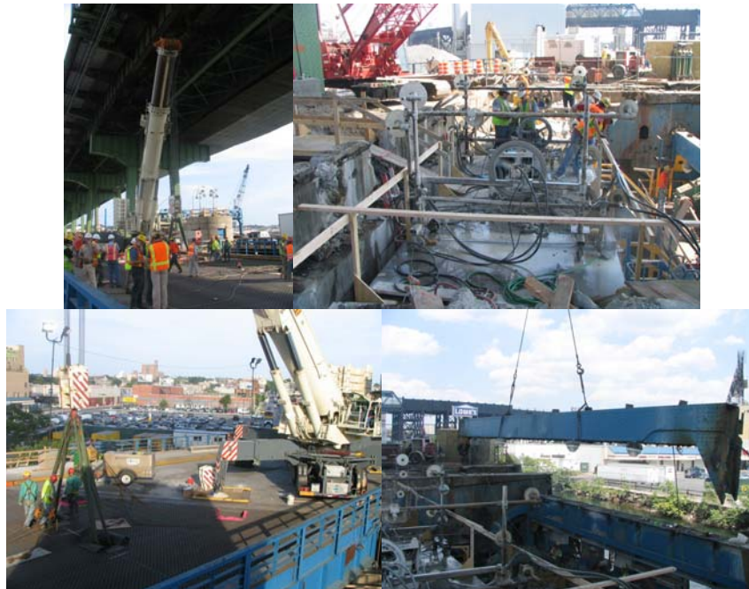
Removing the East Span in July 2007.
