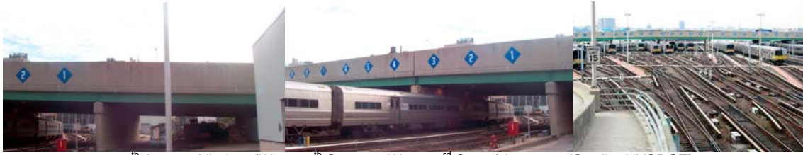
11 th Avenue Viaduct (West 30 th Street to West 33 rd Street) in 2006. (Credit: NYSDOT)
