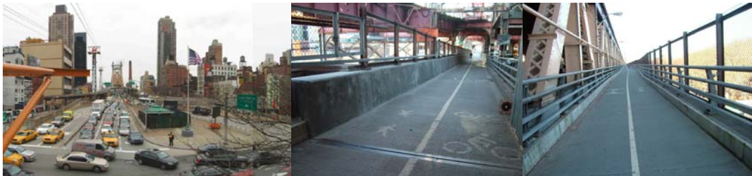
Contract #6 in 2007: Rendering of Bridge Flag Site. Protective Screening at the Queens Approach. Protective Screening and Roadway Lighting Upgrade on the North Outer Roadway. (Screening Credit: Adam Caplan)
