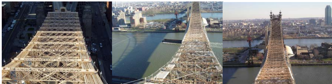
Protective Coating in 2007: Spans 1 and 2 Upper Level.
