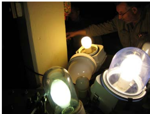
Supervisor Electrician Ben Cipriano With Both Mild and Bright Induction Light Fixtures for Testing. For Comparison Purposes, There is a Mix of Clear and Frosted Globes. (Credit: Russell Holcomb)
