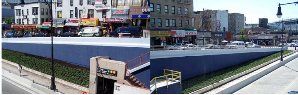
Newly Stained Retaining Walls in May 2008.
