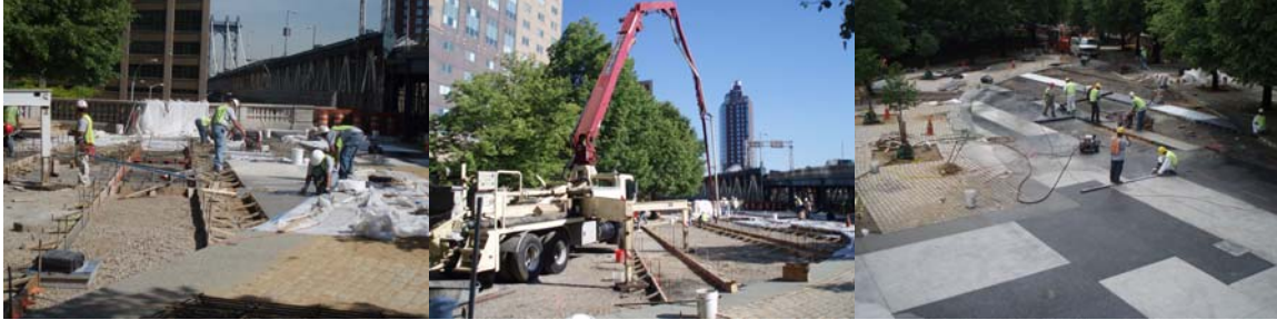
Installation of New Concrete at the Plaza.
