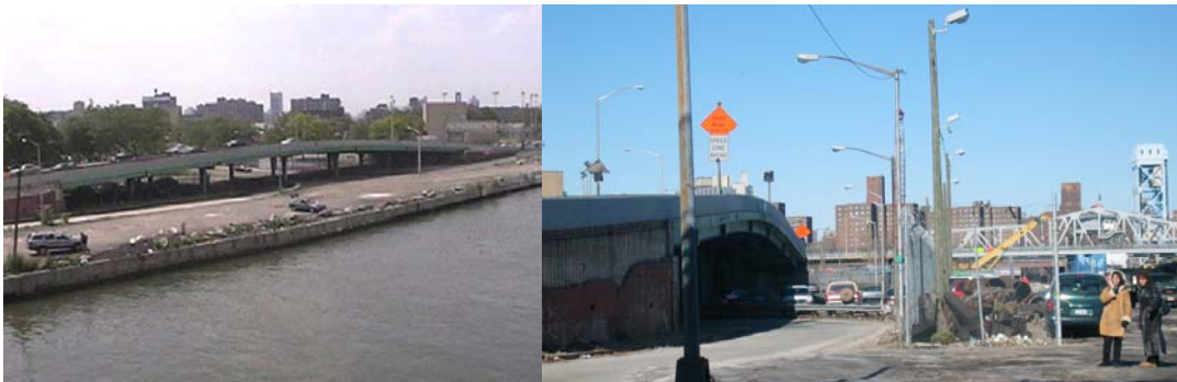
Harlem River Drive at East 127 th Street. Deputy Director of Design-Build Beatriz Duran and Director of Design-Build/Emergency Contracts Chris Sklavounakis at the Bridge.
