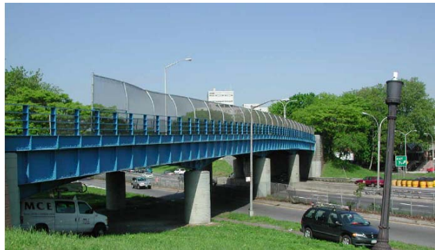
East 8 th Street Bridge in 2002. (Credit: NYSDOT)
