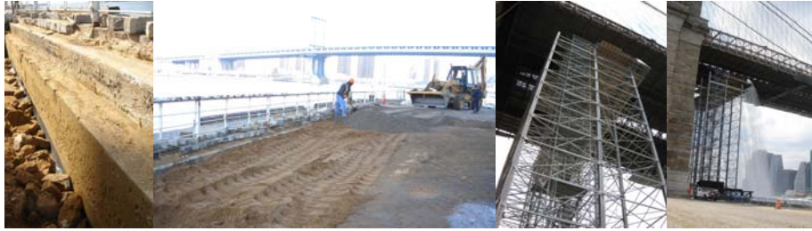
New Concrete Fill Material Under the Sidewalk in February 2008. Excavated Area Backfilled With Sand and Crushed Stone as Top Layer in March 2008. (Credit: Thomas Leung) Waterfall Structure Under Construction in May 2008. (Credit: Russell Holcomb) View of the Structure From the Brooklyn Side in June 2008. (Credit: Thomas Leung)
