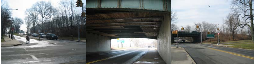
Cross Island Bridge Exit Ramp on the Northeast Side. Bridge Underdeck. South View of the Bridge. (Credit: Tamara Berlyavsky)
