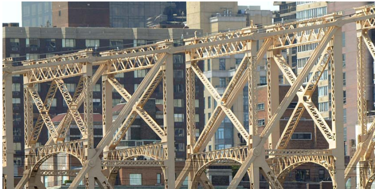
Bridge Detail in 2008. (Credit: Bernard Ente)
