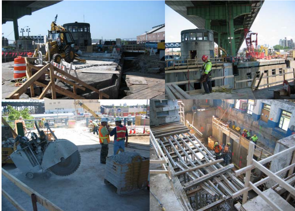
2007: Hamilton Avenue Bridge Construction.
