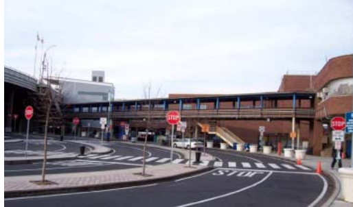
The Ferry Terminal Pedestrian Bridge.
