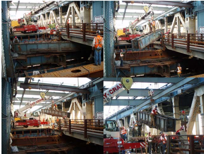
Contract #11 in 2006: Sequence of Removing Existing Floorbeam at Brooklyn Tower.
