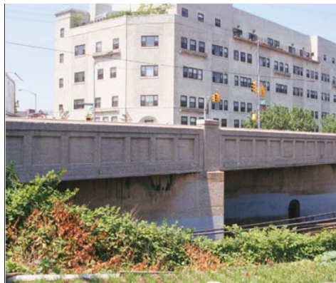
Woodside Avenue Bridge. (Credit: NYSDOT)
