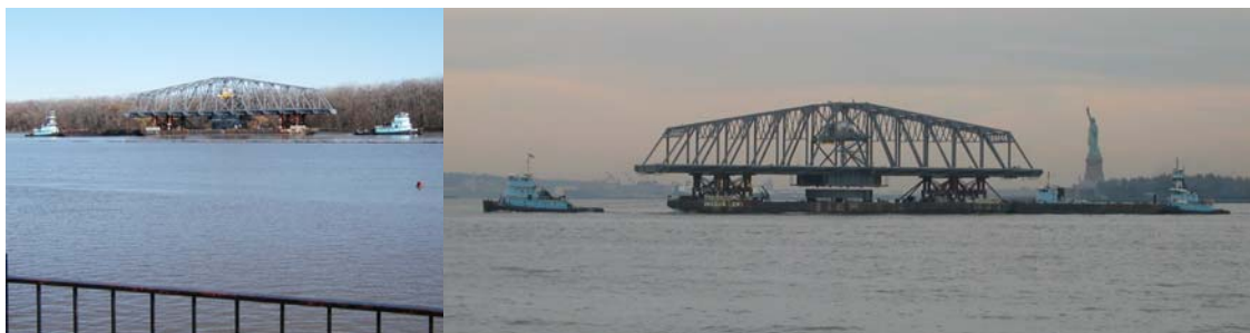
2006: New 145 th Street Bridge Swing Span Leaving Albany. Passing the Statue of Liberty.
