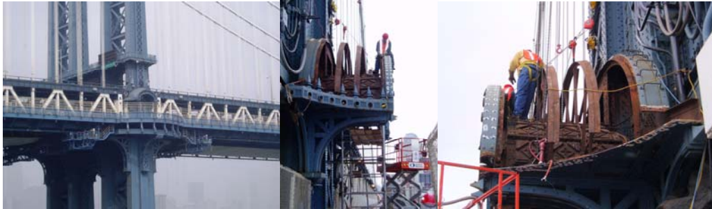
Contract #11 in 2005: The Brooklyn Tower Canopy. Removing the Canopy.
