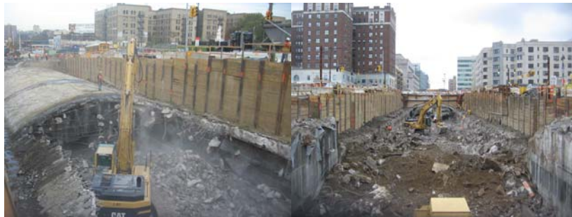
2006: Demolition of the Bridge. Removing Debris From the Bridge.
