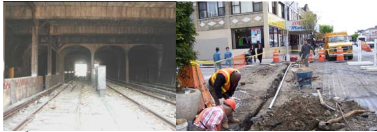
18 th Avenue Bridge in 2003. (Credit: NYSDOT) Bridge Nearing Completion.
