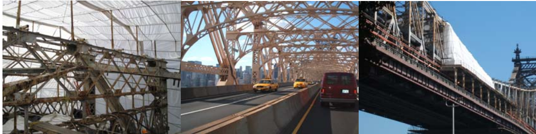
Protective Coating in 2006: Inside the Containment Rigging at Span #1. Finish Coat on the Trusses at Span #5 on the Upper Roadway. Class 1A Containment Installed on the Trusses at Span #2, And the Working Platform Above the South Outer Roadway.
