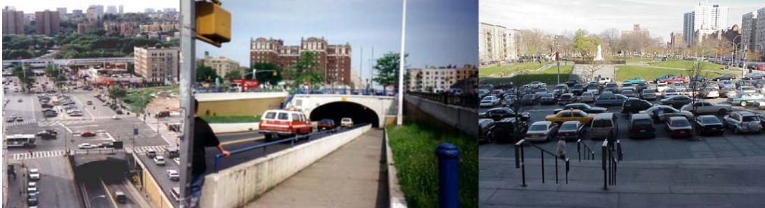
Before Construction: The Bridge over East 161 st Street. View of West Portal. Lou Gehrig Plaza.
