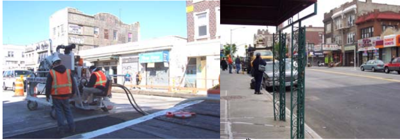
Finishing the Road. Completed 18 th Avenue Bridge.
