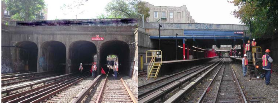
Crooke & Newkirk Avenue Bridges. (Credit: NYSDOT)
