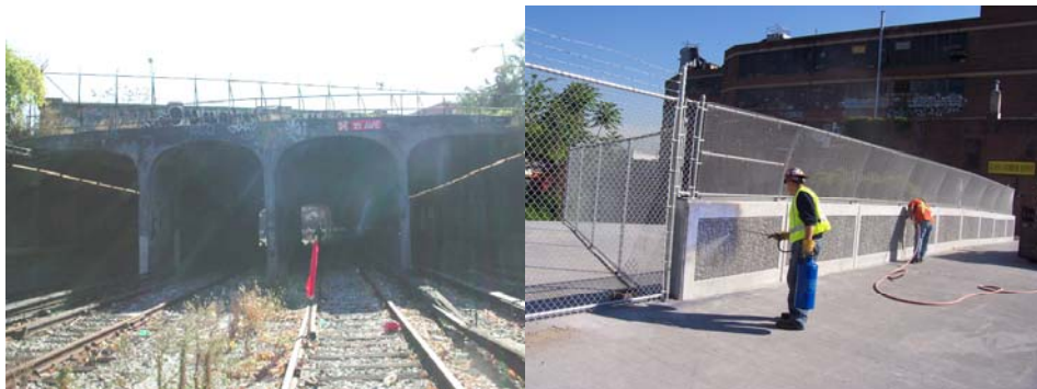
15 th Avenue Bridge in 2002. (Credit: NYSDOT). Final Touches on Completed Bridge.
