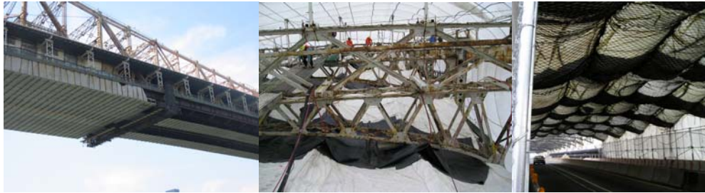
Platform Installed for Painting of the Queensboro Bridge. (Credit: Vadim Sokolovsky) Working Inside the Containment. Protected Roadway.
