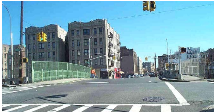
East 183 rd Street Bridge in 2002. (Credit: NYSDOT)
