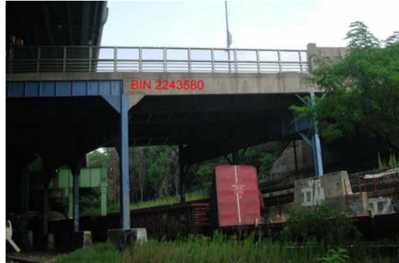
5 th Avenue Bridge. (Credit: NYSDOT)
