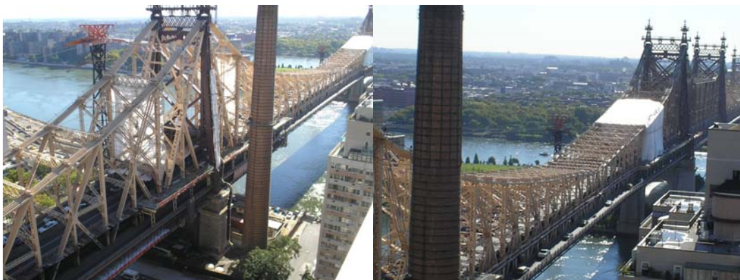
Bridge Painting in Progress: July 2007.
