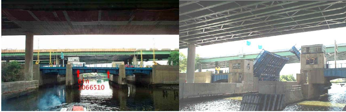
Unionport Bridge in 2002. (Credit: NYSDOT)
