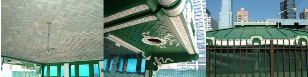
Contract #6 in 2006: Restored Queensboro Kiosk Ceiling and Other Elements.
