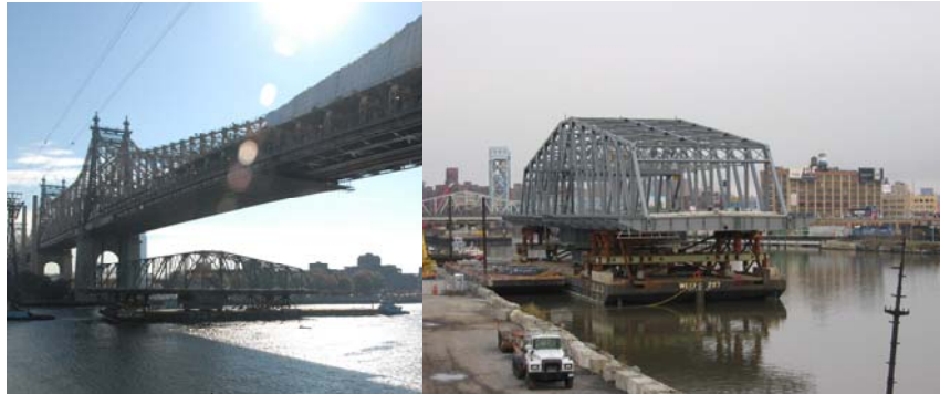
2006: New 145 th Street Bridge Swing Span Passing Under the Queensboro Bridge. (Credit: Peter Basich) Third Avenue Bridge Site. (Site Credit: Russell Holcomb)
