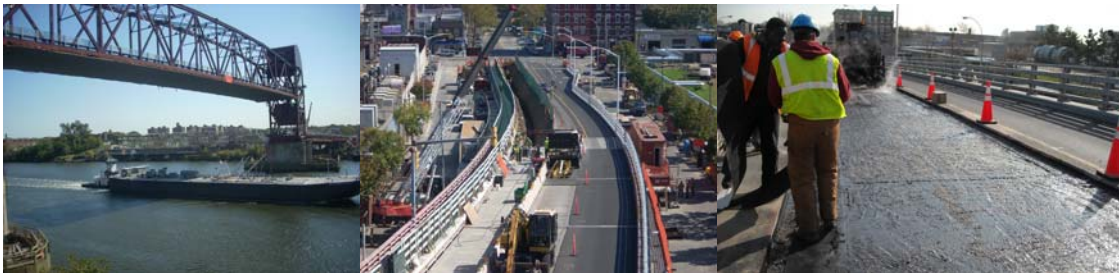
Open Lift Span During United Nations General Assembly Week in September 2008. Stage II Roadway Construction of the Queens Approach in October 2008. Asphalt Placement on the Queens Approach in November 2008.
