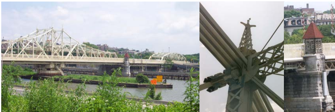
2004: East View of Macombs Dam Bridge Swing Span and Camelback Truss. (Credit: Peter Basich) Architectural Detail of the Bridge. (Credit: Michele N. Vulcan) Close-up of a Gate House. (Credit: Peter Basich)
