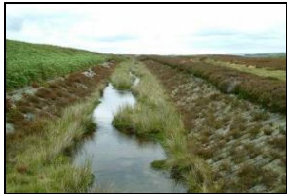
Northern inlet channel.
