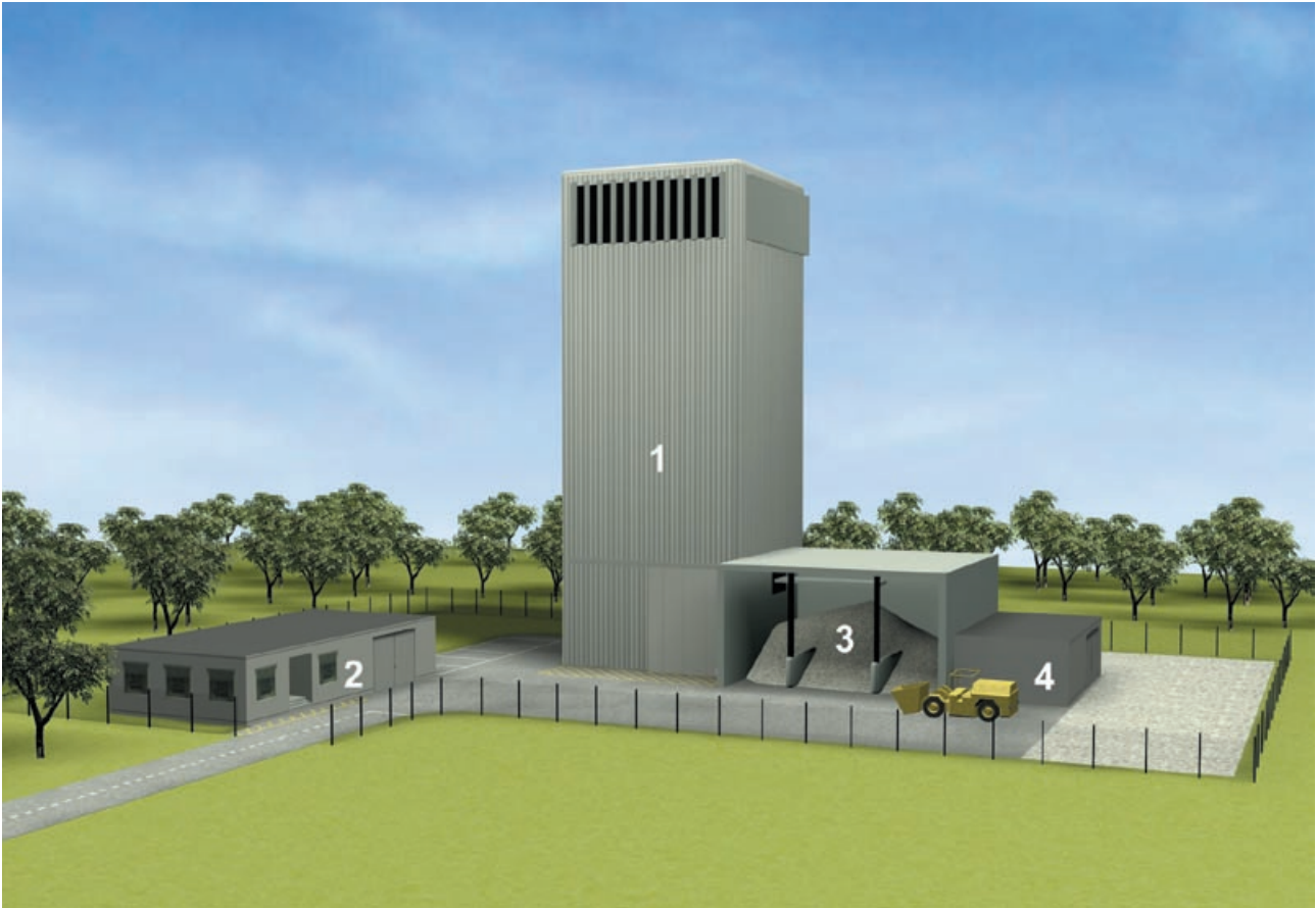
Figure 10 Model view of the area at the top of the shaft showing the shaft head frame with exhaust air vents (1) and auxiliary buildings (2 to 4).
