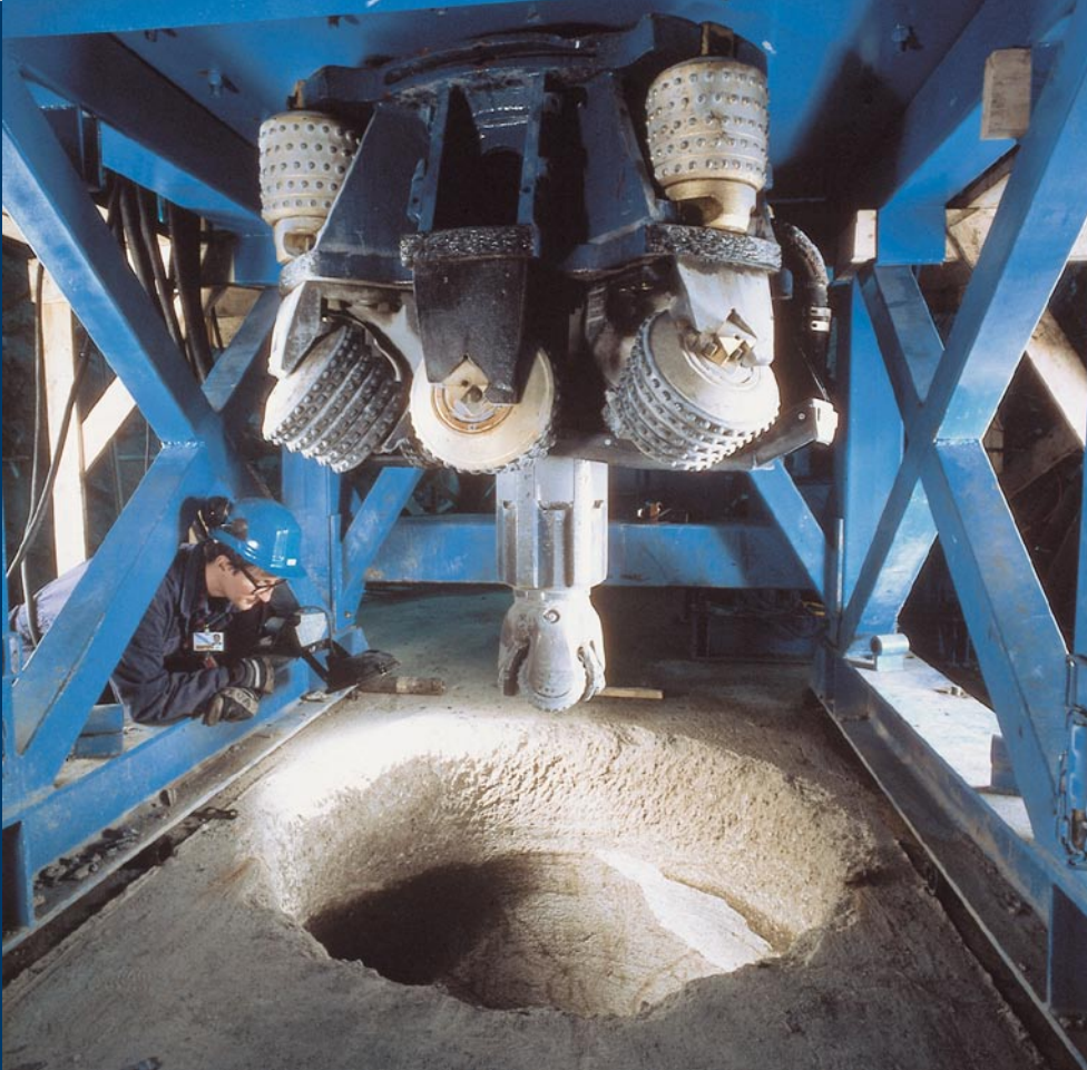
Drilling of deposition holes.
