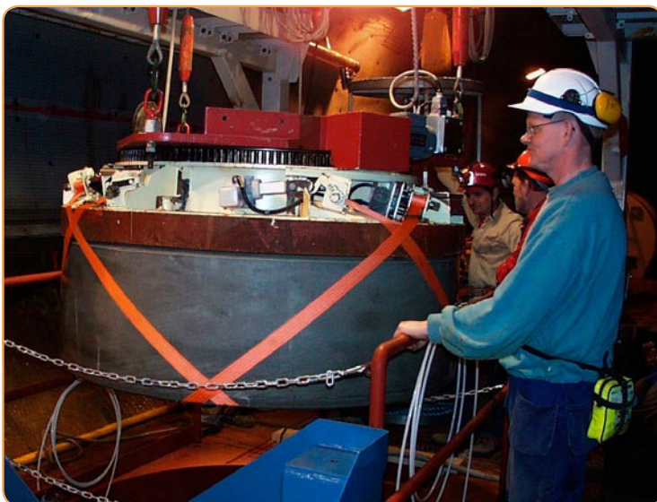
The buffer is made of bentonite clay.
