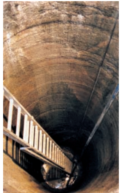
The deposition holes are eight metres deep and just under two metres in diameter.
