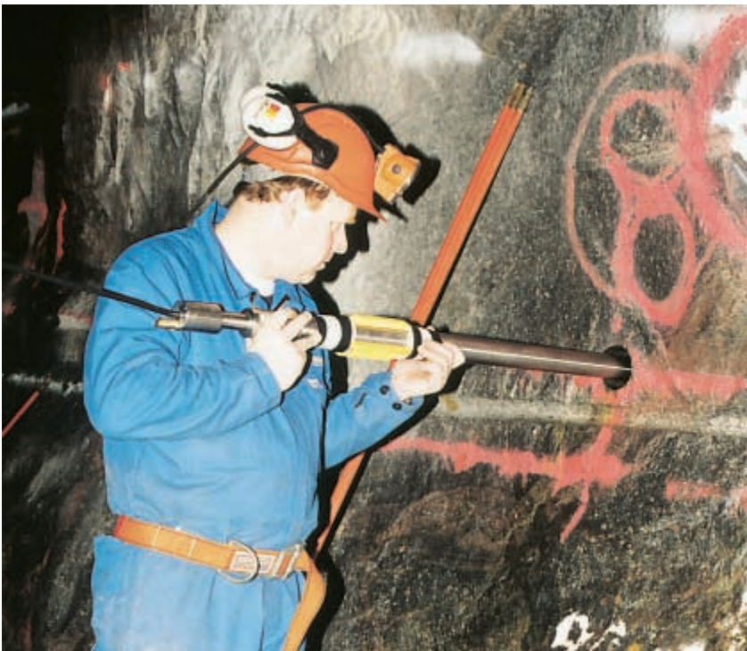
The rock must be thoroughly investigated prior to construction.
