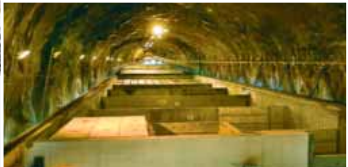
⑥ A rock vault fitted with shafts. Intermediate-level waste in drums or moulds is deposited in the shafts. When a shaft is full a concrete lid is placed on top of it.
