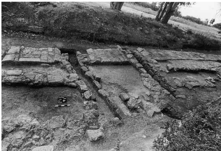
5. The northern part of the 'Lower Aqueduct', upon which a road was built, looking east.
