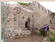
7. Early city wall incorporated in Ottoman-period wall, looking southwest.
