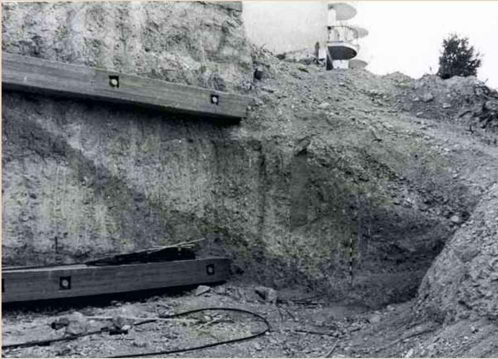
2. South side of trench, looking southeast.
