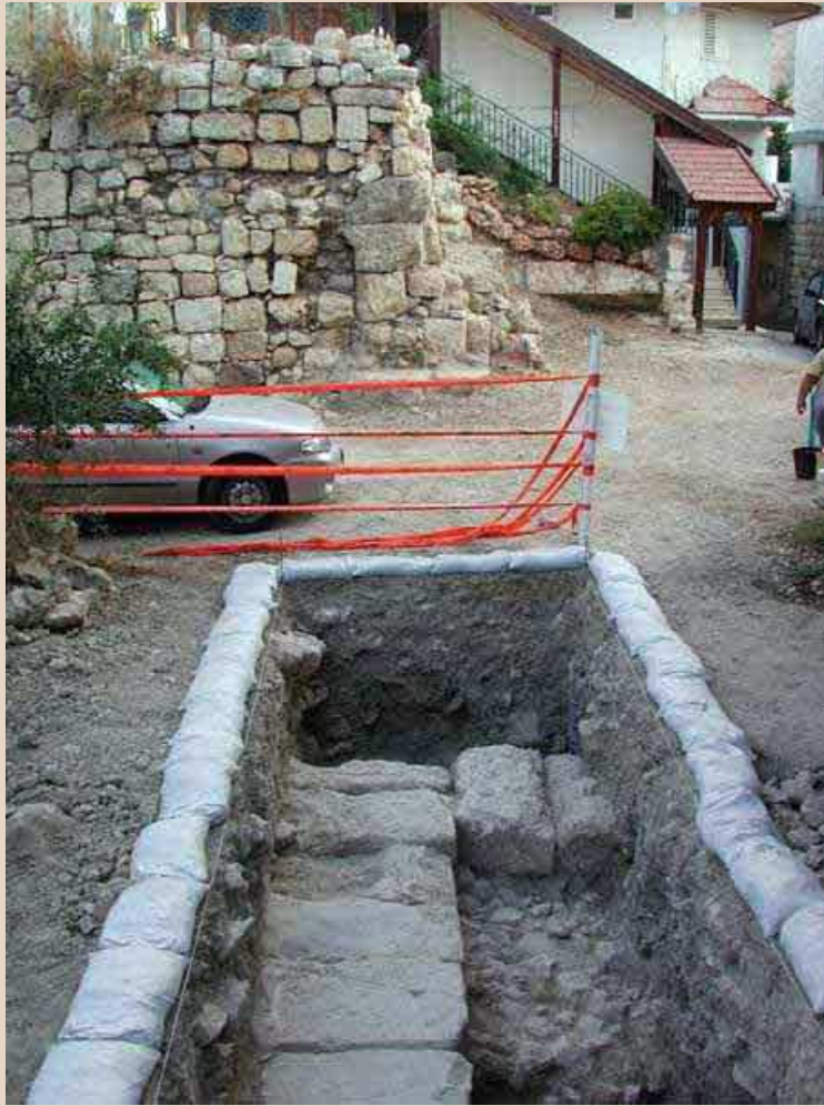
7. Wall 14 and its continuation in the Crusader building, looking north.
