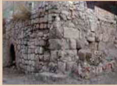
2. Remains of the Crusader-period building, looking northwest.
