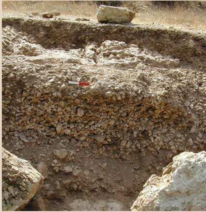
1. Section of the soil fills between the terrace wall and the bedrock outcrop, looking
