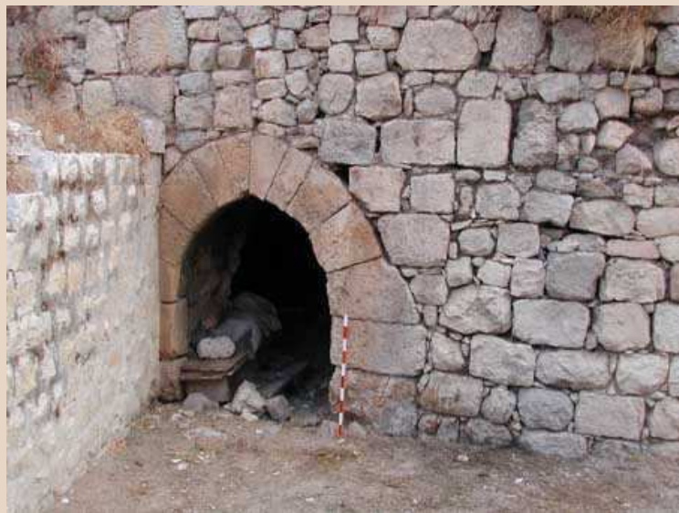
10. The Crusader building, an opening with a pointed vault, looking north.
