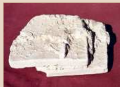
1. Tiles with light gray bonding material.
