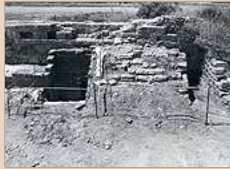
3. Area A, Arches 113 and 115 and their thickenings in Aqueduct D, looking north.
