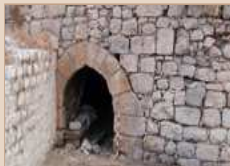
10. The Crusader building, an opening with a pointed vault, looking north.
