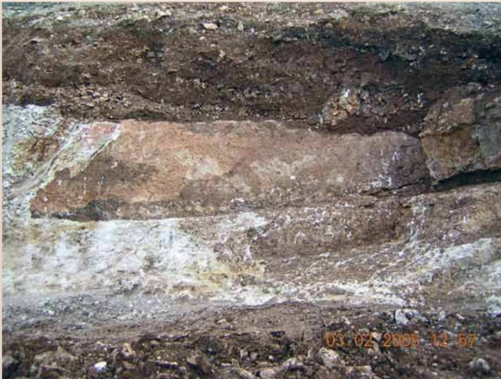
2. Rock-cutting 1, looking west.
