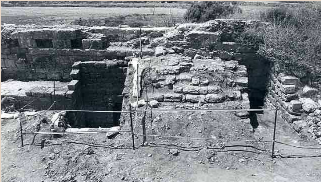
3. Area A, Arches 113 and 115 and their thickenings in Aqueduct D, looking north.
