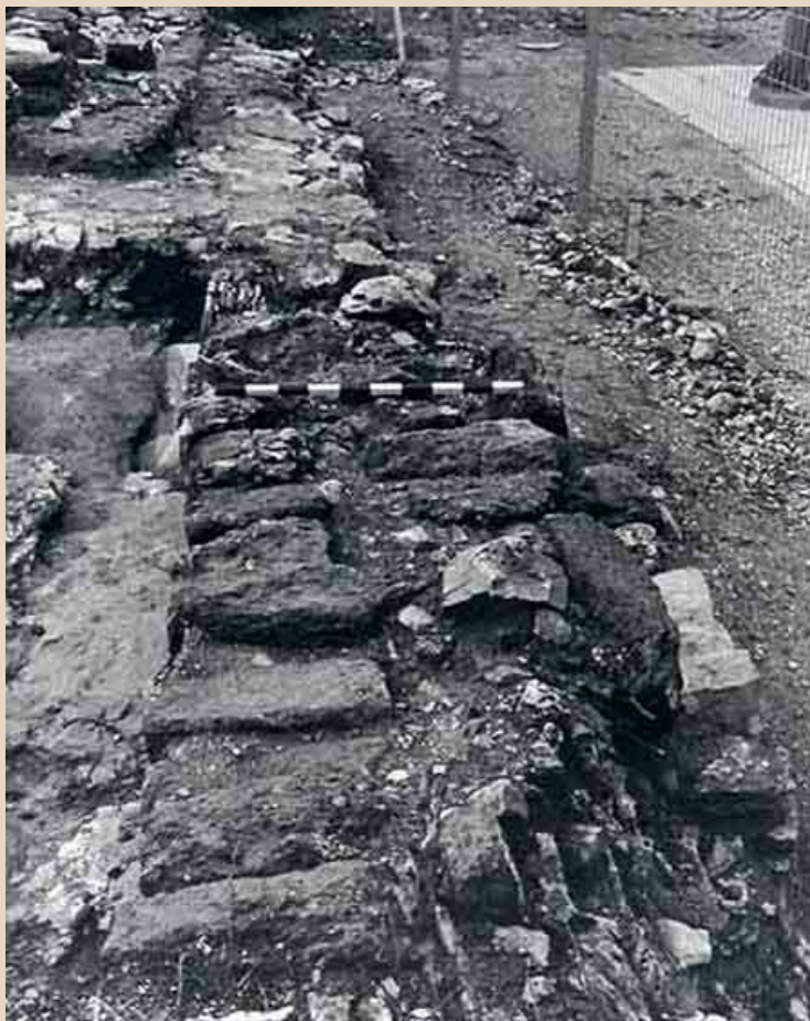
1. Wall remains of the building, looking west.
