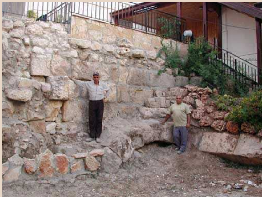
8. Remains of a water reservoir, looking west.
