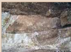
2. Rock-cutting 1, looking west.
