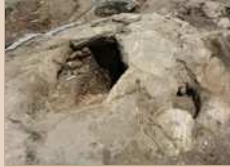
2. The openings, looking southeast.
