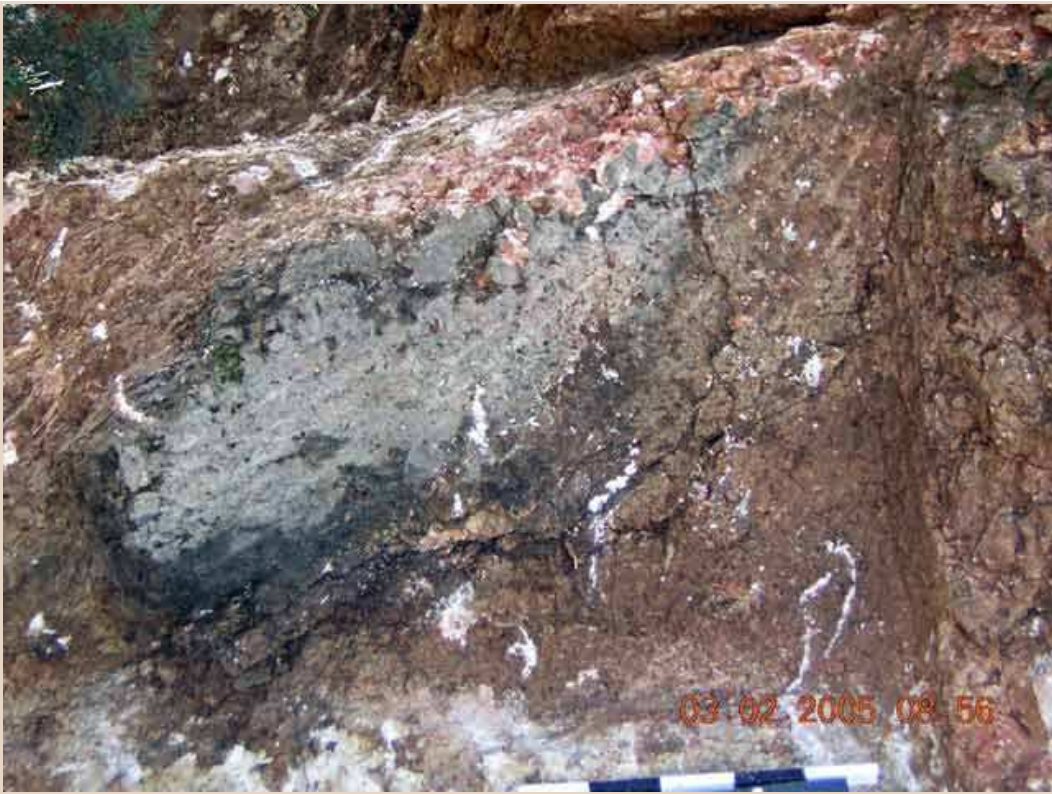
6. Rock-cutting 3, looking west.
