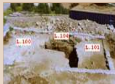
1. General view of excavation.
