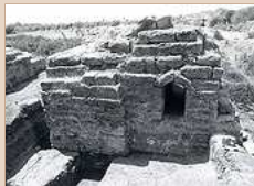
5. The narrow passage between Piers 5 and 6, looking south.
