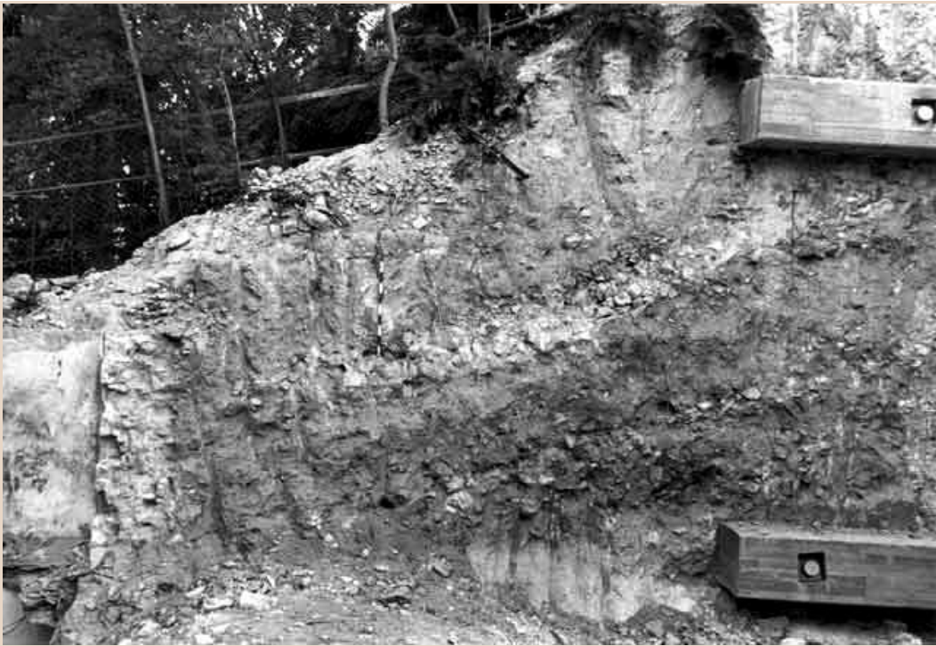
4. North wall of trench, looking north.
