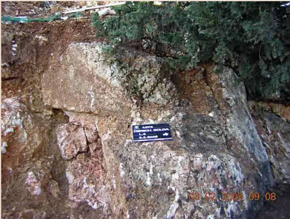
4. Rock-cutting 2, looking west.
