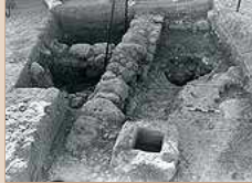
2. The excavation, looking east.
