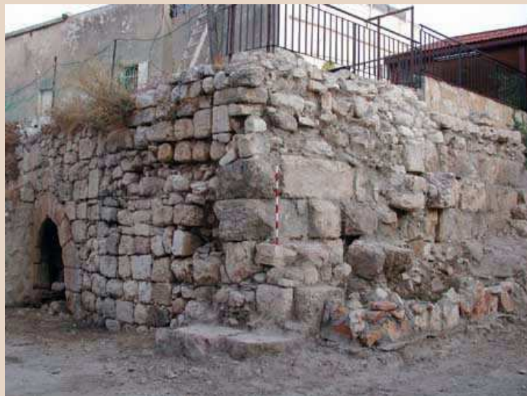
2. Remains of the Crusader-period building, looking northwest.
