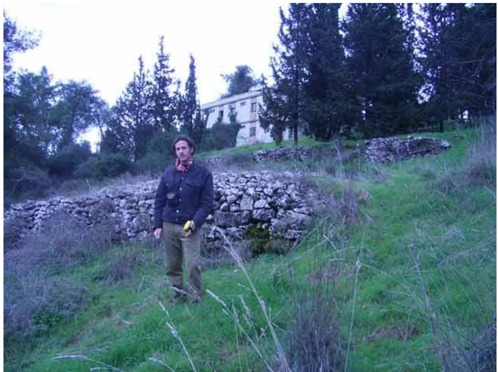
3. Farming terrace retaining walls, looking south.
