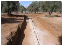
7. Southwestern part of aqueduct, looking southwest.
