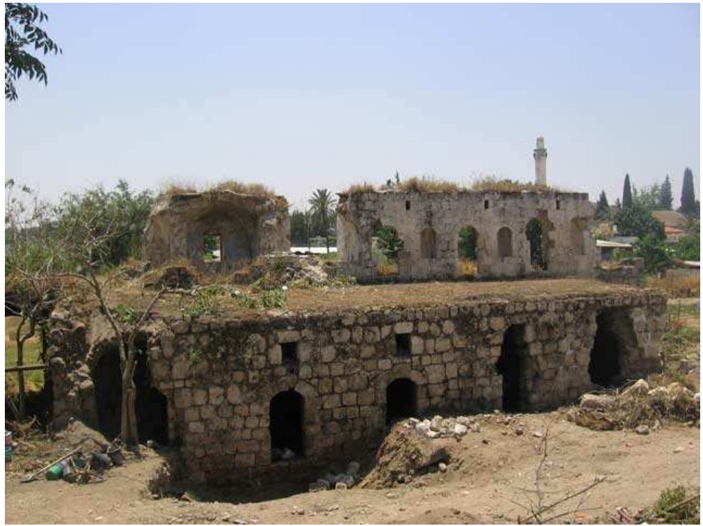
4. Southern wing after cleaning, looking southwest.
