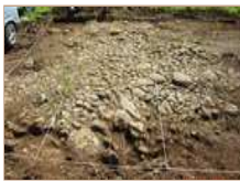
8. The road prior to excavation.
