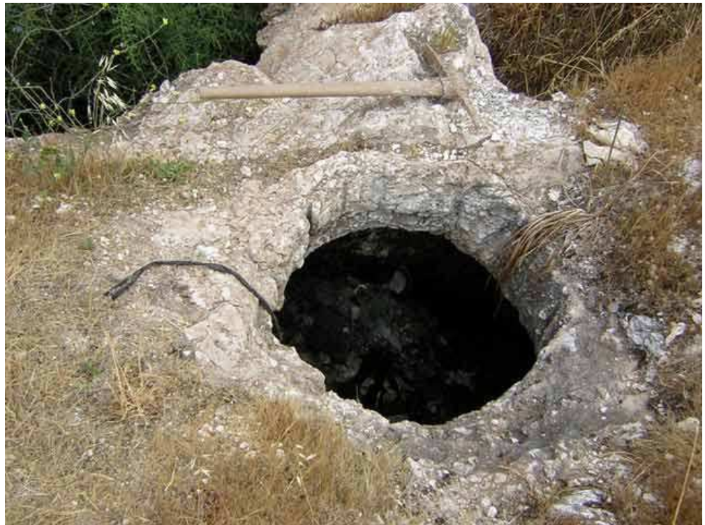
8. Water cistern, looking northwest.
