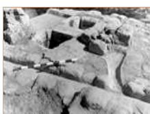
4. The vaulted roof, looking northeast.
