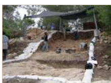
4. General view, looking west.
