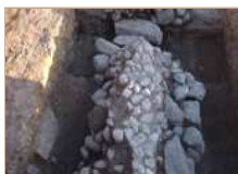
2. General view of aqueduct remains, looking north.
