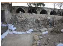
3. Modern debris inside courtyard.
