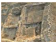
2. The southern house, looking east.
