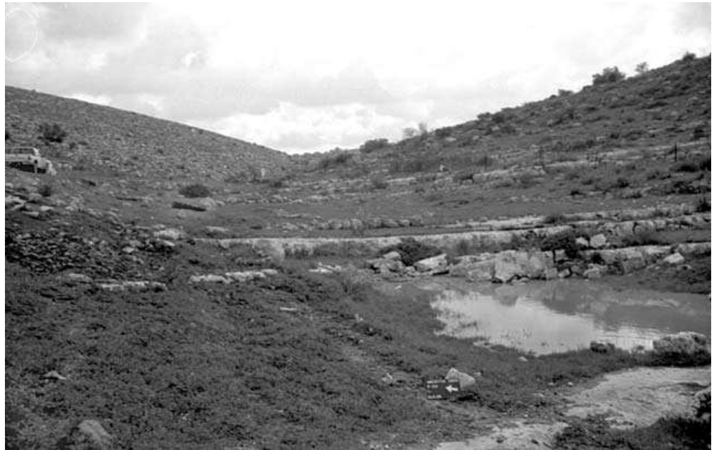
3. The system of dams in the wadi channel, south of Road 30.
