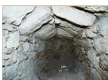
3. Area T, the underground gabled unit (L434), looking east.
