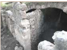
2. The reservoir, looking east.
