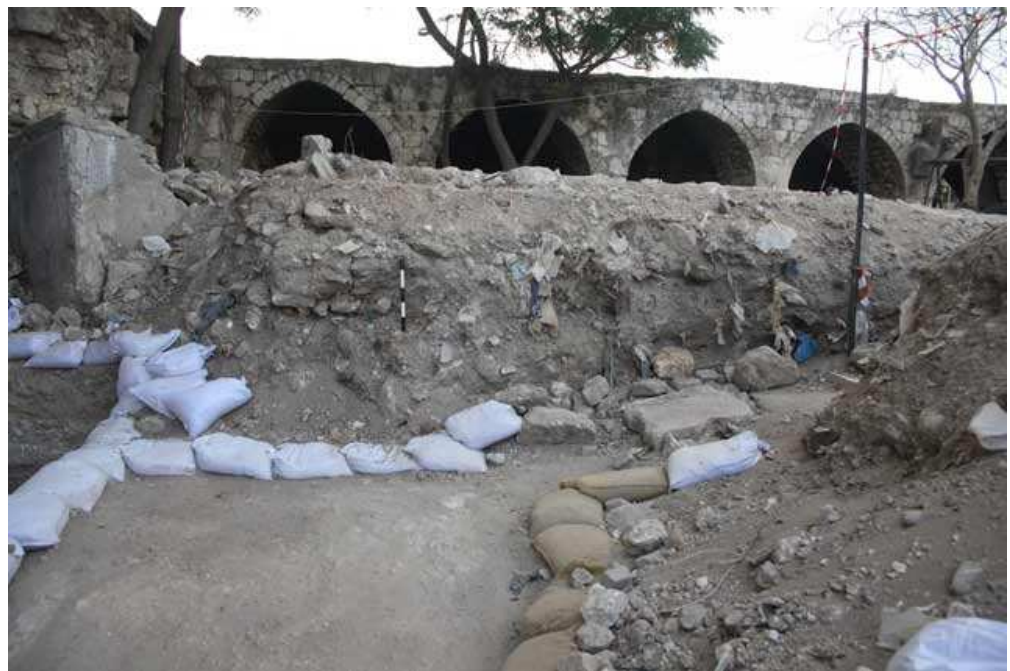
3. Modern debris inside courtyard.
