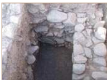
3. Walls from the Iron Age I (right) and the Middle Bronze Age II, looking north.
