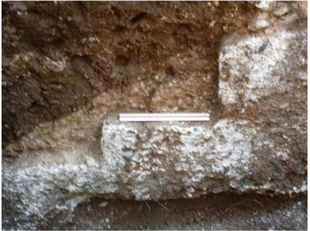
4. The staircase (L2), looking south.
