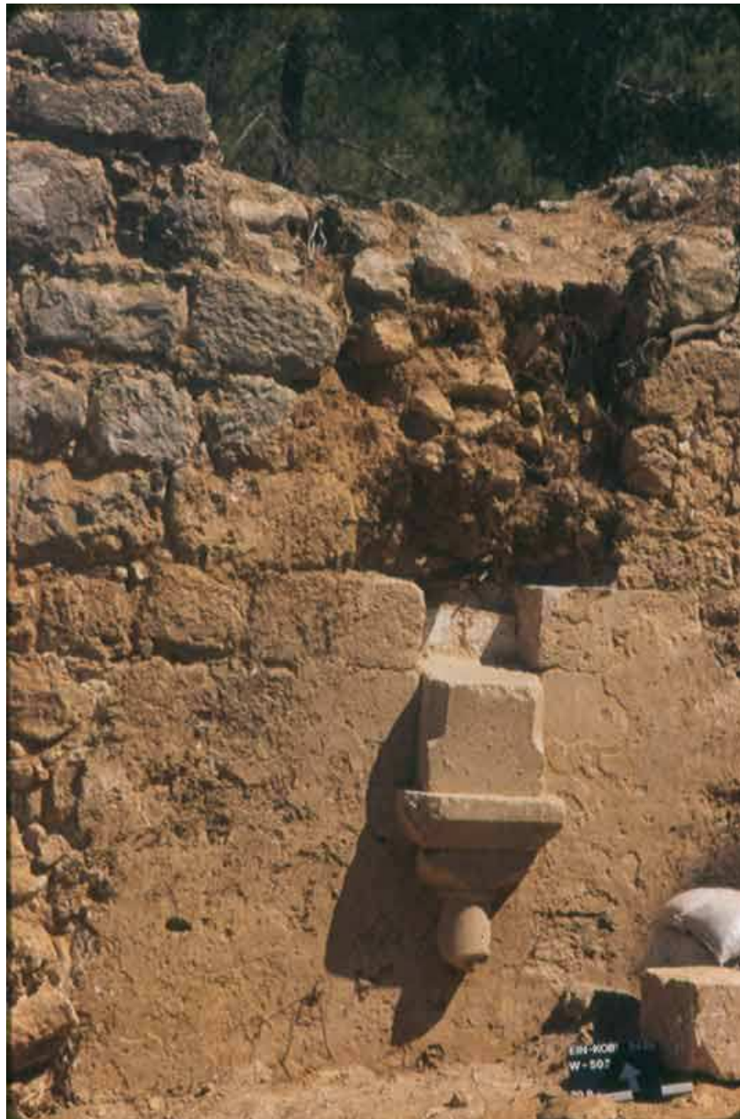
5. An elbow column in the northern wall of the church, looking north.
