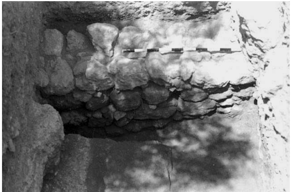
2. Wall 248, looking north
