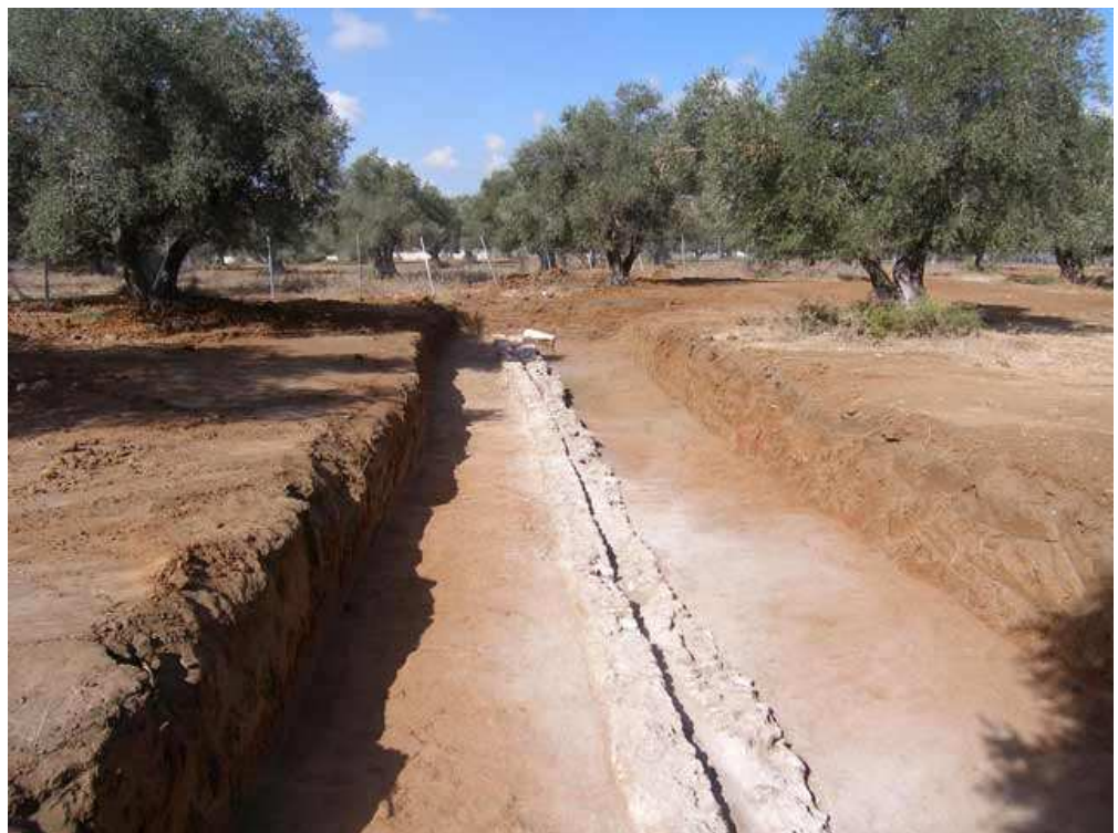
7. Southwestern part of aqueduct, looking southwest.
