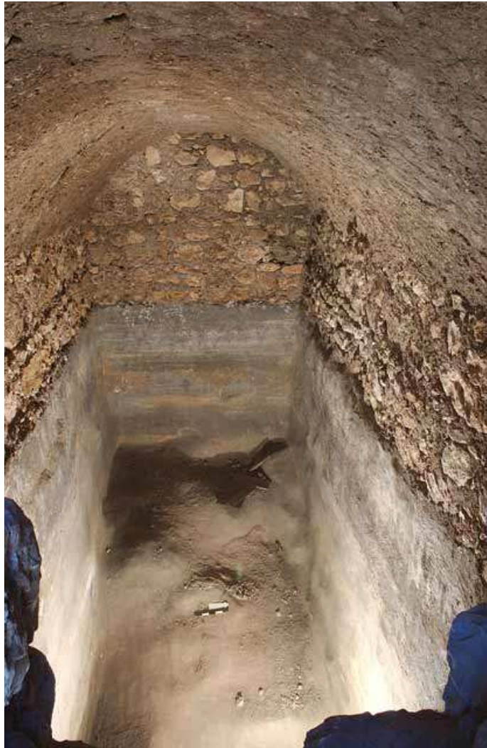
4. The water cistern, looking west.
