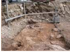
1. The excavation, looking east.
