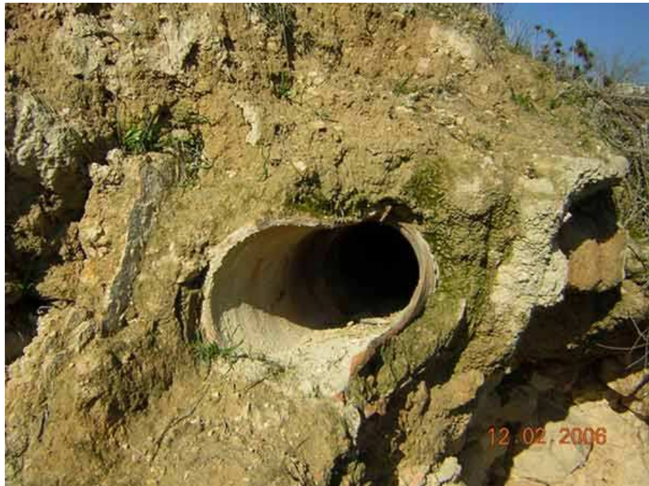
3. The later ceramic pipe inside the aqueduct (Site 14).
