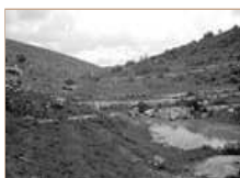
3. The system of dams in the wadi channel, south of Road 30.
