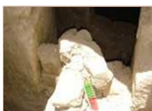
4. E1, blocked stairway.
