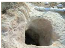
4. The opening to the cistern, looking east.
