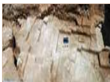
4. Courtyard Quarries 1011, 1012, looking north.
