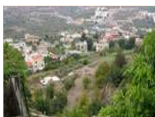
2. The excavation area, looking west.
