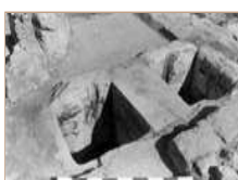
3. The openings in the vaulted roof, looking northeast.
