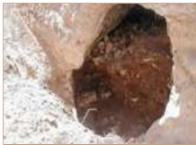
2. Water cistern, looking east.
