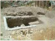
1. General view of the excavation, looking west.
