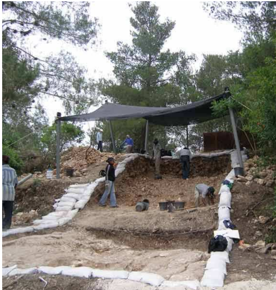
4. General view, looking west.
