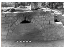
5. The blocked arch in W8, looking southeast.
