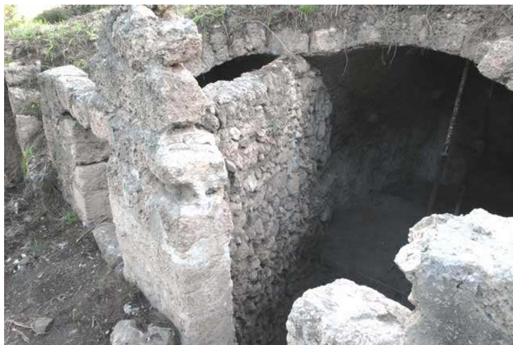
2. The reservoir, looking east.
