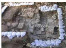
2. General view of the excavation, looking west.
