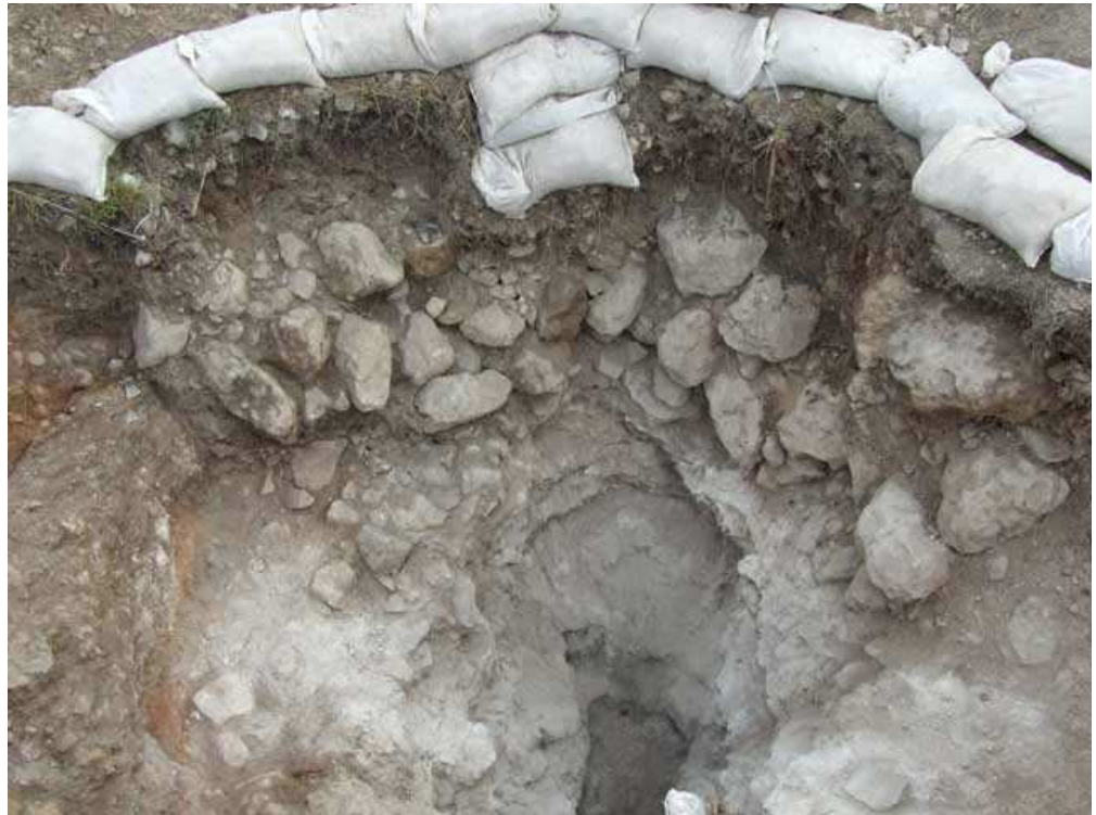
9. Area 6, the lining of limestone, lime and ashes in kiln pit, looking east.
