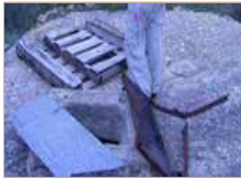
2. Opening of the water cistern (Site 12), looking north.
