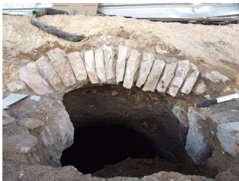
3. The arched opening and the square top of the cistern, looking north.
