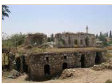
4. Southern wing after cleaning, looking southwest.
