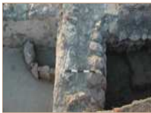
4. Wall 1, looking east.
