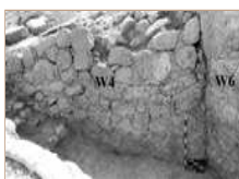
4. Wall 4 abutting Wall 6, looking east.
