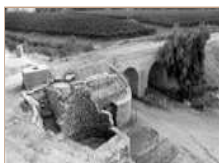
2. General view, looking northwest.
