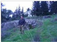
3. Farming terrace retaining walls, looking south.
