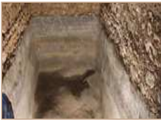
4. The water cistern, looking west.
