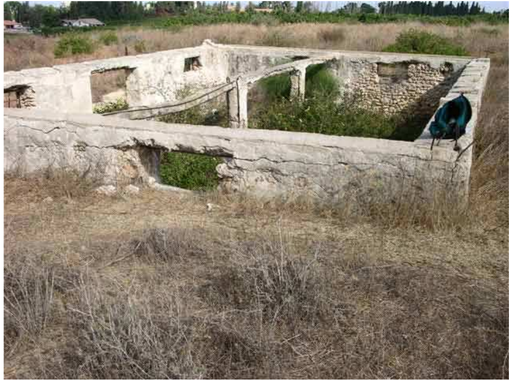
3. Modern building, looking north.
