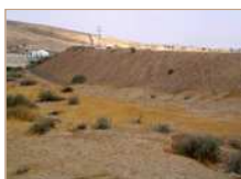
3. The railroad embankment, looking southeast.
