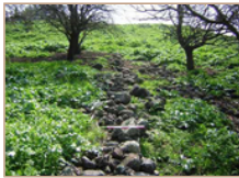
7. Terrace Wall 4, looking north.
