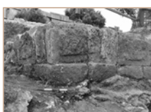
3. Area A, the early phase, corner of building with drafted margins, looking northeast.
