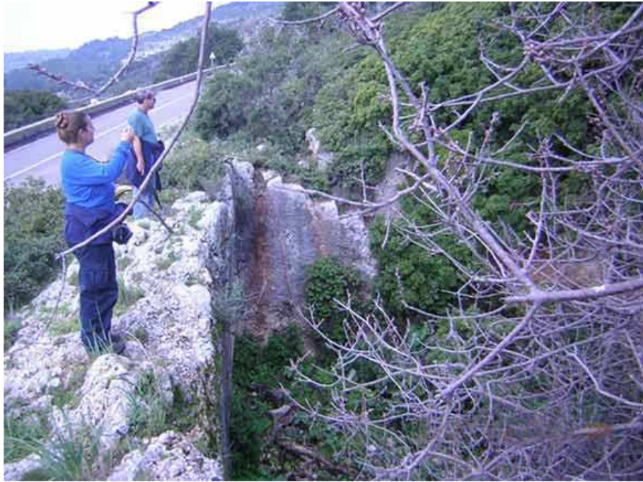
2. Site 17, rock-hewn water reservoir, looking west.
