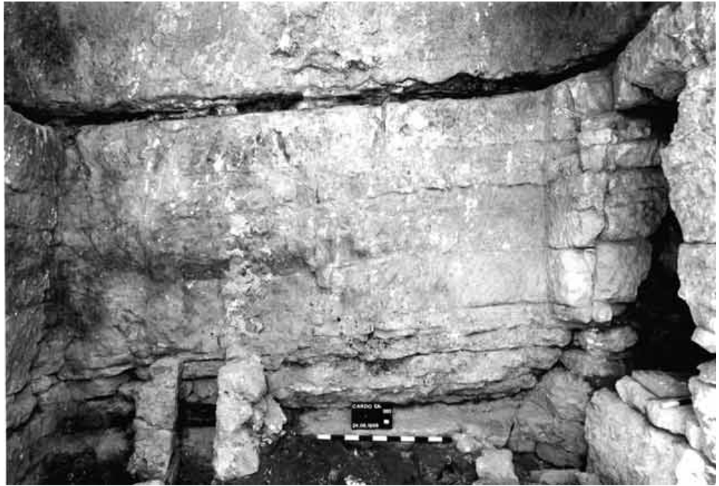
3. The upper and middle stories, looking west.
