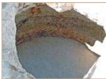
2. Cistern, looking north.
