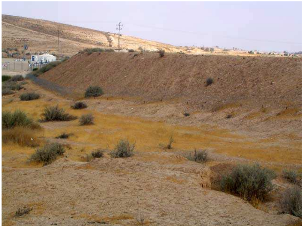
3. The railroad embankment, looking southeast.
