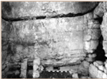
3. The upper and middle stories, looking west.
