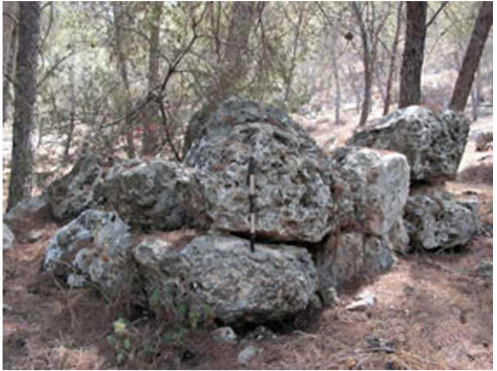
3. Built corner of field tower, looking west.
