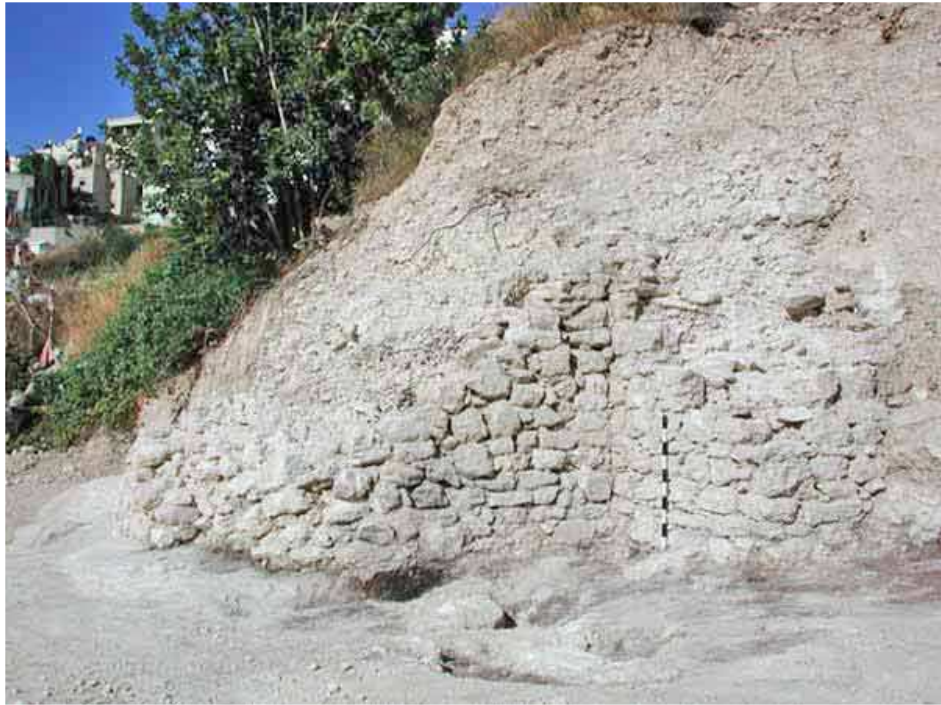
9. Area E, field tower, looking south.
