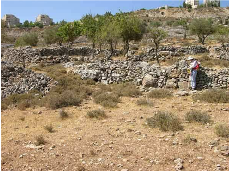
4. Site 6, retaining wall of farming terrace, built on ancient wall, looking north.
