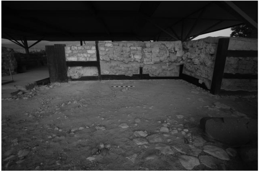
3. Area A-6, the restoration of the Ceremonial Palace façade, looking west.
