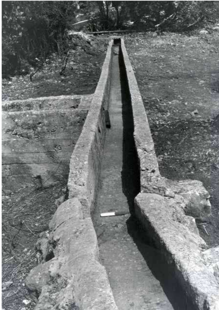
3. The concrete Mandatory aqueduct above the ancient aqueduct's wall, looking north.
