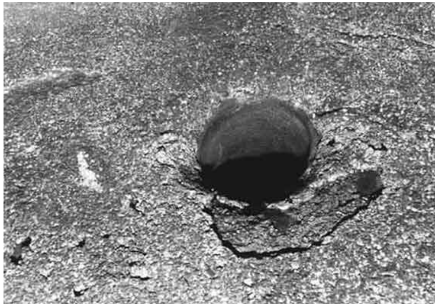
2. A ceramic pipe opening, view from inside the cistern.
