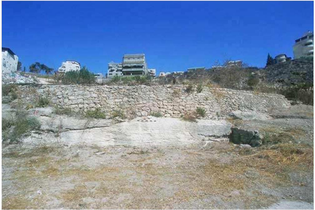
8. Wall 116, looking west.
