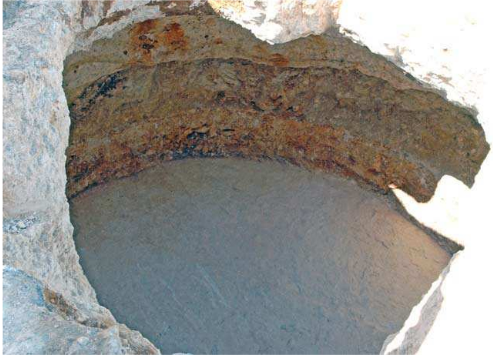
2. Cistern, looking north.
