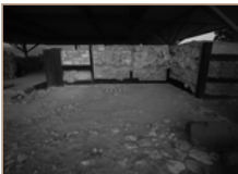
3. Area A-6, the restoration of the Ceremonial Palace façade, looking west.
