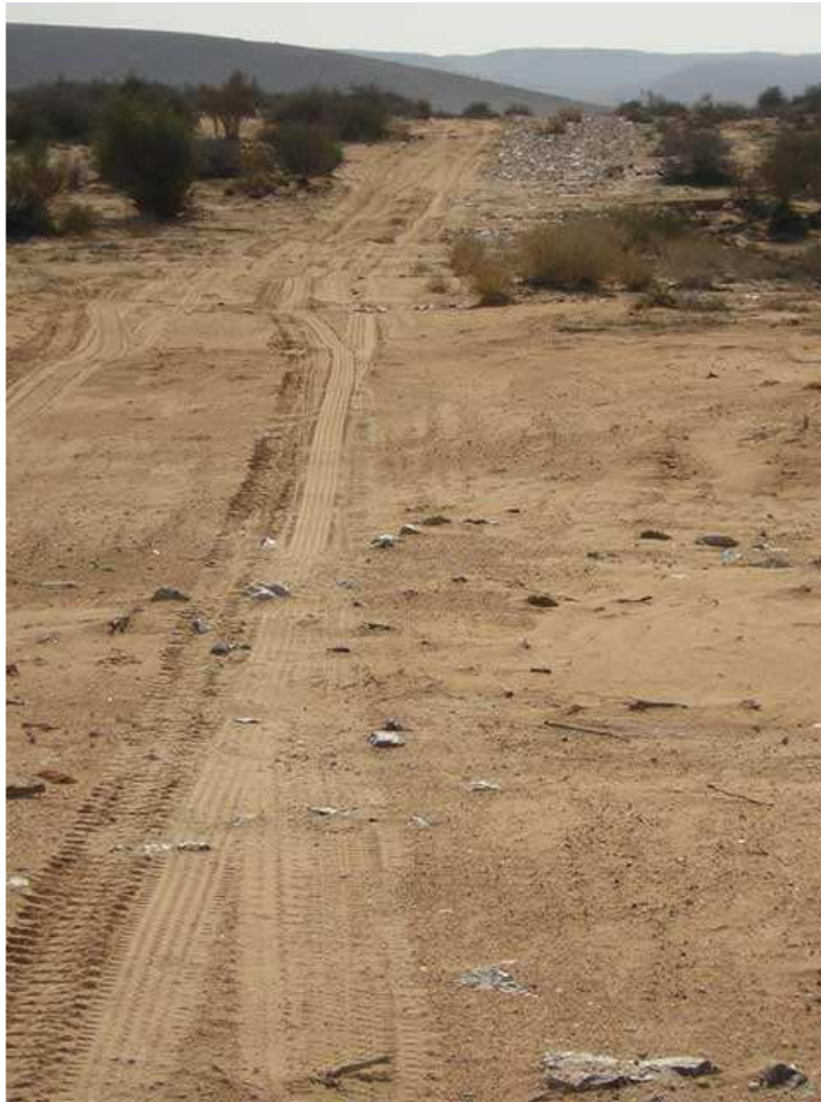
7. Southern section of road, looking south.
