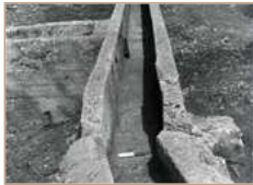
3. The concrete Mandatory aqueduct above the ancient aqueduct's wall, looking north.
