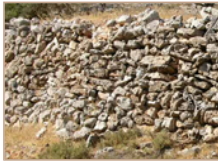
2. Site 1, retaining wall of farming terrace, looking southwest.
