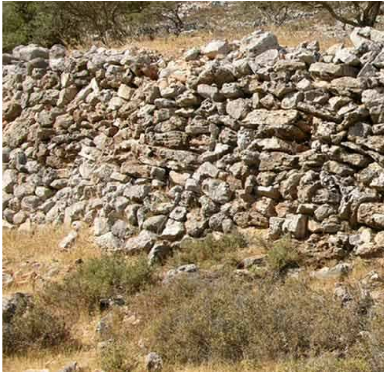
2. Site 1, retaining wall of farming terrace, looking southwest.
