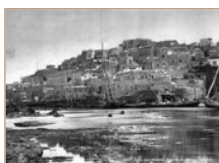
8. Yafo and the Ottoman seawall in center of harbor, looking east (photographed by Felix Bonfils, 1875).
