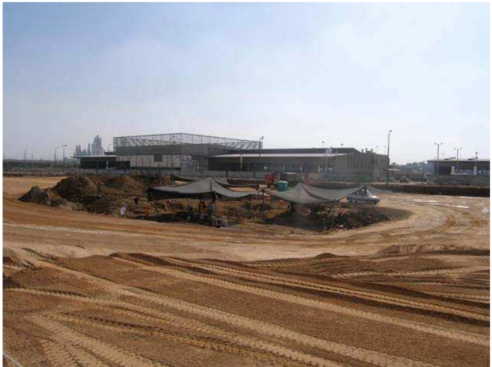
1. The excavation, looking southwest; in background, the Ta'avura factory under construction.
