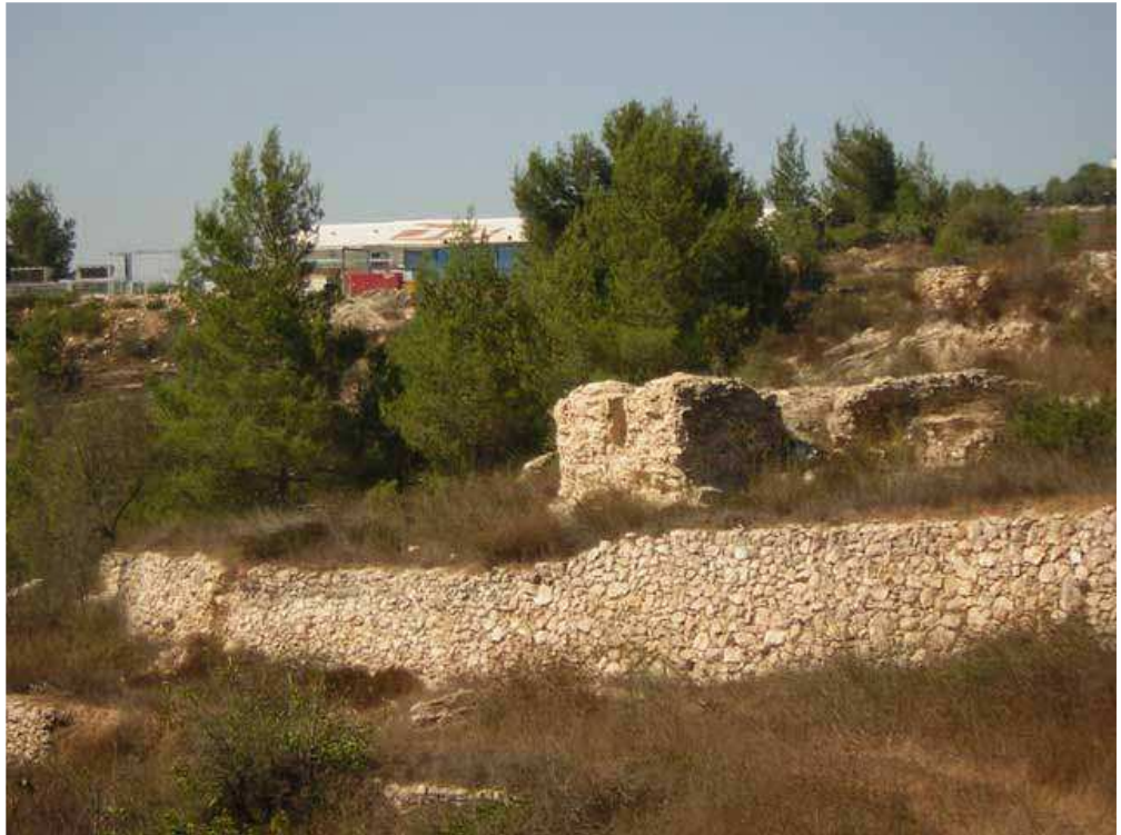
2. Site 14, rectangular building, looking north.
