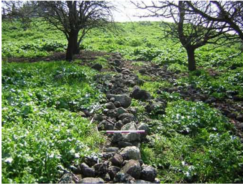
7. Terrace Wall 4, looking north.
