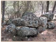
3. Built corner of field tower, looking west.
