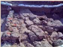
3. Foundation of Wall 6 and Walls 5 and 4, looking south.
