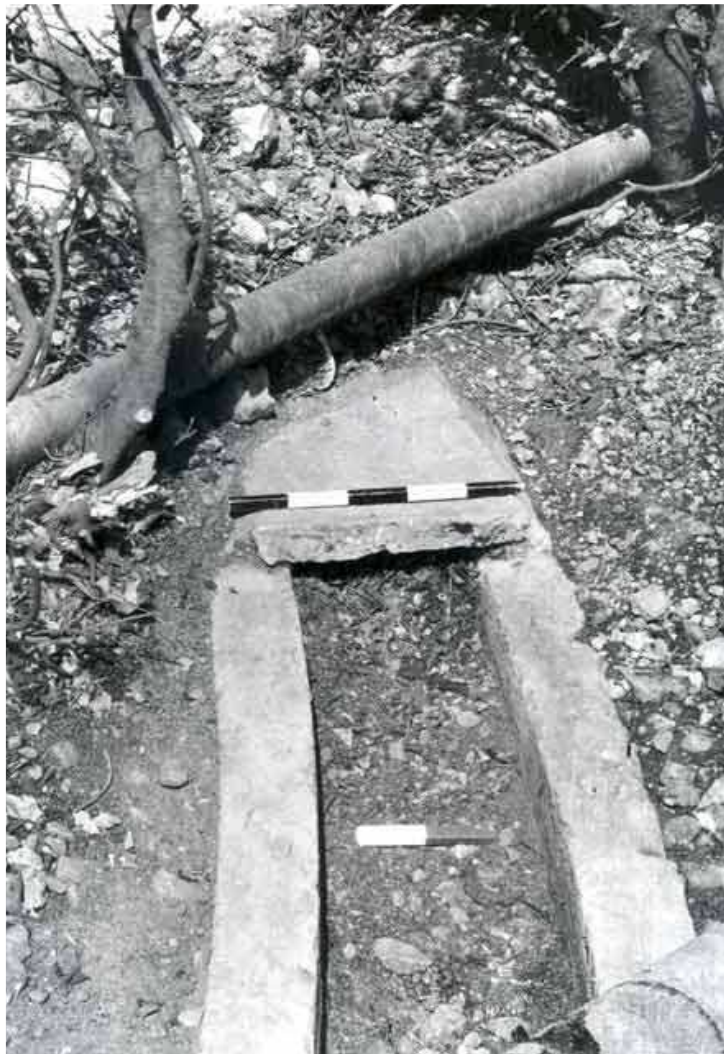
2. The concrete covering slabs atop the concrete Mandatory aqueduct, looking north.
