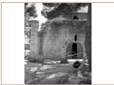
3. The structure, at the end of current excavation.
