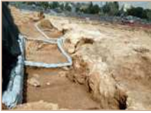
1. General view of excavation, looking northeast.
