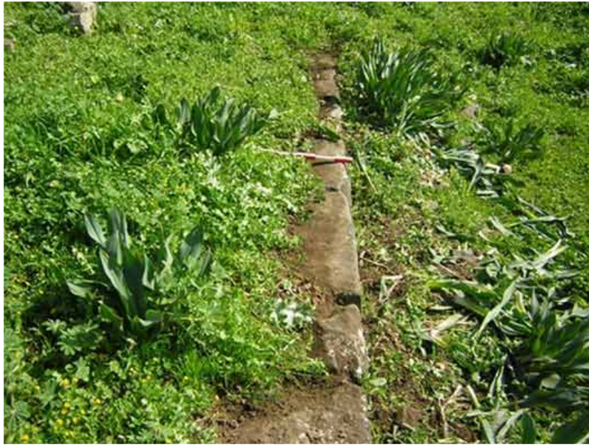
5. Wall 8, looking south.
