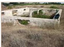
3. Modern building, looking north.
