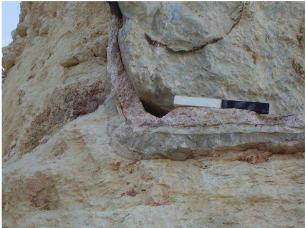
5. Western cistern, southwestern corner, looking north.
