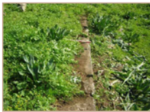
5. Wall 8, looking south.
