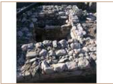
4. Phase II, the northern and southern wall casing, looking south.
