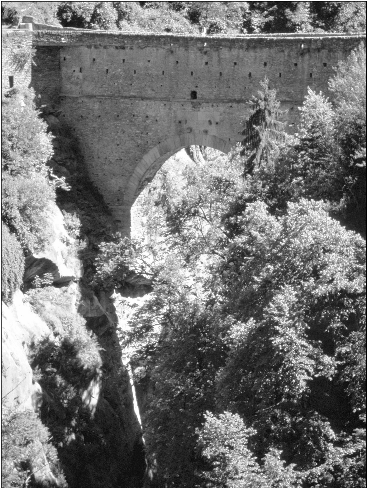
Fig. 5: The aqueduct bridge from north.
