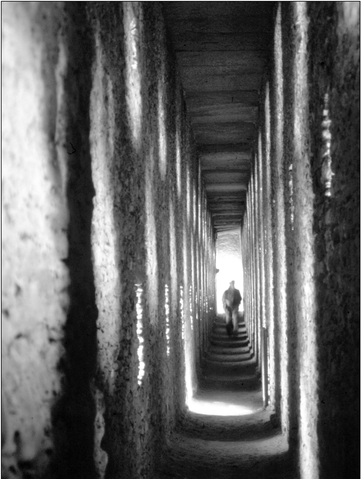
Fig. 7: Control-floor in the interior of the bridge-
