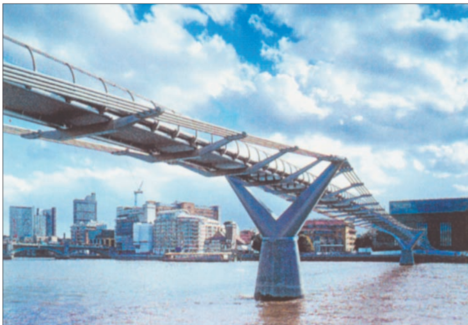
Millenium Bridge i London, Foster & Partners
