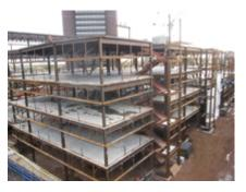
On the south site: Structural steel for the south building, at the end of October, was approximately 70 percent complete and the crane portion of the work should be completed by the end of November. Preparations for elevated concrete slabs from the second floor through to the roof levels began with half of the second floor concrete slab being placed in October (photo). The concrete slab placements will continue on all levels through the building during the months of November and December.
