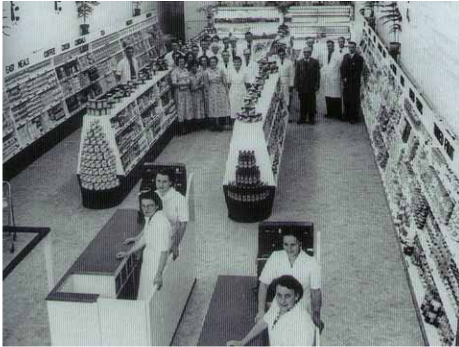
Figure 69 Supermarket in Cashel Street. One of Christchurch's earliest self-service stores. Canterbury Museum 12005 (P.F. Ford)
