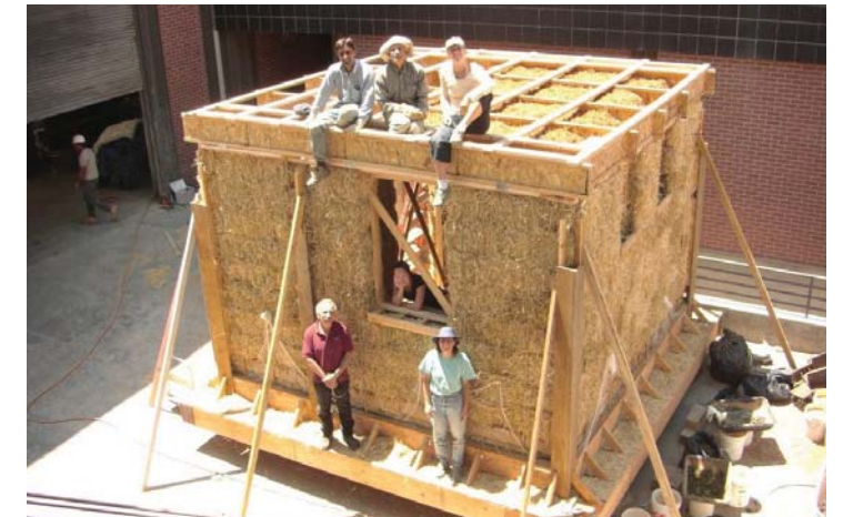
Fig. 17: Construction of a Full-Scale Straw Bale House
