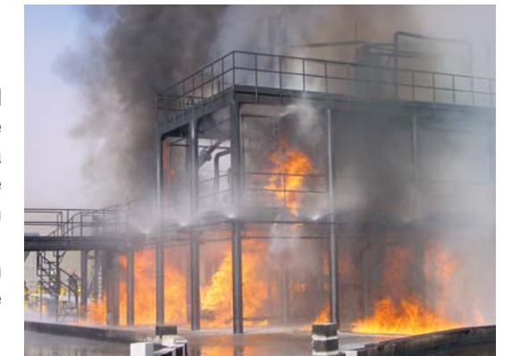
Fig. 27: Unprotected Steel Structure during Firefighter Training
