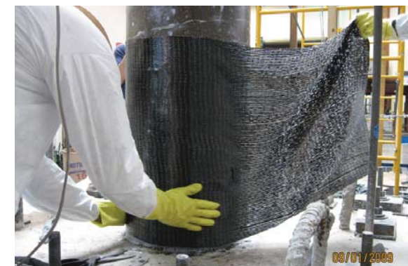
Fig. 11: Wrapping a Damaged Column with CFRP
