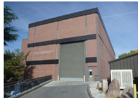
Fig. 33: The James E. Rogers and Louis Wiener Jr. Large-Scale Structures Lab
