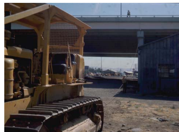
Fig. 1: Setting Up A Pull Test Using a D-8 Tractor, 1974
