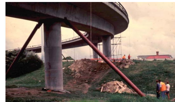
Fig. 2: Quick-Release Testing the Dominion Road Bridge in Auckland, New Zealand, 1985
