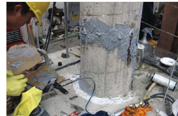
Fig. 10: Applying Mortar to a Damaged Column
