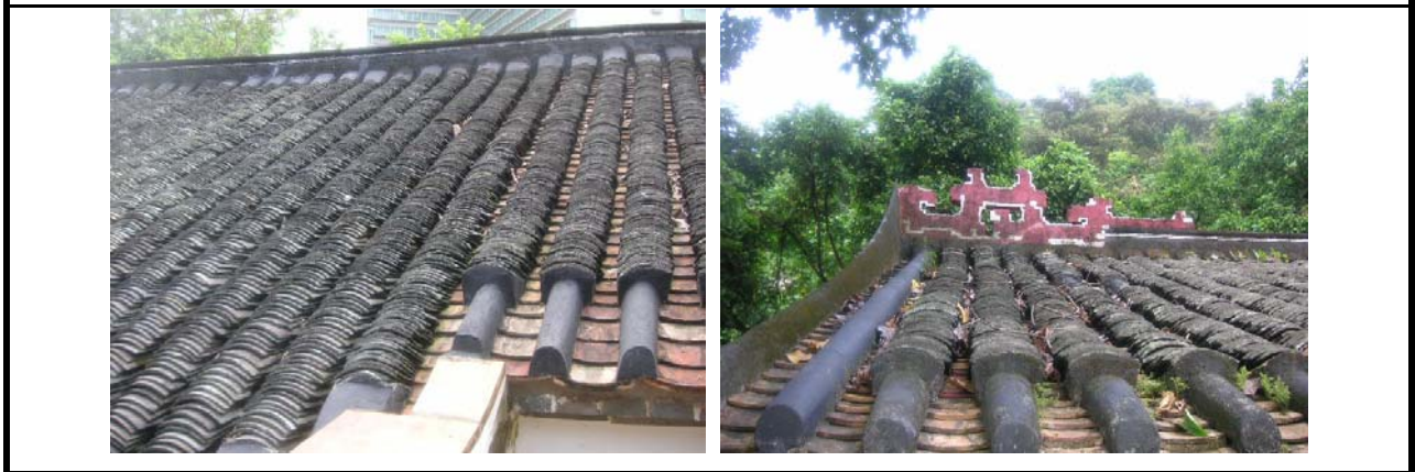
1.6) Chinese style tiled roofs and the geometric motifs at the front and rear ridge-ends at the roof
