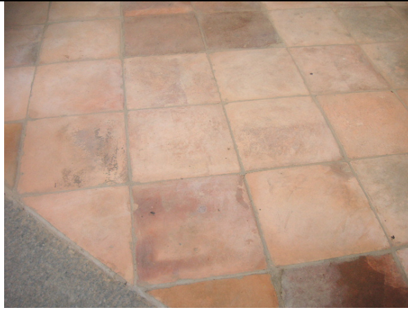
2.1) Canton floor tiles, including their laying pattern
