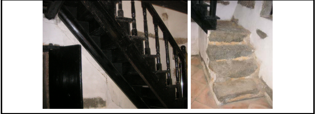
2.10) Timber staircase, granite landings and ornamental balustrades in the four side rooms
