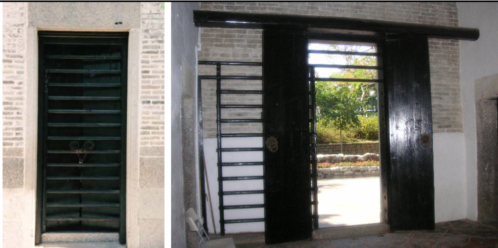
1.8) Sliding timber grille door and ironmongery
