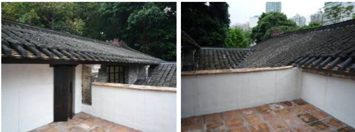
Flat roof of the Old House
