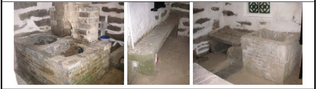
2.12) The brick stove with chimney, stone bench, water tank, and the associated facilities in the kitchen
