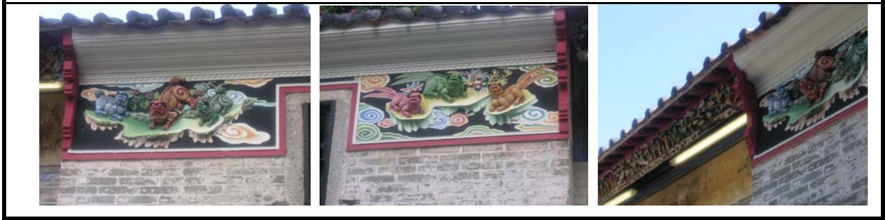
1.4) Decorative mouldings and timber brackets on the all façades
