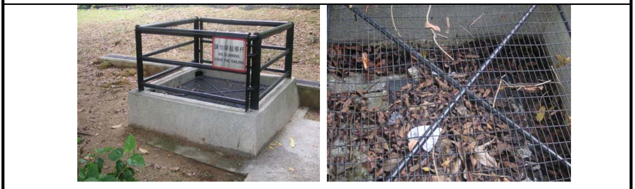
3.3) The water well located next to the House
