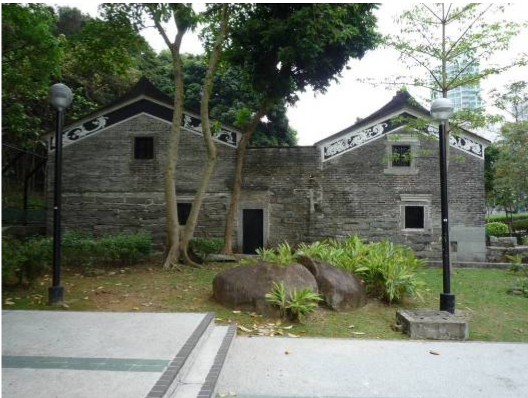
Side facade (facing north) of the Old House
