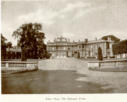
Esher Place—The Entrance Front.
