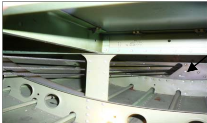
Bulkhead at STA 376.0 (Looking Aft)
