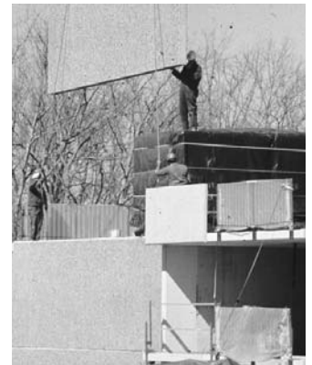
Construction View: placing the bearing wall, note the wrapped module.
