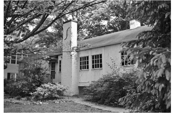
This three bedroom Gunnison Size 6-G constructed in 1949 includes optional architectural detailing and working fireplace. This example is located in Knoxville, Tennessee. (photo: Randy Shipp)
