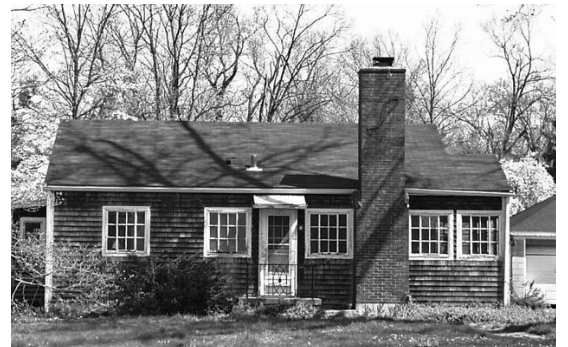
This two bedroom Gunnison Size 2-F constructed c. 1947 includes an optional Wind-O-Wing extension (to right) and working fireplace. This example is located in Lexington, Kentucky. (photo: Randy Shipp)
