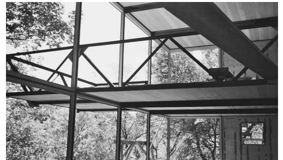
View of steel angle frame work. (photo: David W. George FAIA)
