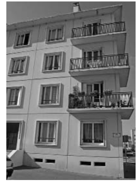
View of corner of balconies.
