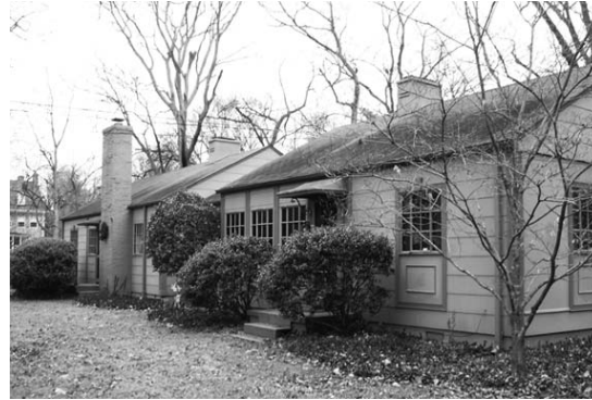
This Gunnison duplex consisting of a Size 3 (left) and a Size 2 (right) joined by an open arcade was constructed c. 1939. These examples are located in Nashville, Tennessee. (photo: Randy Shipp)
