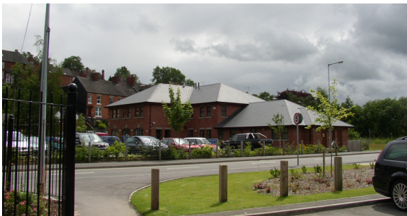
Doctors Surgery, Clifton Road – its form respects the gentle slope down to the brook.
