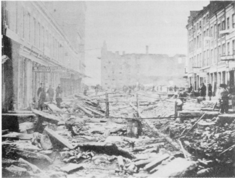
Rochester tried unsuccessfully to suspend the draft to focus on repairs following the flood of 1865. Looking south on Front Street after the swift waters receded, the damage is visible. Rochester Public Library.
