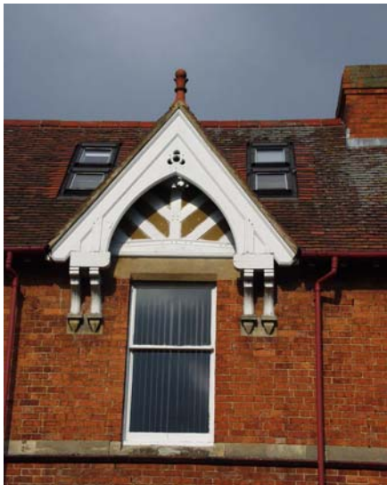
Dormer window Hightown Road – inopportune positioning of the roof lights detracts from the quality of the roof and detailing.
