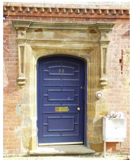
Doorway detail, Hightown Road
