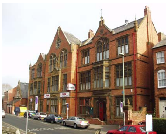
The Mechanics Institute, Marlborough Road
