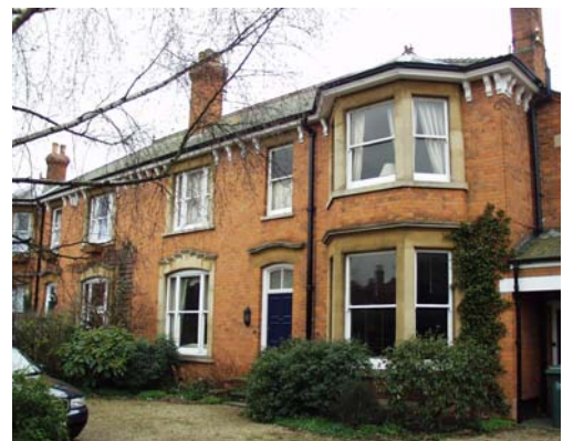
Broughton Road (south)
