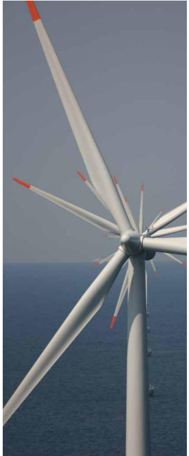
PHOTO: NYSTED OFFSHORE WIND FARM
