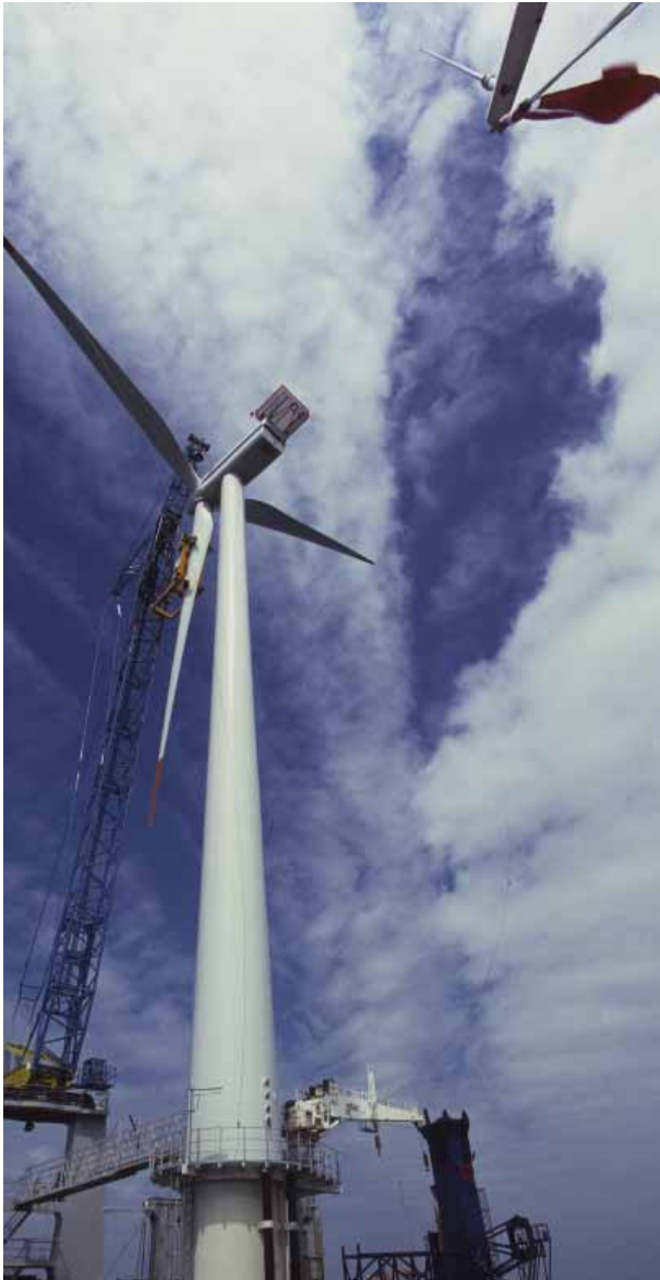
FIGURE 1.4 Construction of wind turbine at Horns Rev.
