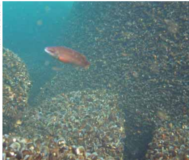
FIGURE 1.5 Scour protection with common mussels at Nysted.
