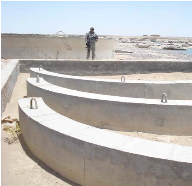
Photo 3: Concrete Arches in a Fabrication Pit
