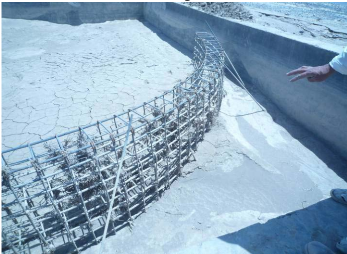
Photo 6: Reinforcement Bar Cage for a Concrete Arch in a Fabrication Pit
