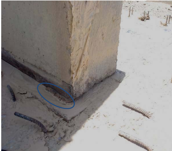
Photo 7: Connection of a Concrete Arch to its Pier
