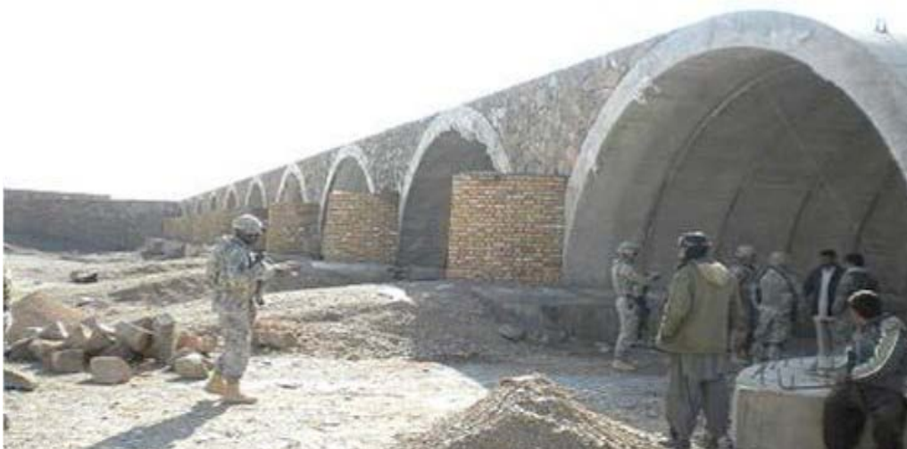
Photo 4: Tojg Bridge Construction, as of January 2010
