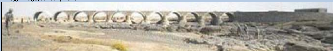
Tojg Bridge, January 2010
