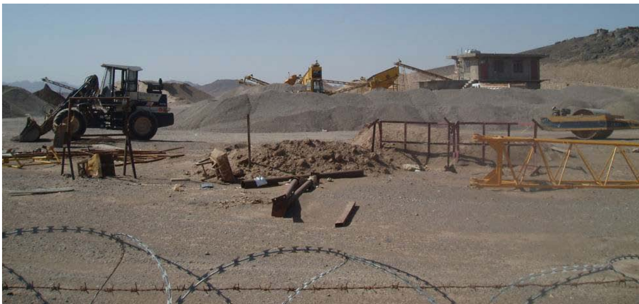
Photo 5: Gravel Plant Associated with the Tojg Bridge Contract
