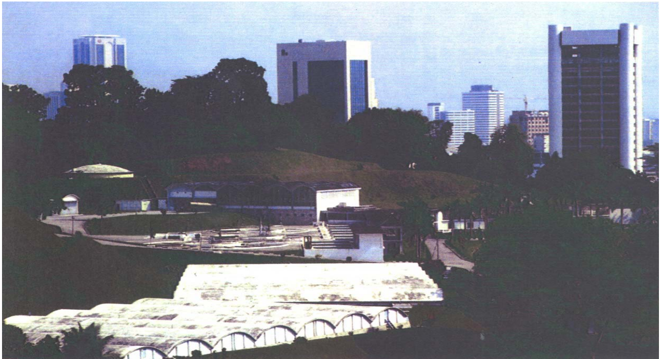
Bukit Nanas Treatment Plant high above Kuala Lumpur when commissioned in 1959, now in the shadow of tall buildings
