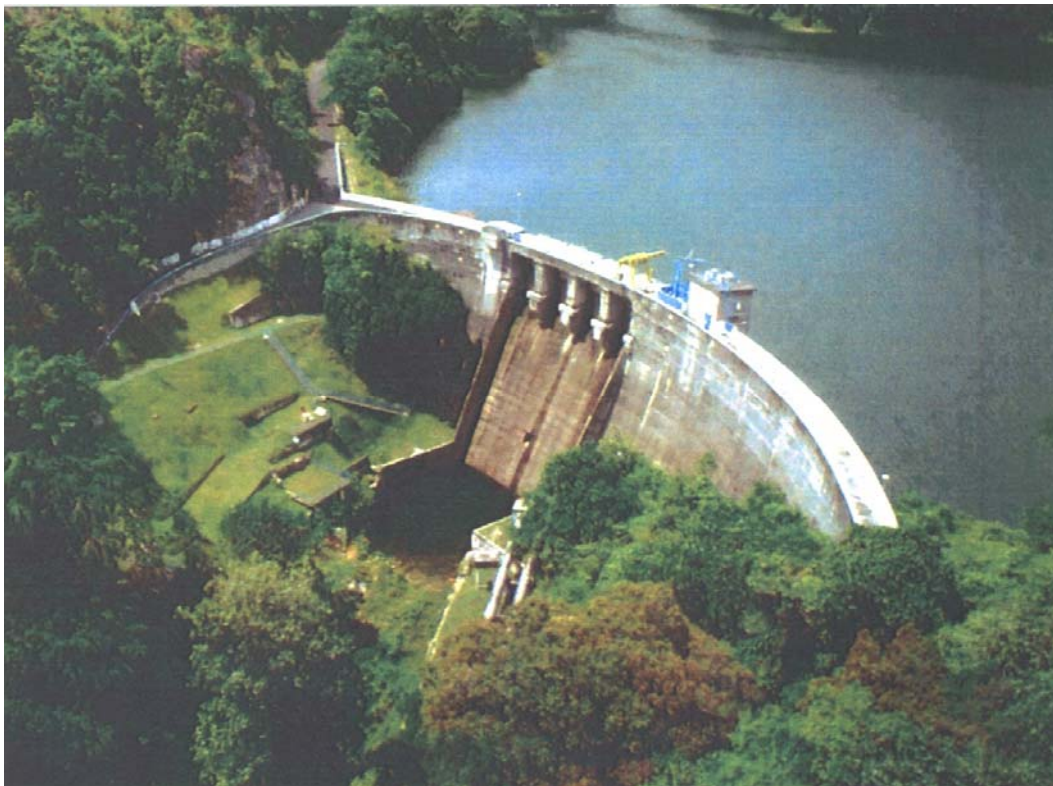
Klang Gates Dam, Kuala Lumpur : completed in 1959 for water supply and raised 3 metres (10 feet) in late 1979 for flood mitigation
