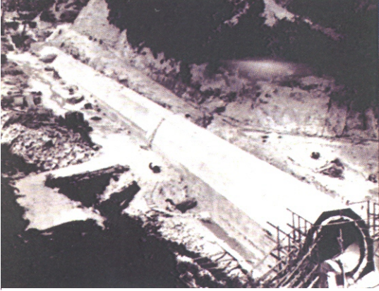
The overflow / scour tunnel of a dam under construction
