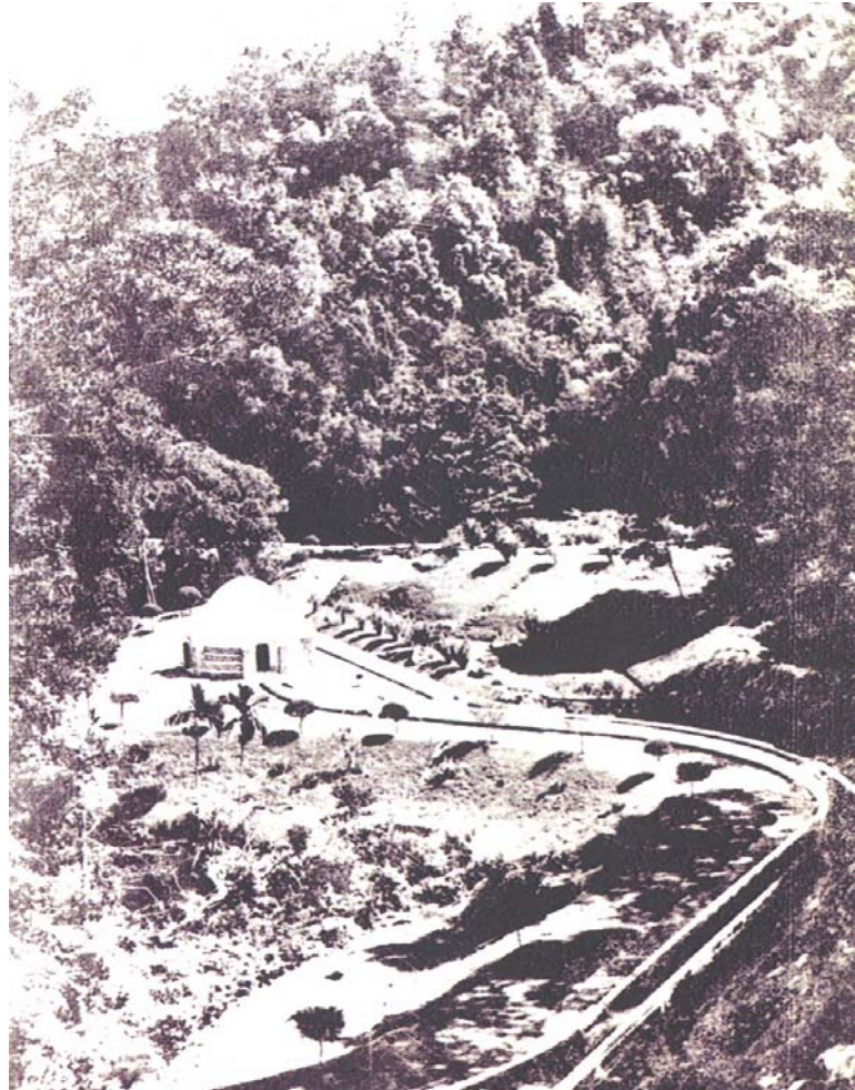
Batu Ferringhi Aqueduct : constructed between 1926-1929 – 6km long, of which 1.4km is in tunnel
