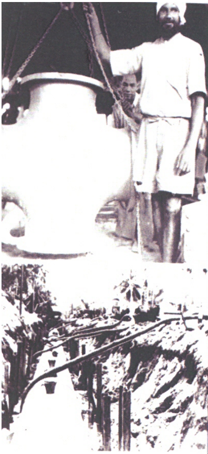
Handling and laying pipes in pre-War days
