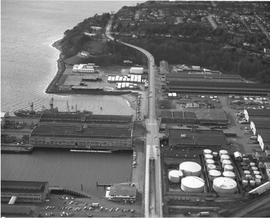
Figure 5. An aerial photo view from the east shows the tank farm site in Area 1 to the right foreground, with southern portions of Area 2 and the eastern edge of Magnolia Bluff in the background. This photo dates from February 13, 1975 (Port of Seattle).
