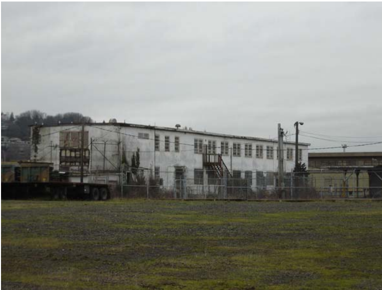
Current view of the southeast corner of Building #220 (West Stockade/Brig)
