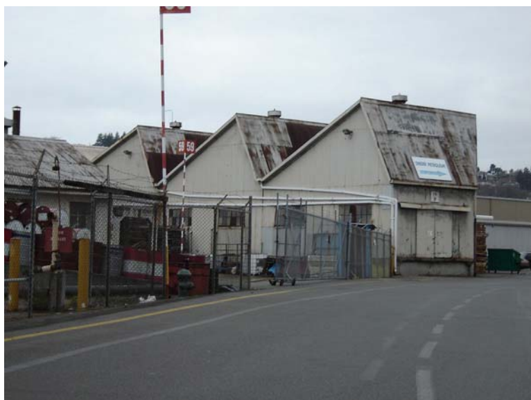
Oblique view of the south and east facades of Building #19.
