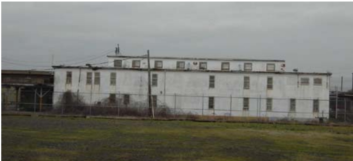
Current view of the south facade of Building #216
