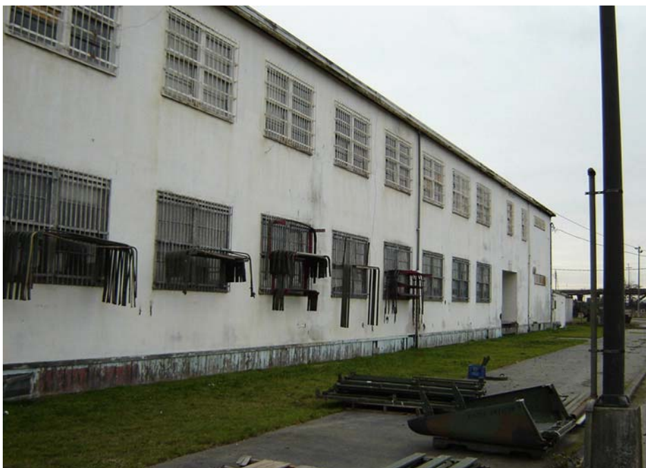
Detail view of Building #220, west facade. Conditions at Building #216 are similar.
