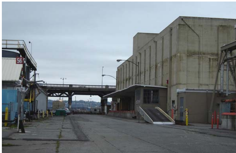
Current oblique view of the east side/northeast corner of Building #39.
