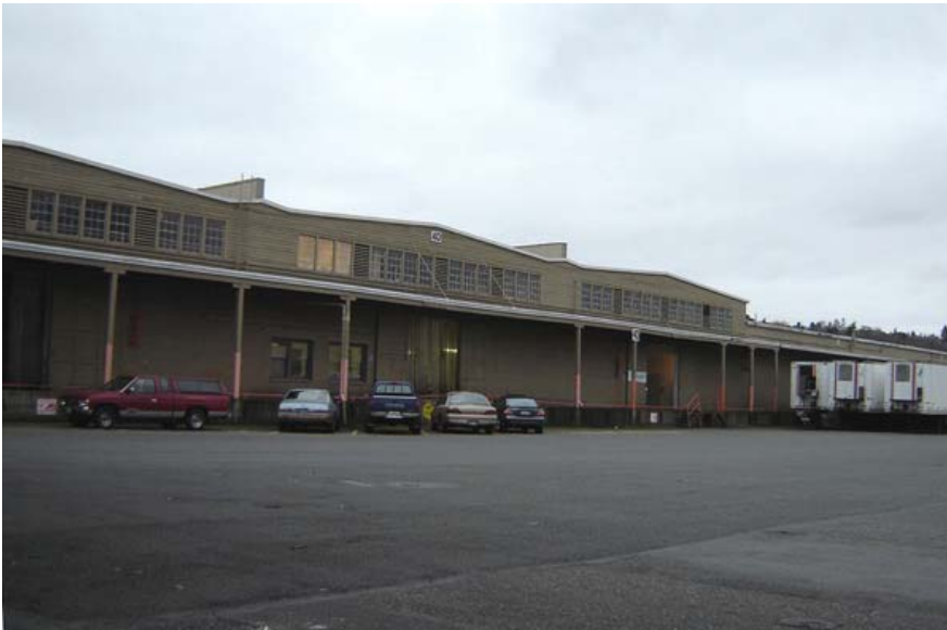
Current partial view, looking northwest, of the east facade of Warehouse #40.
