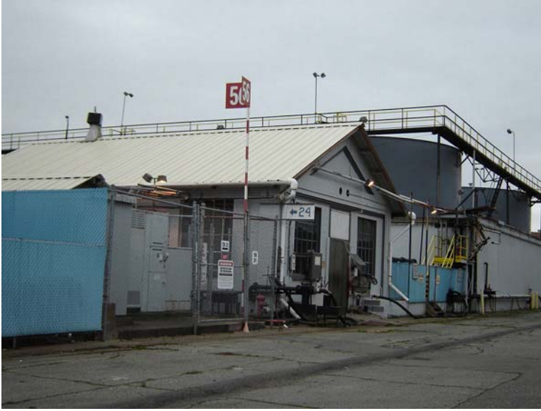
Oblique view of the northwest corner of Building #26 (Fuel Pump House)
