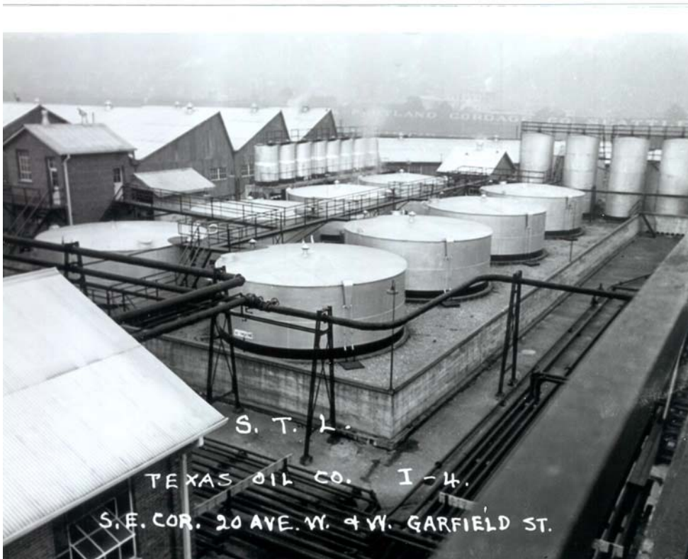
These two photos of the Texas Oil Company Tank Farm site, are from the King County Tax Assessment form, and date from 1937. Portions of Building #19 are visible in the background.
